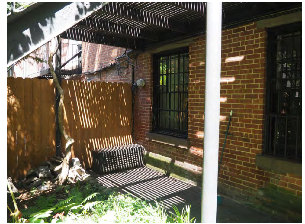
Existing basement windows facing rear yard
