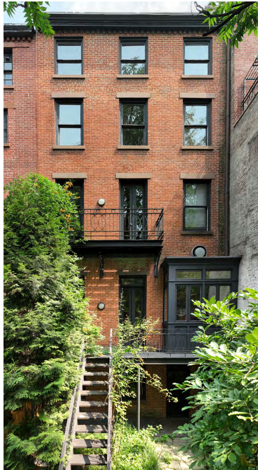
Existing rear facade from yard
