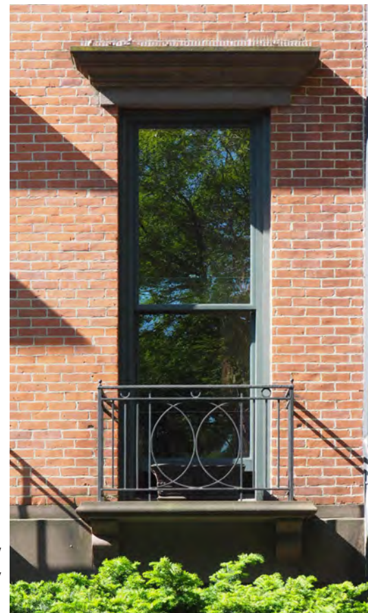
Existing parlor window and balcony
