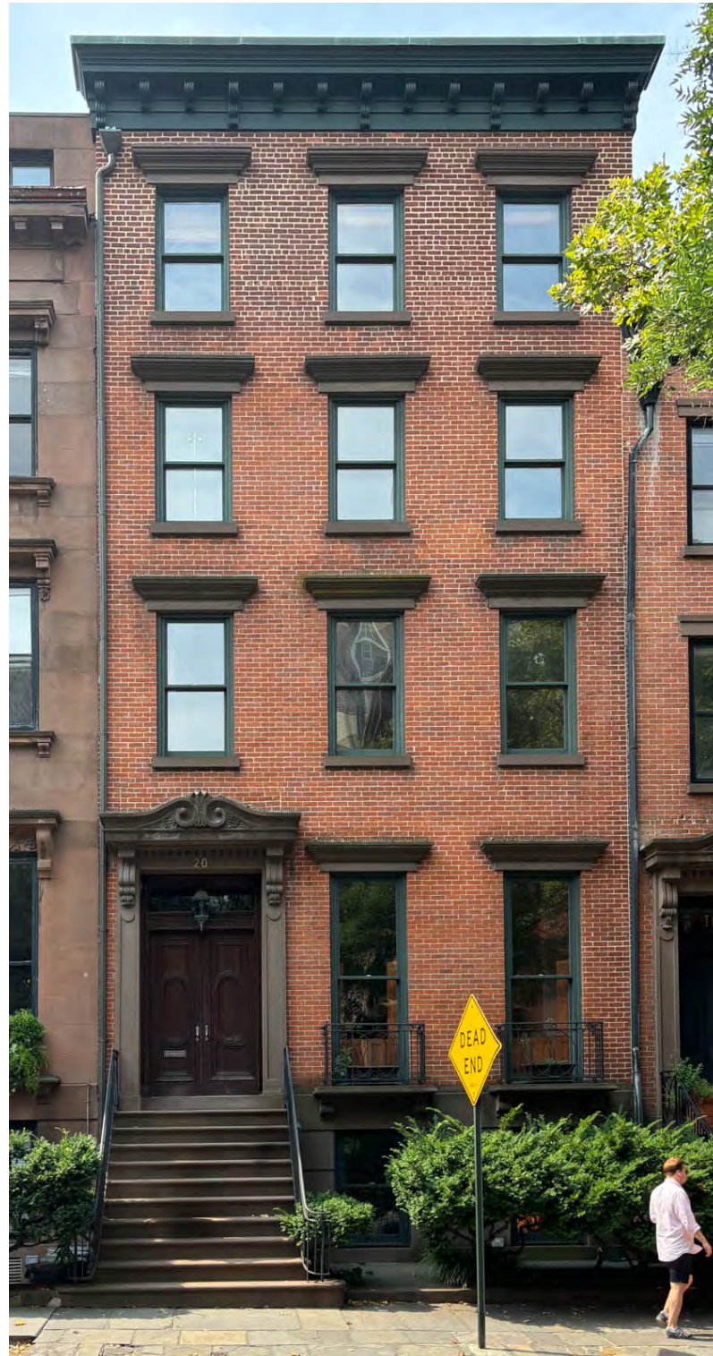
Existing front facade
