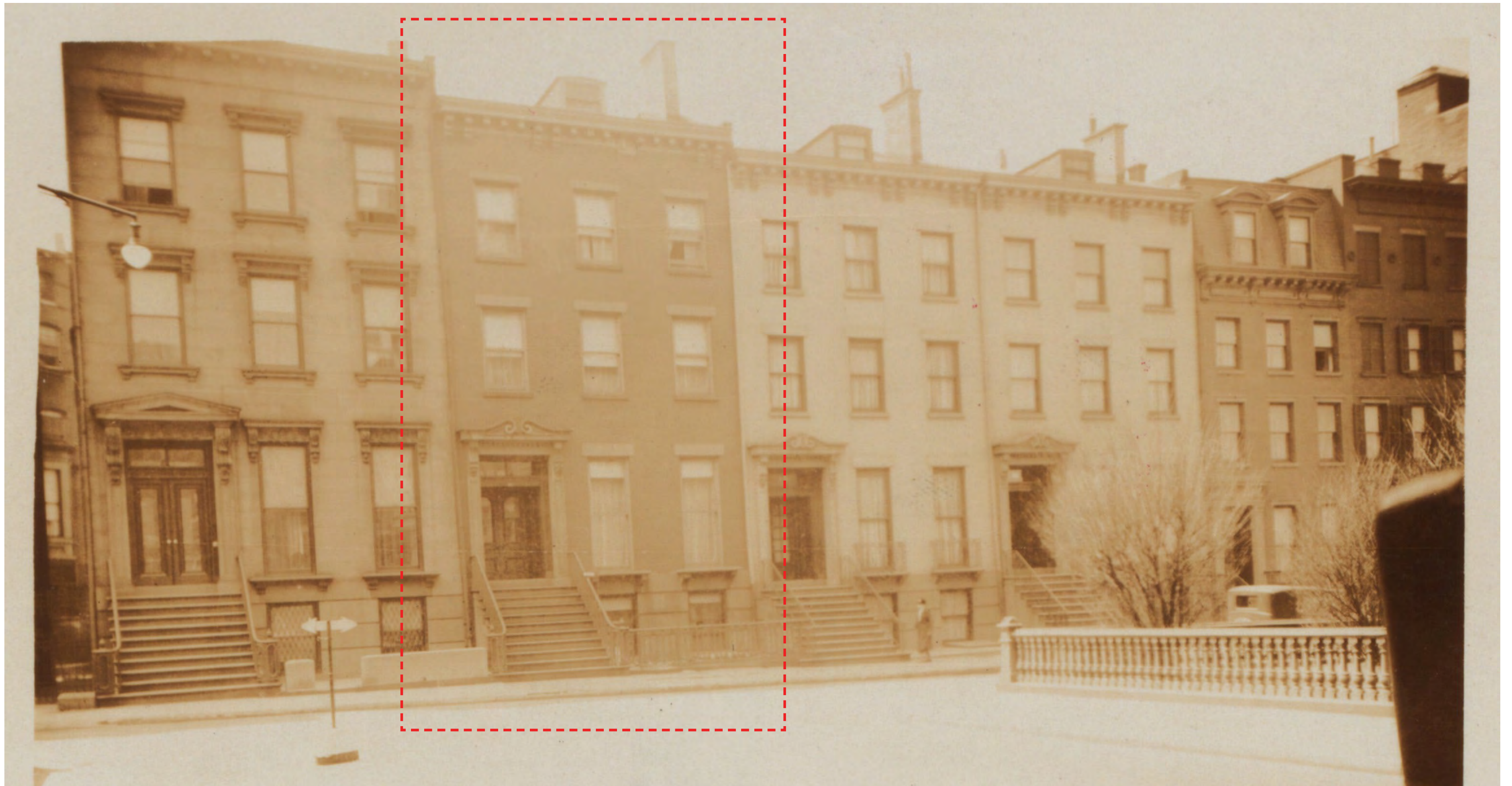
20 Remsen Street front facade and adjacent context NYPL, 1932
