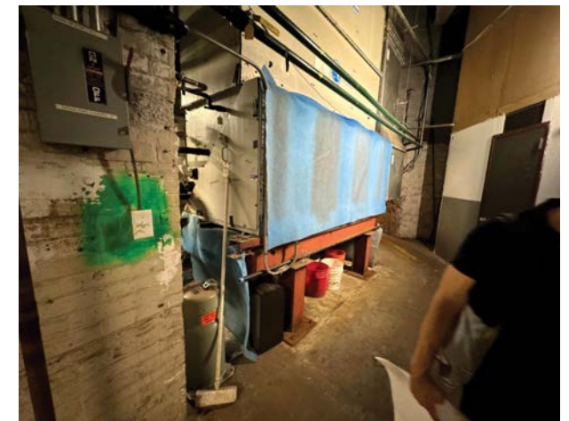
EXISTING NORTH COOLING TOWER TO BE REMOVED
