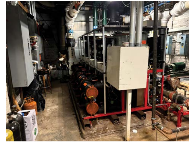
EXISTING MULTI-STACK CHILLER
