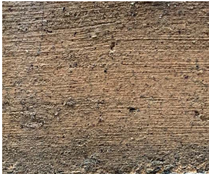
Photo of Existing Church Brick
