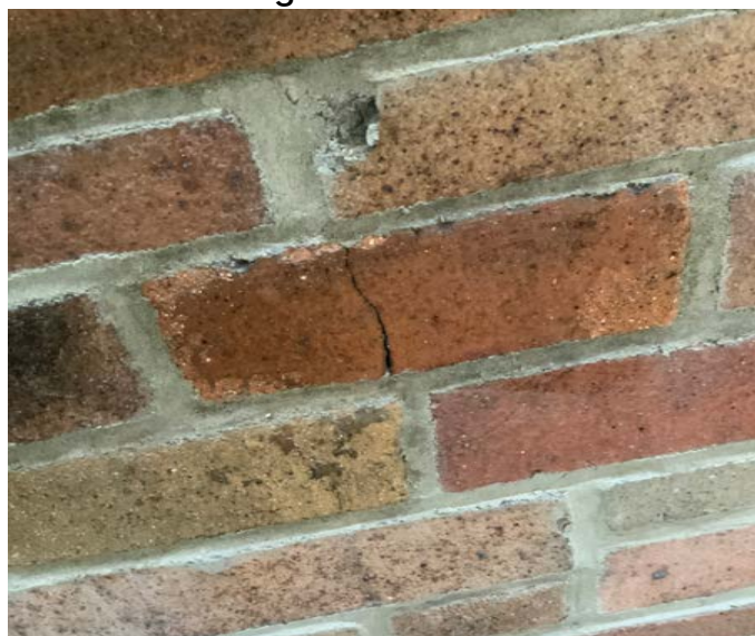
Photo of Existing Church Brick
