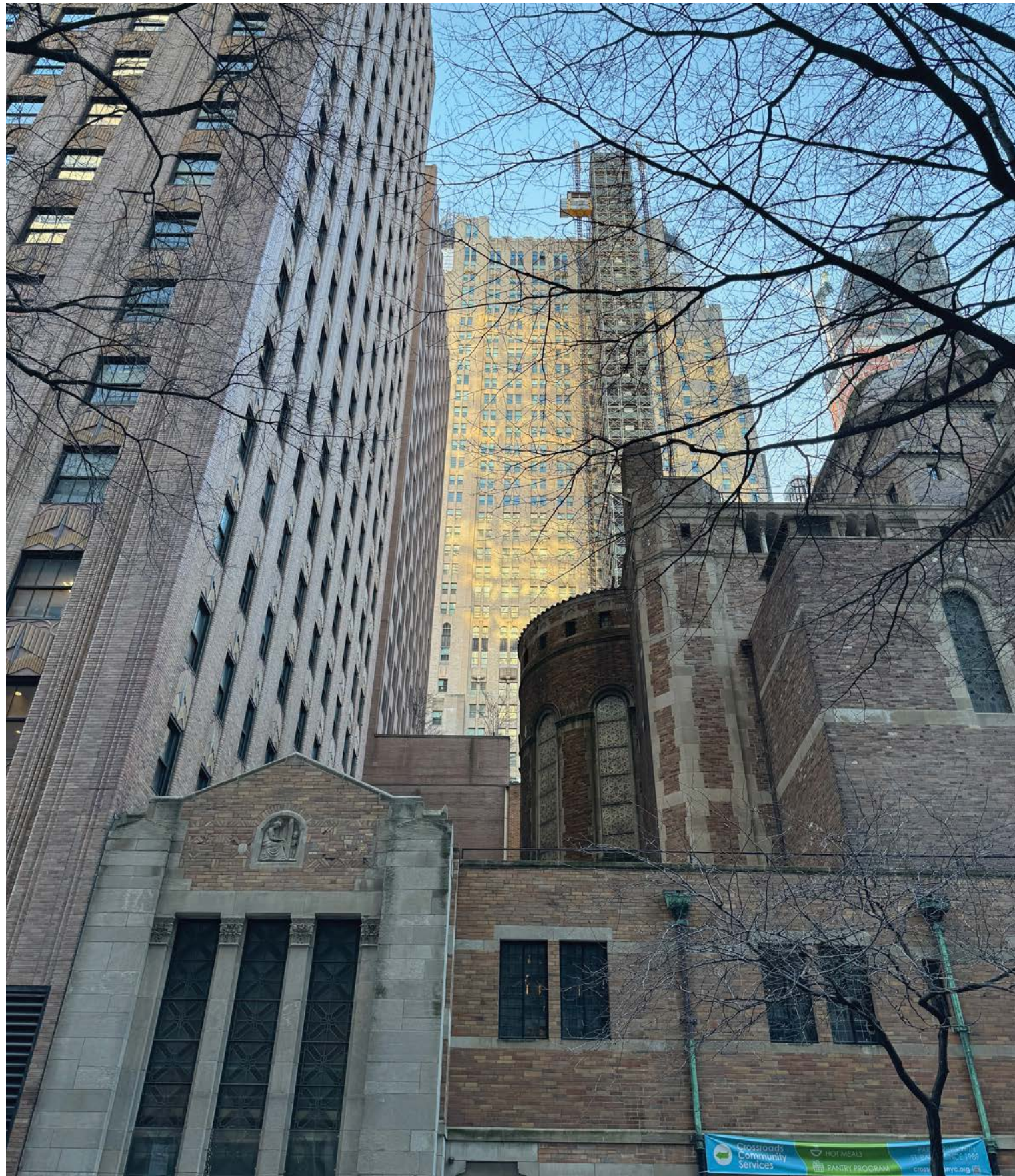
PHOTO VIEW A - FROM SIDEWALK
