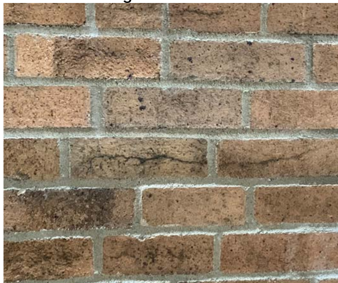
Photo of Existing Church Brick
