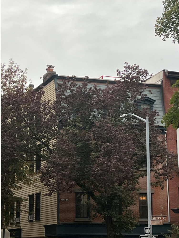
VIEW FROM CRANBERRY STREET WHERE THE PROPOSED BULKHEAD FIRST COMES INTO VIEW
