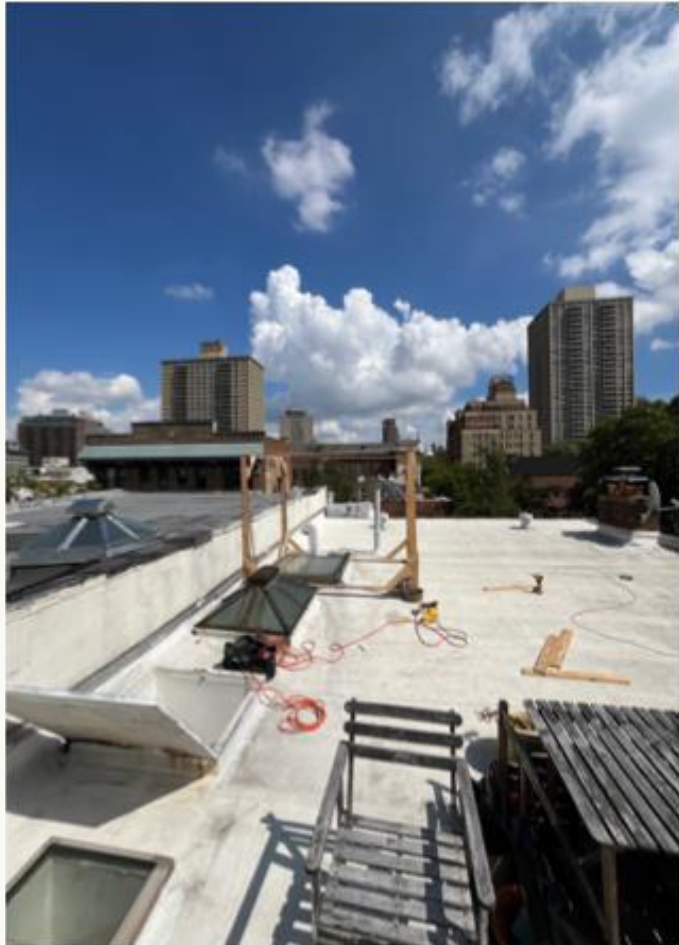
Bulkhead mock-up, view east
