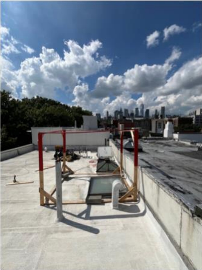
Bulkhead mock-up, view west
