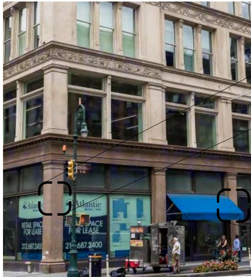
EXISTING CORNER CONDITION
