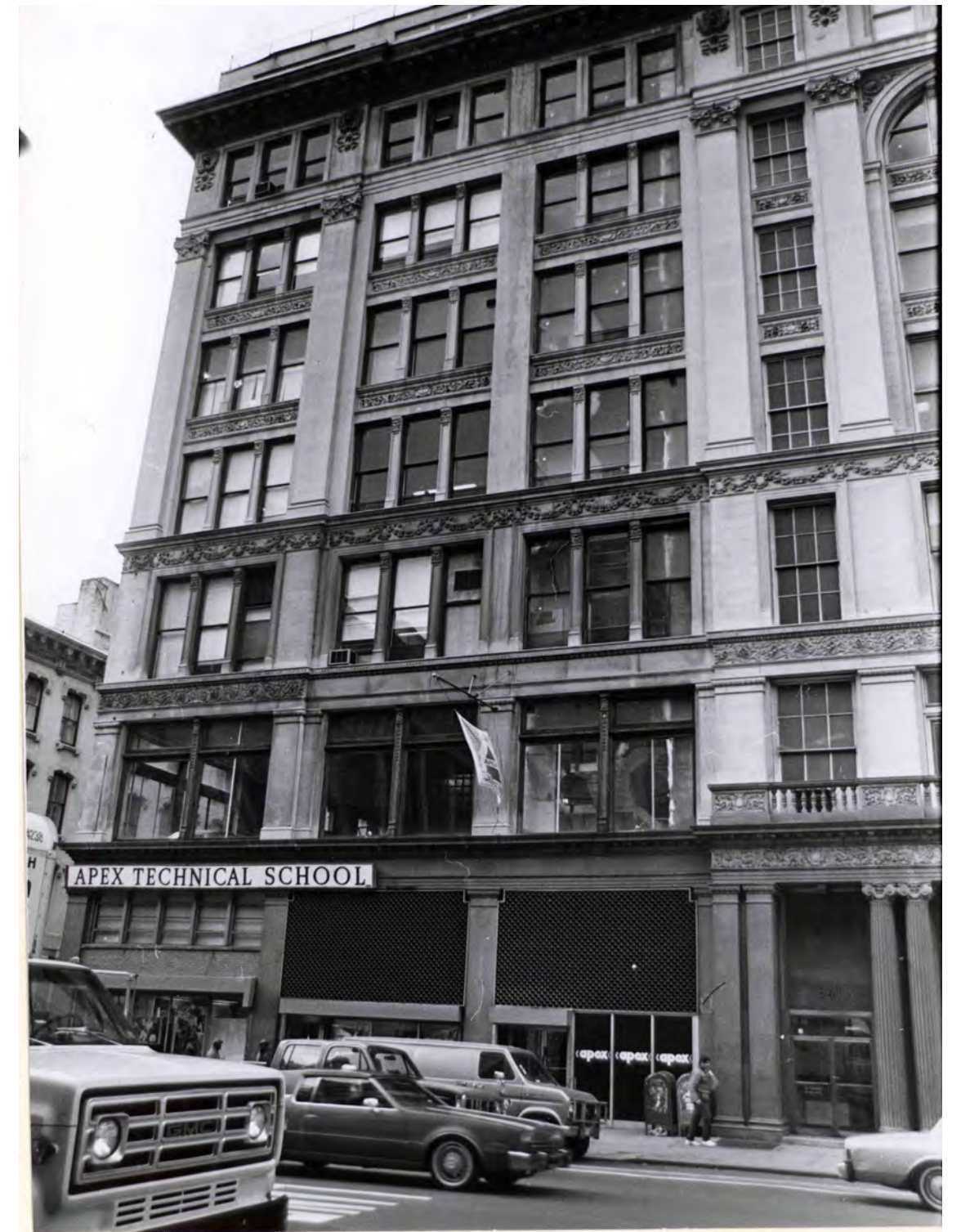
LPC Designation Photo, 1989
