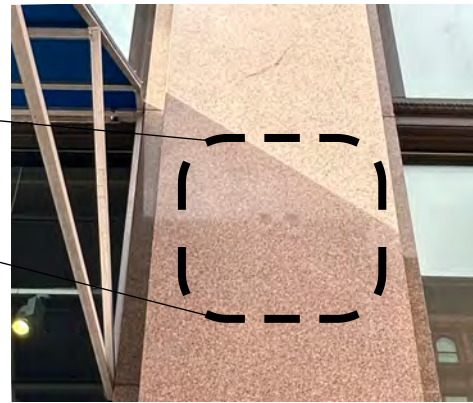
EXISTING ANCHOR PATCHING AT GRANITE
