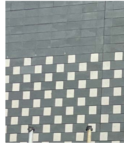
EXISTING NORTH WING BLOCK WALL
