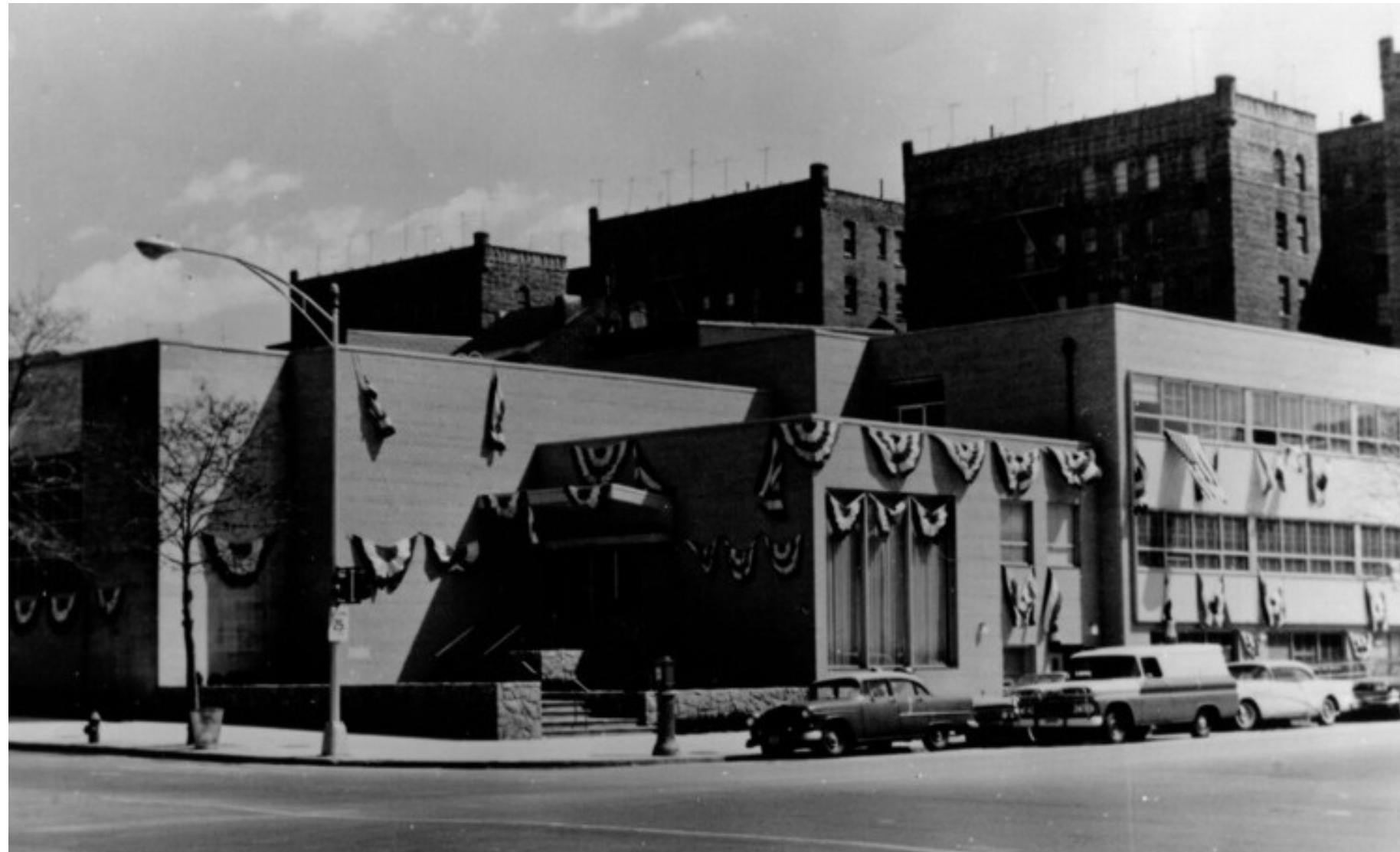
EXISTING 1961 SYNAGOGUE FACADE = BRICK
