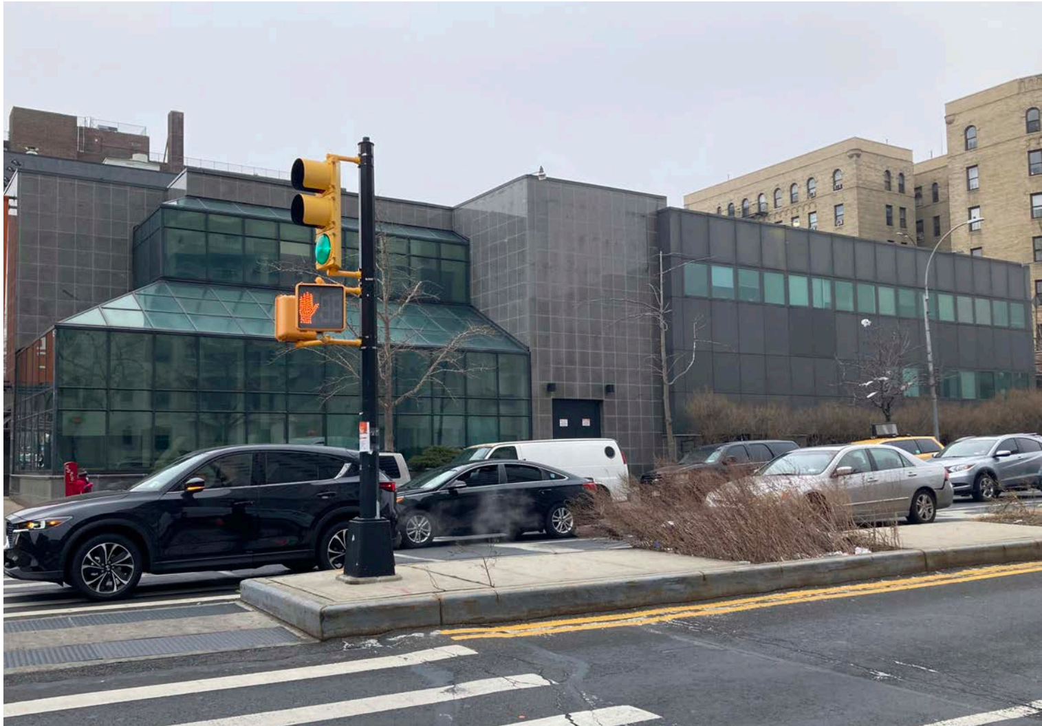
EXISTING FACADE WITH METAL PANEL
