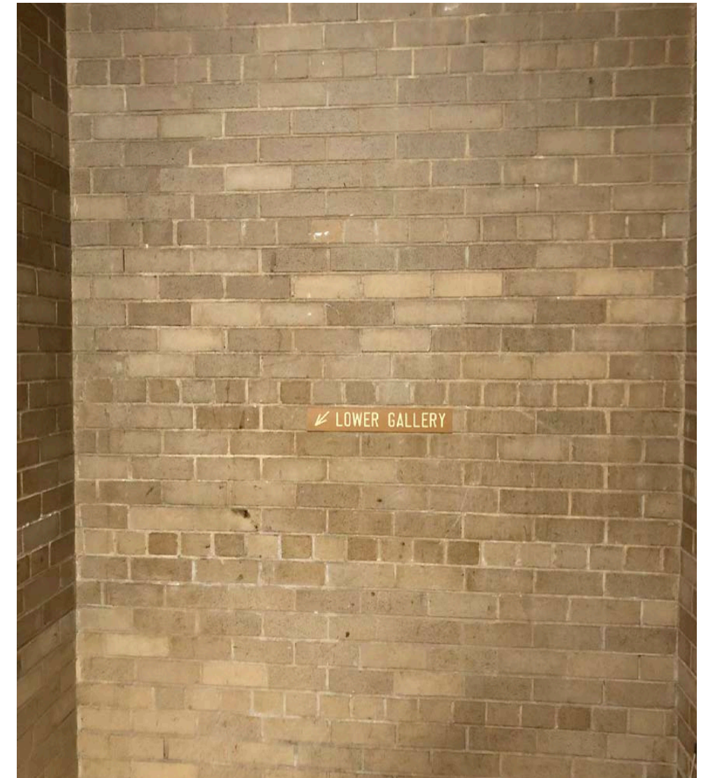
COLOR OF EXISTING FACE BRICK, SEEN FROM INSIDE BUILDING
