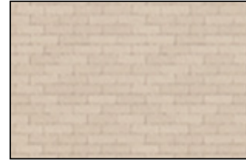
Stained Existing Brick
