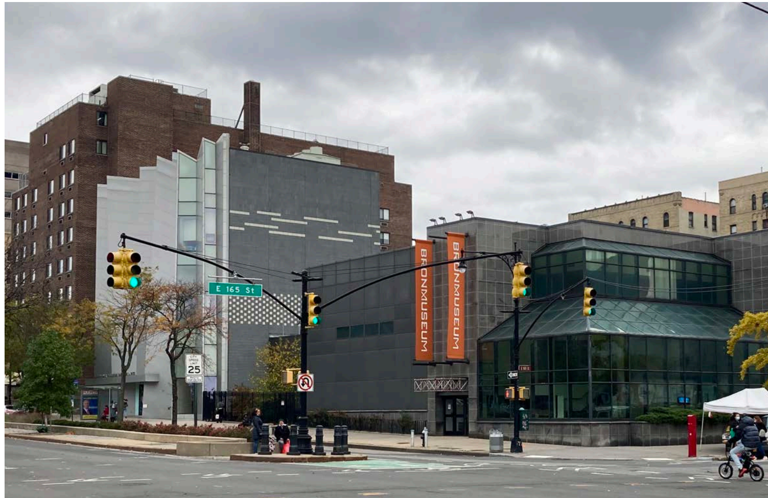
EXISTING FACADE WITH METAL PANEL
