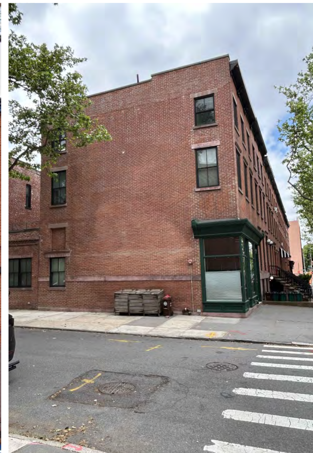
E 132 KANE STREET SIDEWALL WINDOWS LPC-009
