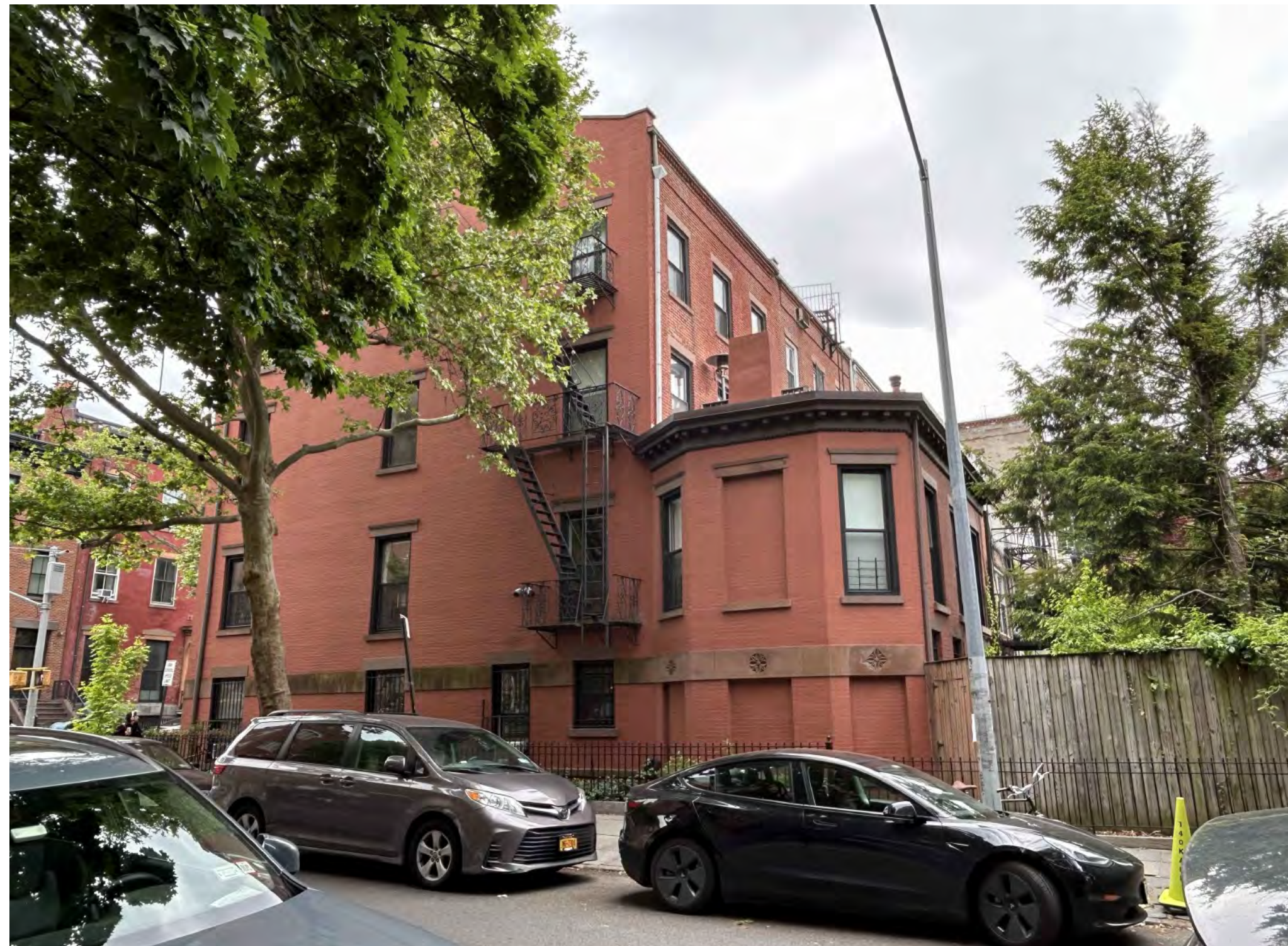
D 424 HENRY STREET SIDEWALL AND 2-STORY ADDITION LPC-009
