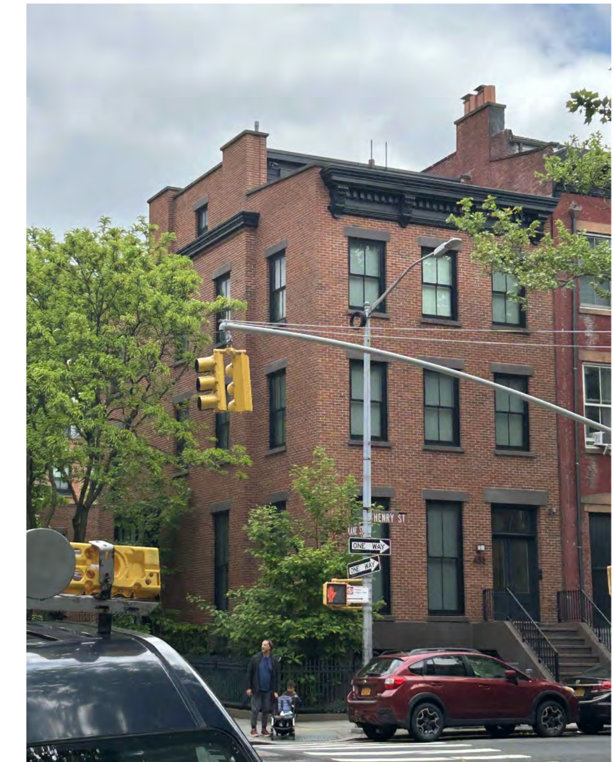
A 435 HENRY STREET ROOF AND DECK (NEW BUILD) LPC-009
