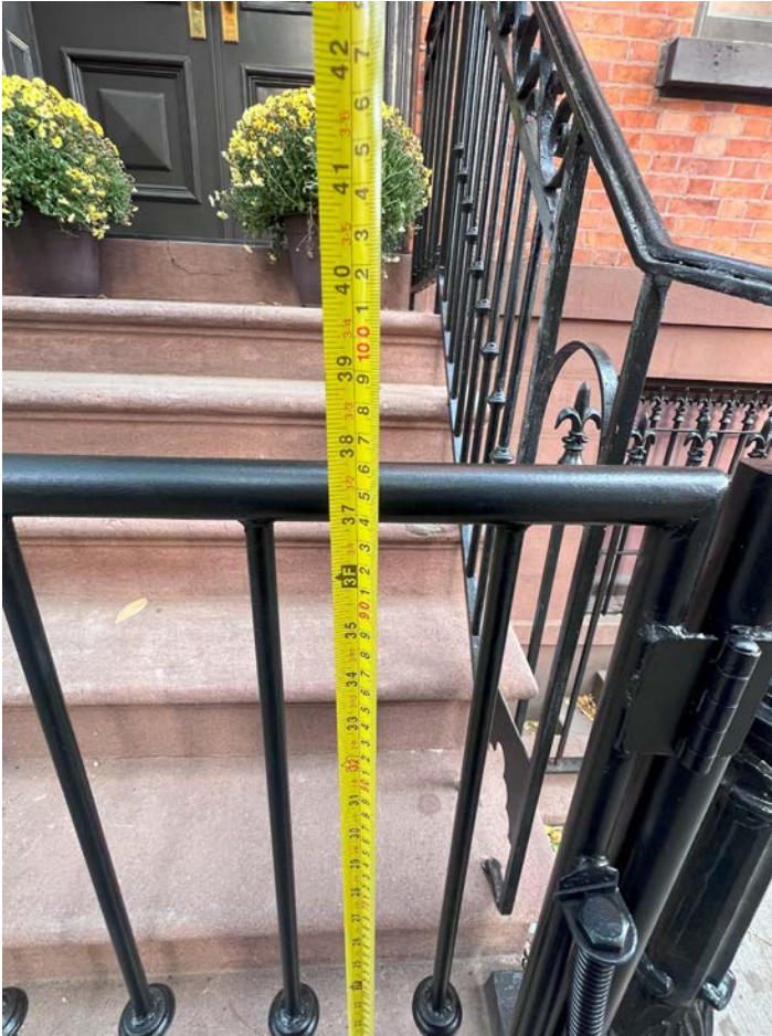
Measurement: First step to top of gate (37.5")
