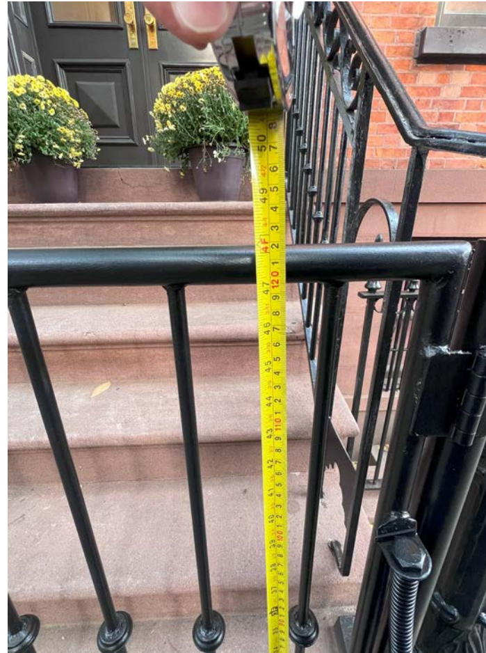
Measurement: sidewalk to top of gate (48")
