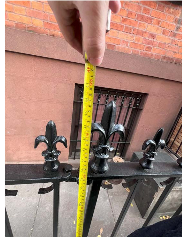
Measurement: sidewalk to top of areaway fence (46"; this is higher than first step to top of gate)
