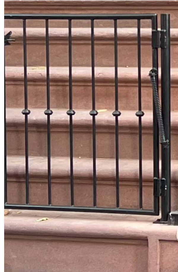
Design of proposed spindles for stoop gate
