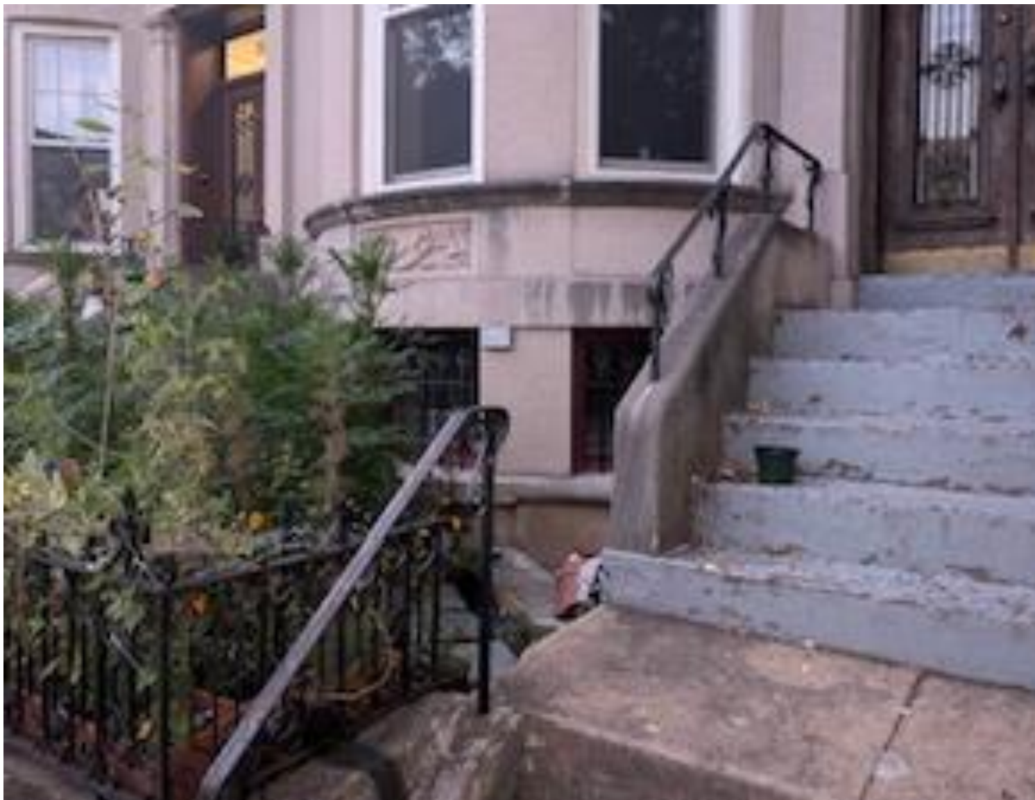
Basement Windows as Visible From Sidewalk Below Stoop
