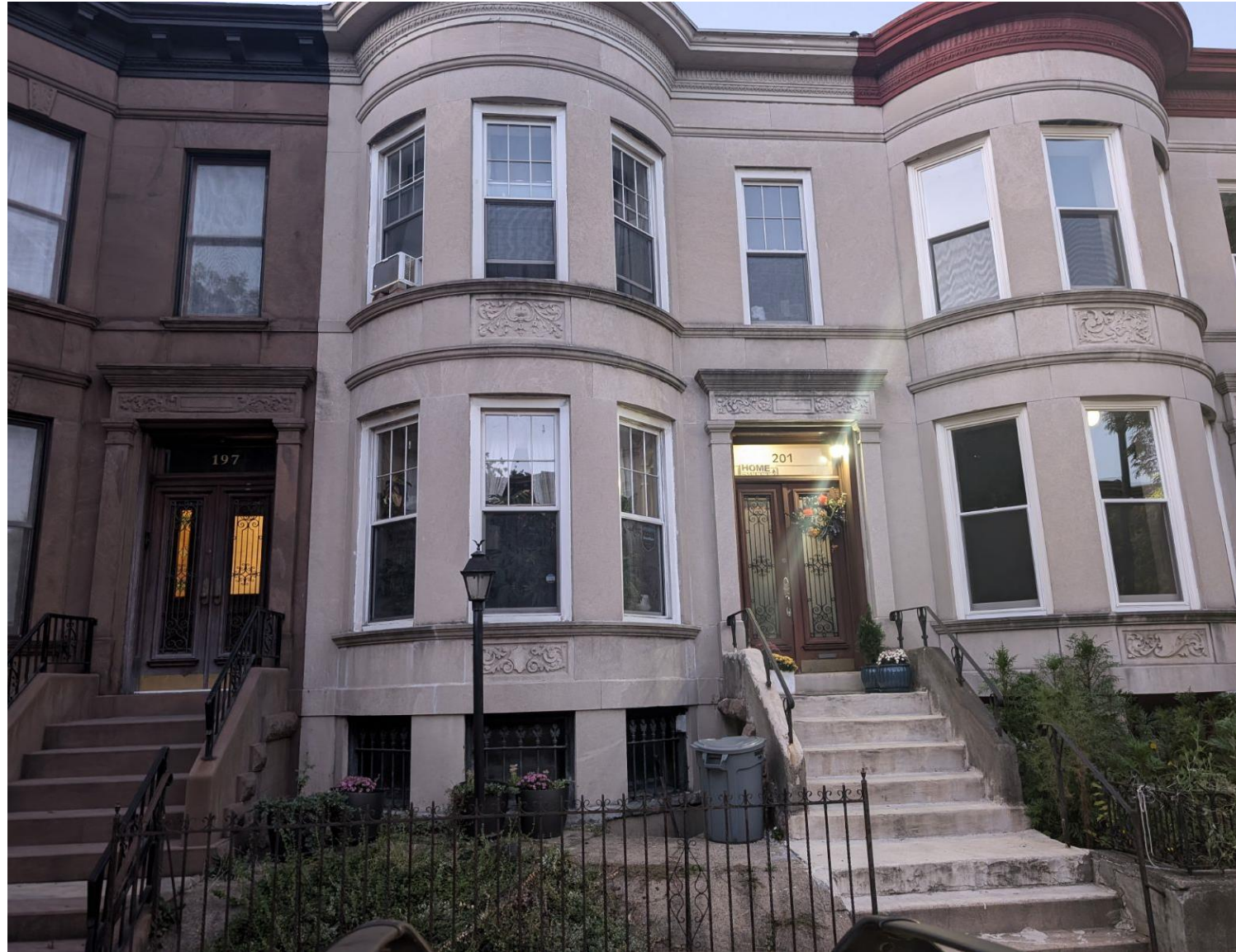
201 Maple – Adjacent Townhouse (203 is to its right)
