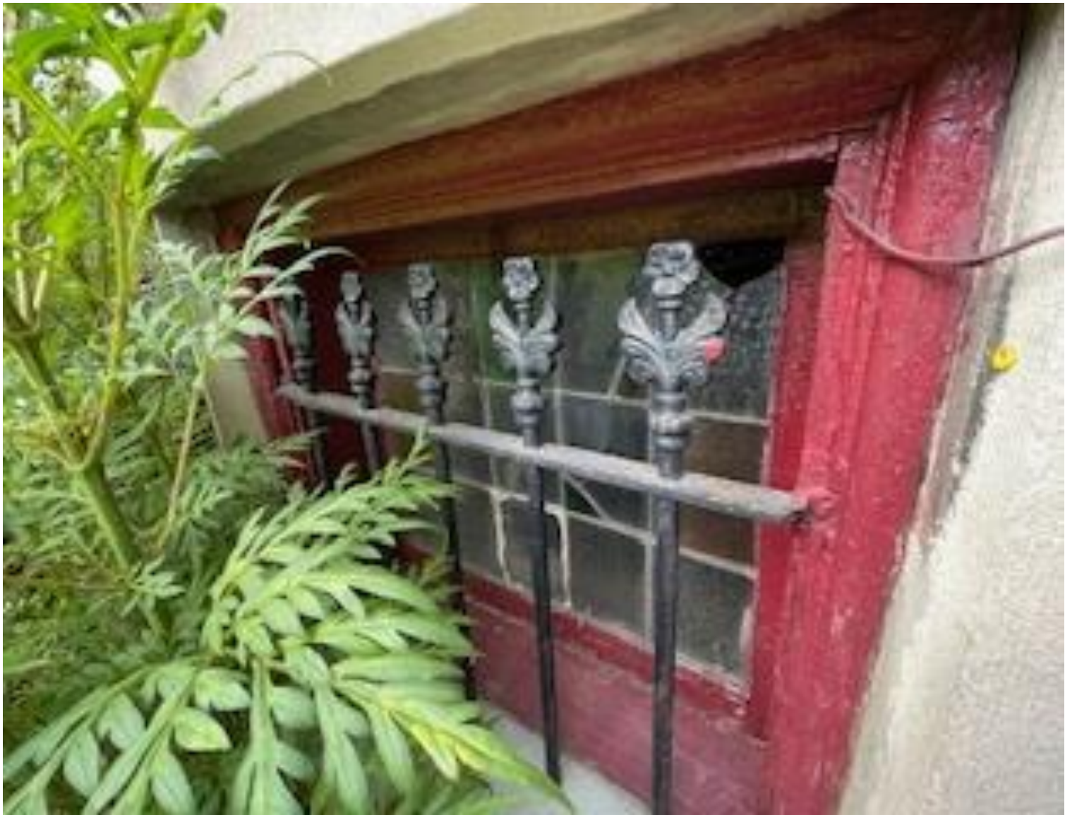
Middle Basement Window
