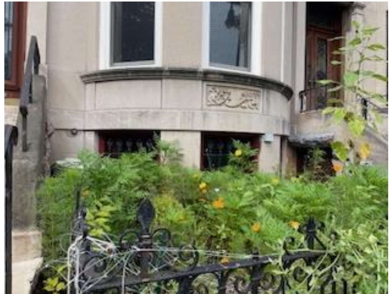
Basement Windows as Visible From Sidewalk
