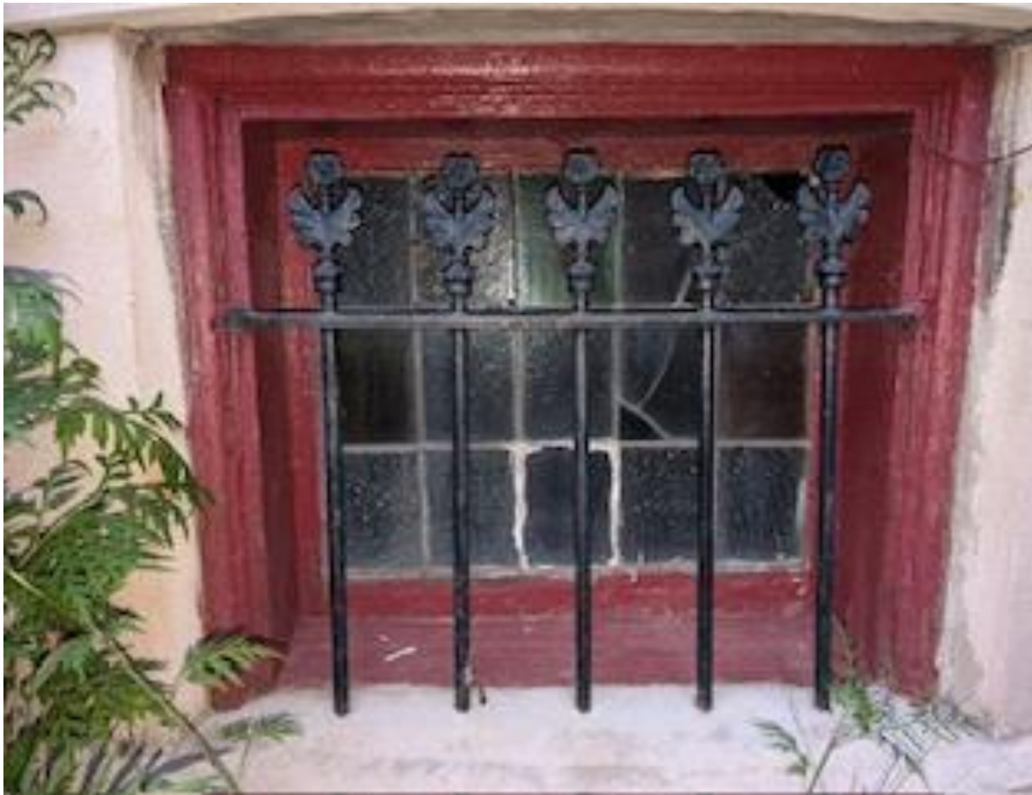
Middle Basement Window
