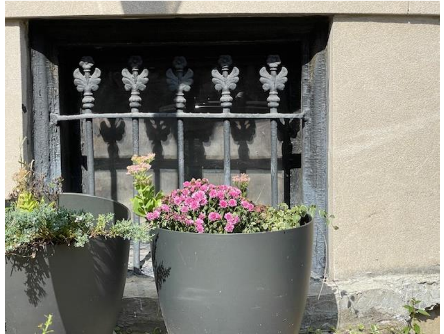
201 Maple Street – Basement Window
