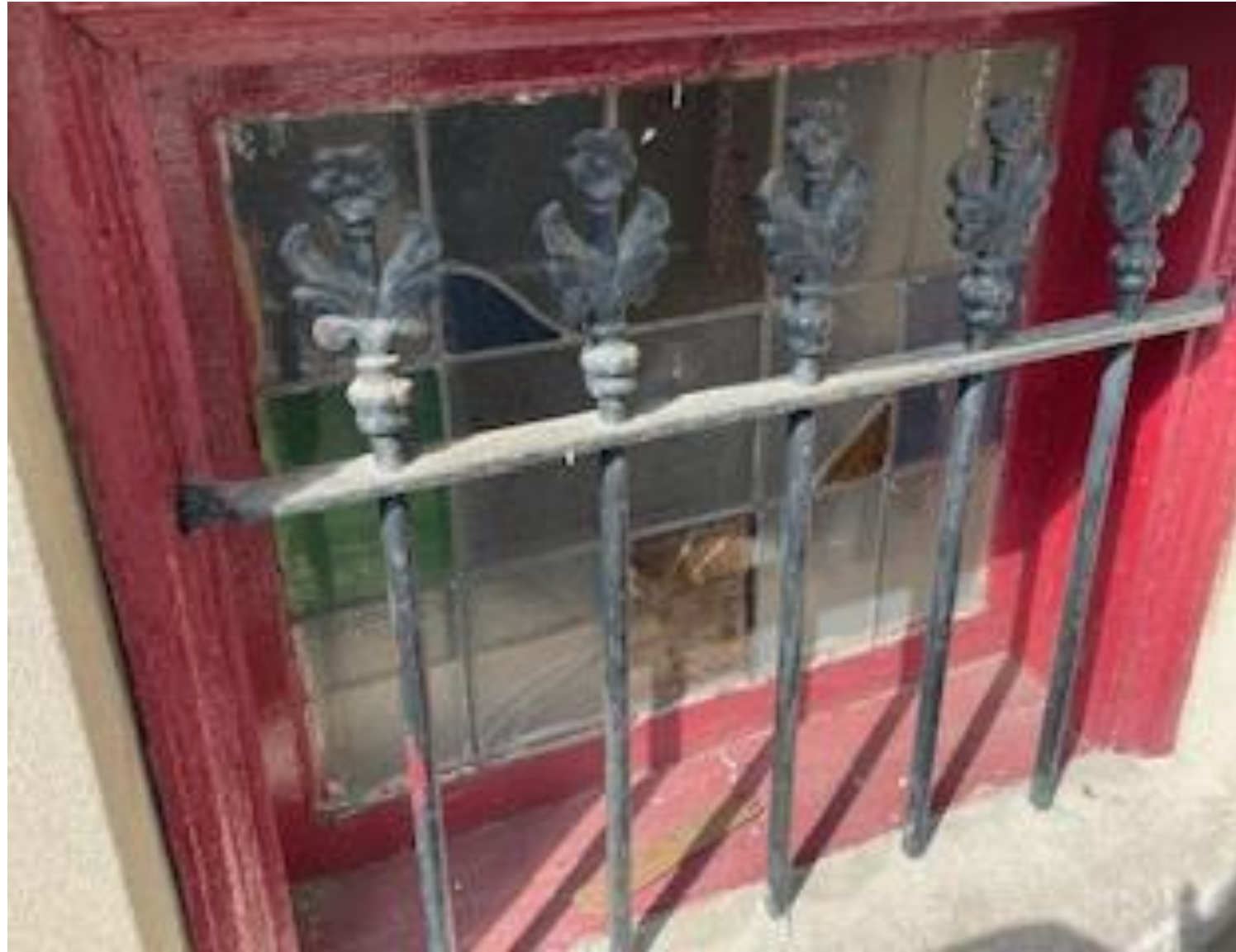
Right Basement Window
