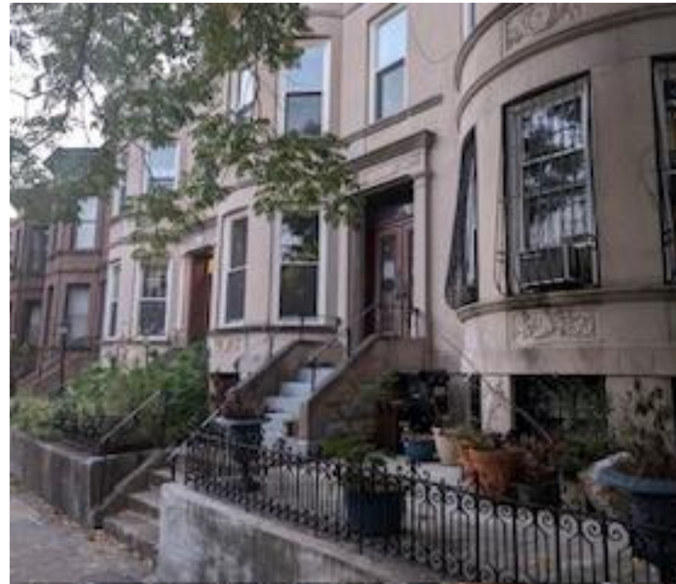
205 – 199 Maple – Looking to Bedford
