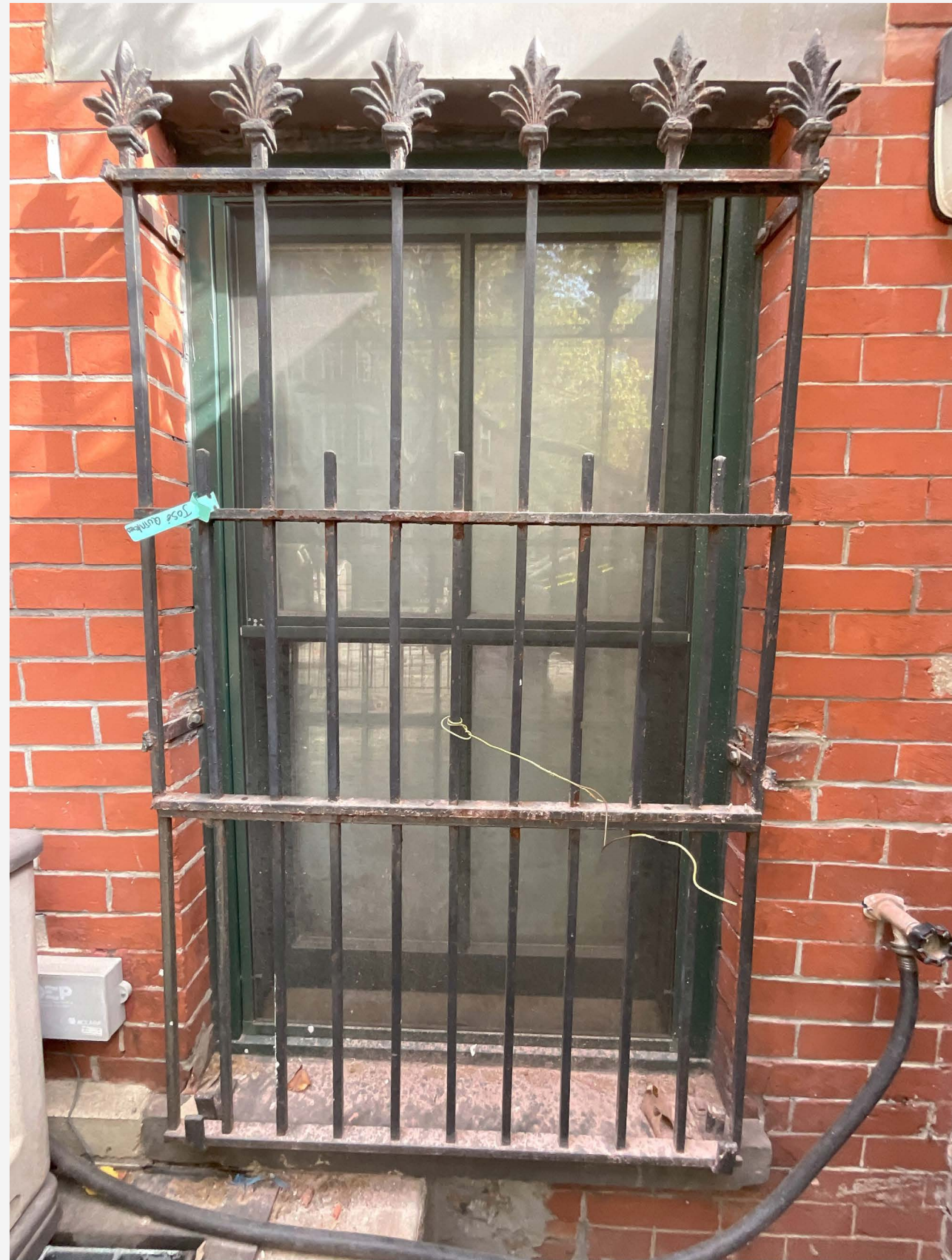
BASEMENT LEVEL WINDOW PHOTO
