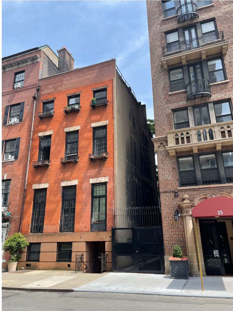
VIEW FROM 9TH STREET
