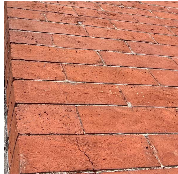
7. Hairline cracks and poor brick face condition are typical
