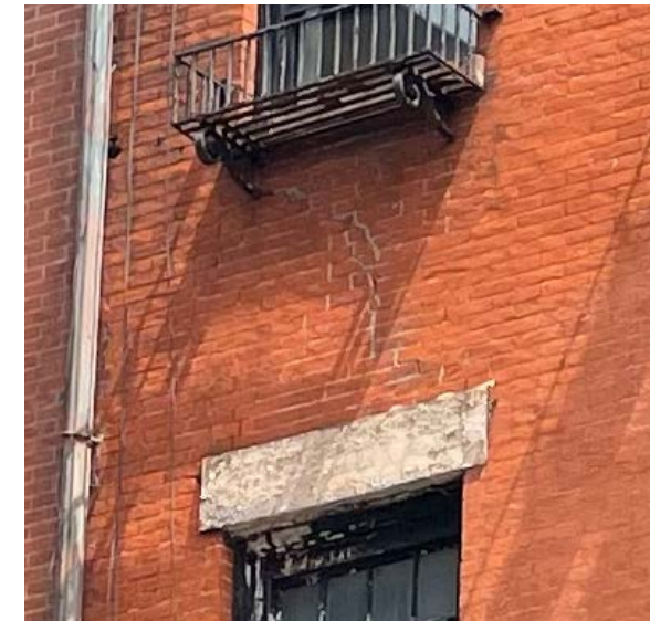
7. Hairline cracks and poor brick face condition are typical
