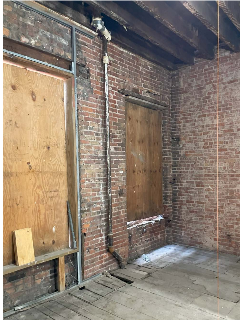
REAR WALL INTERIOR / Second Floor
