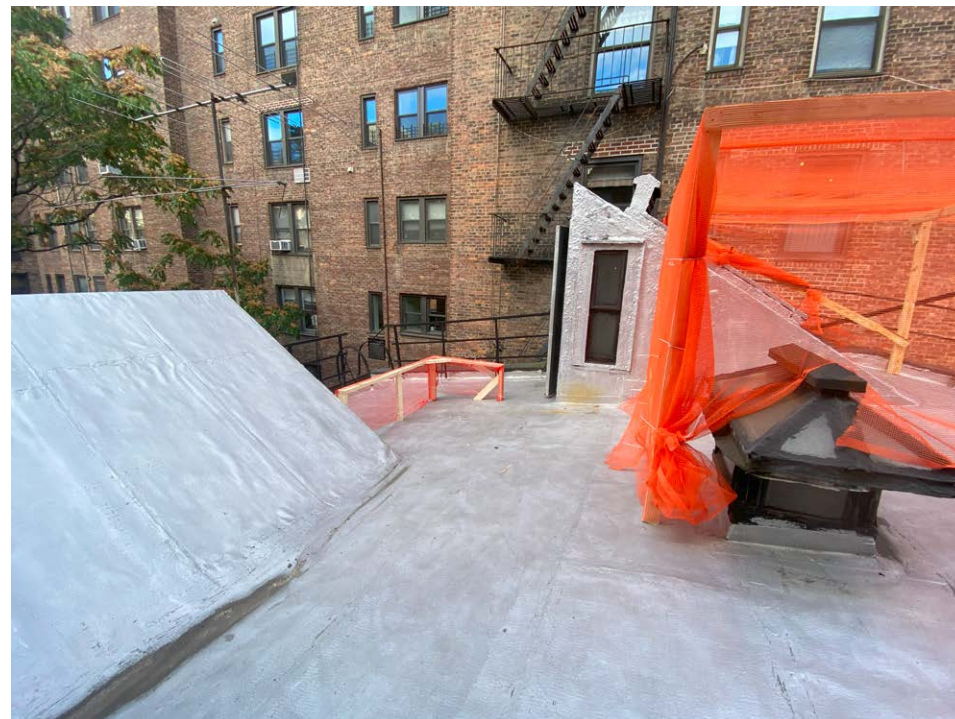
ROOF BULKHEAD AND RAILING / Looking East
