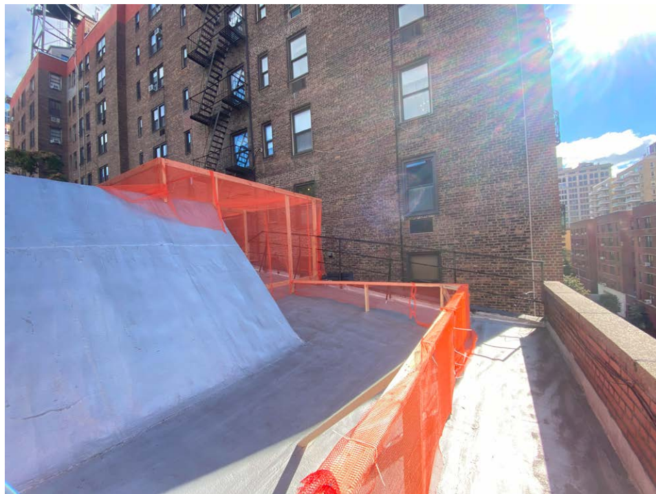
ROOF BULKHEAD AND RAILING / Looking East
