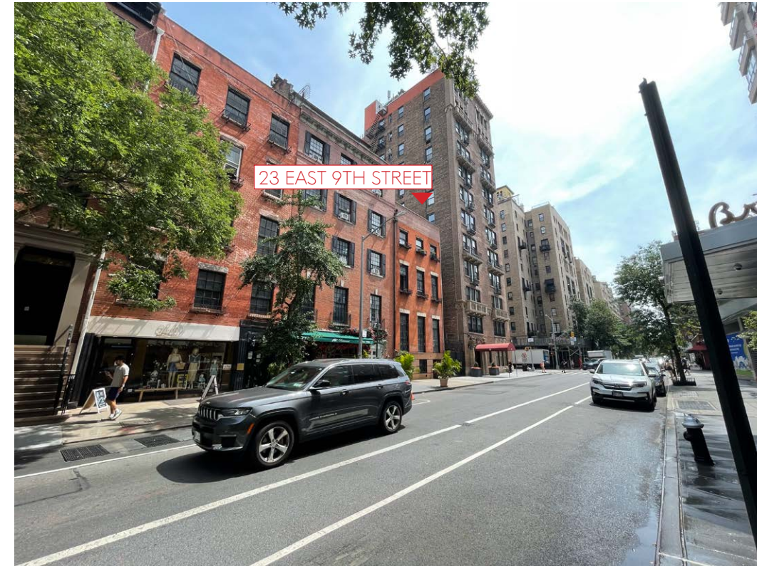
PROJECT LOCATION - STREET VIEW FROM E 9TH STREET LOOKING EAST
