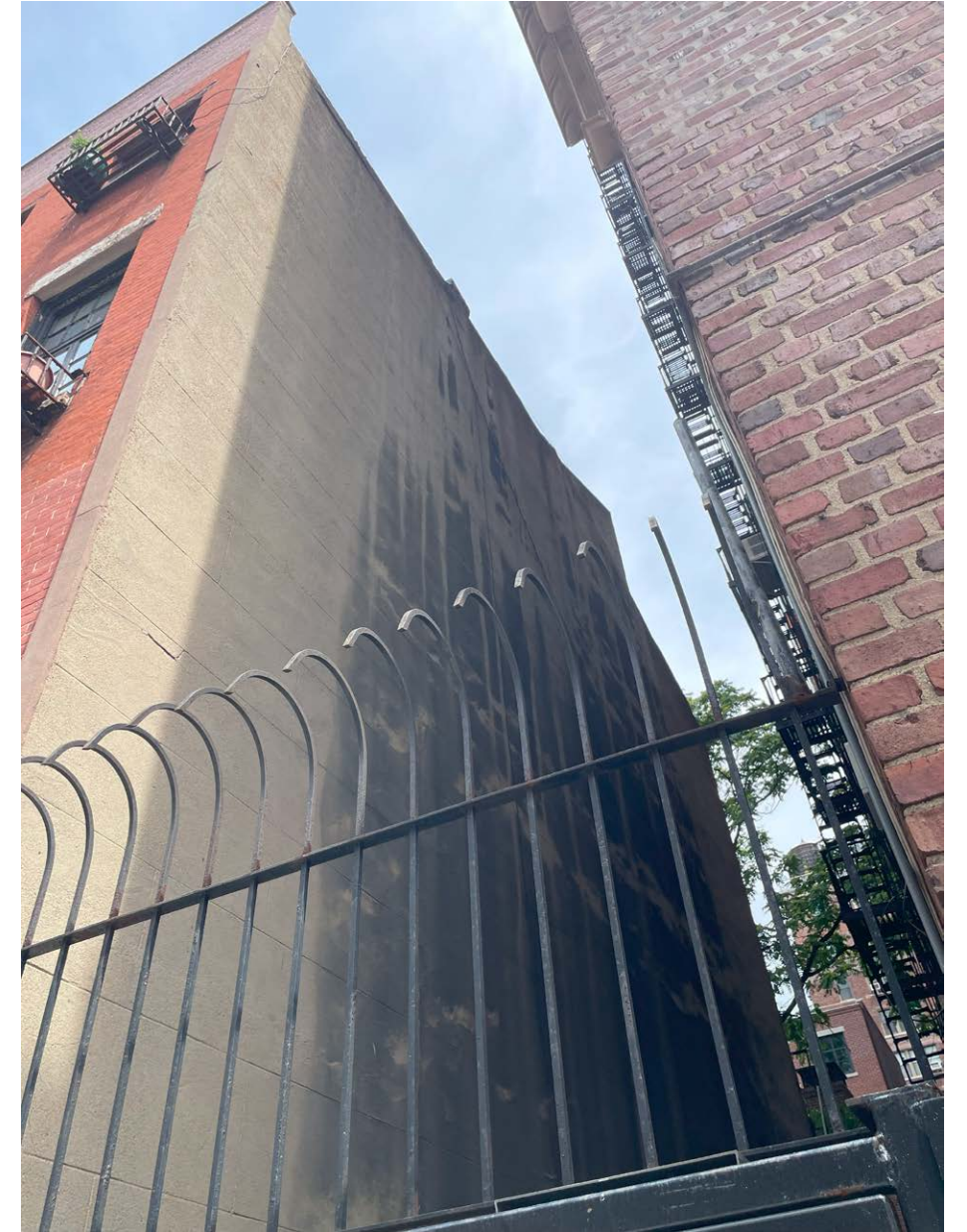
VIEW LOOKING UP AT GATE
