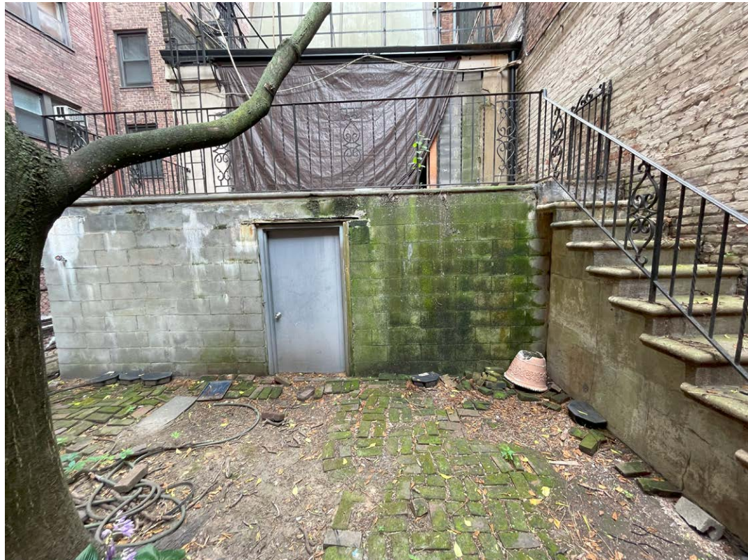
REAR YARD / Looking South
