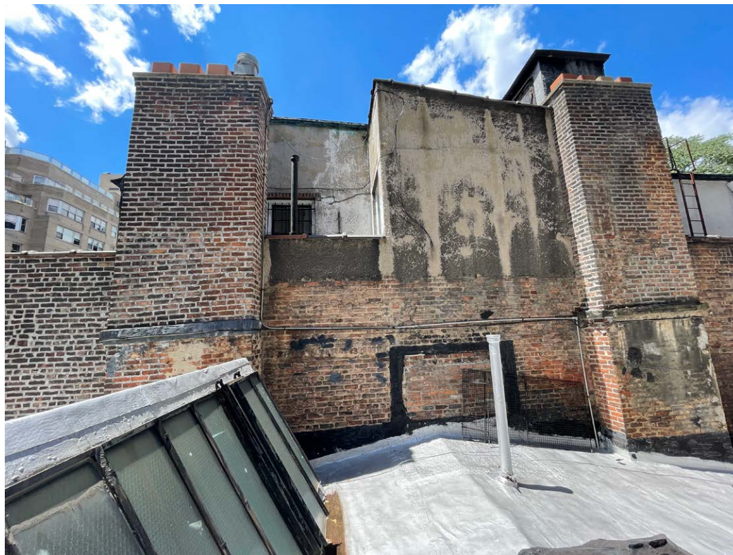
EXISTING CHIMNEYS / Looking West
