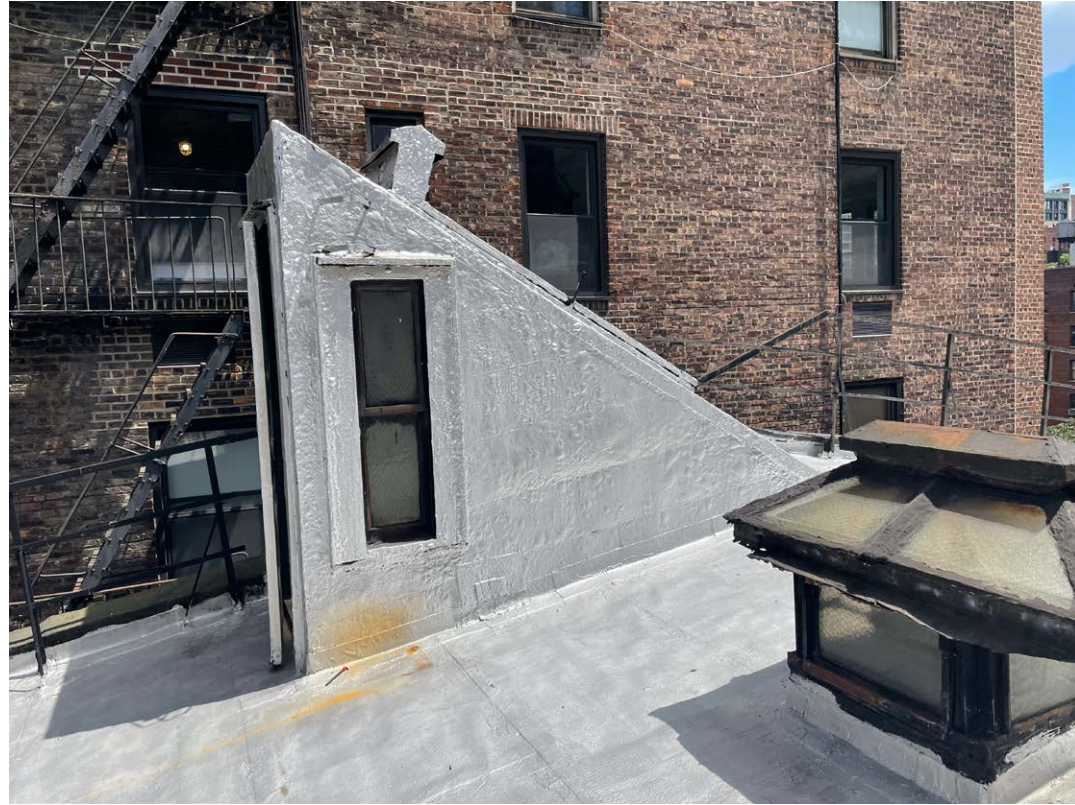
EXISTING STAIR BULKHEAD / Looking East
