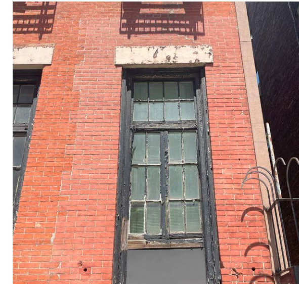
1. Brick repairs have been made with mismatched bricks
