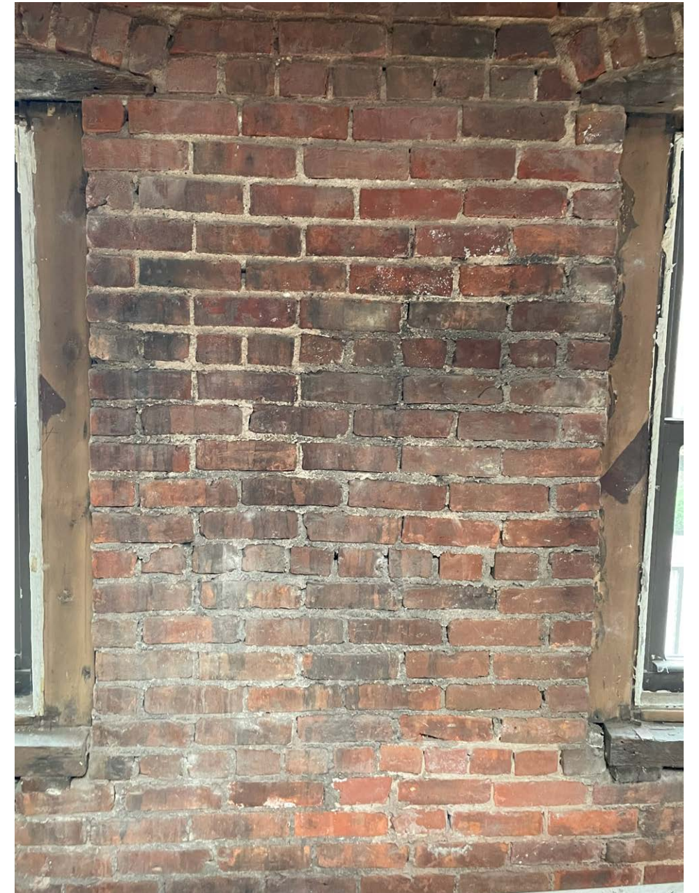
PRIMARY FACADE WALL INTERIOR / Third Floor
