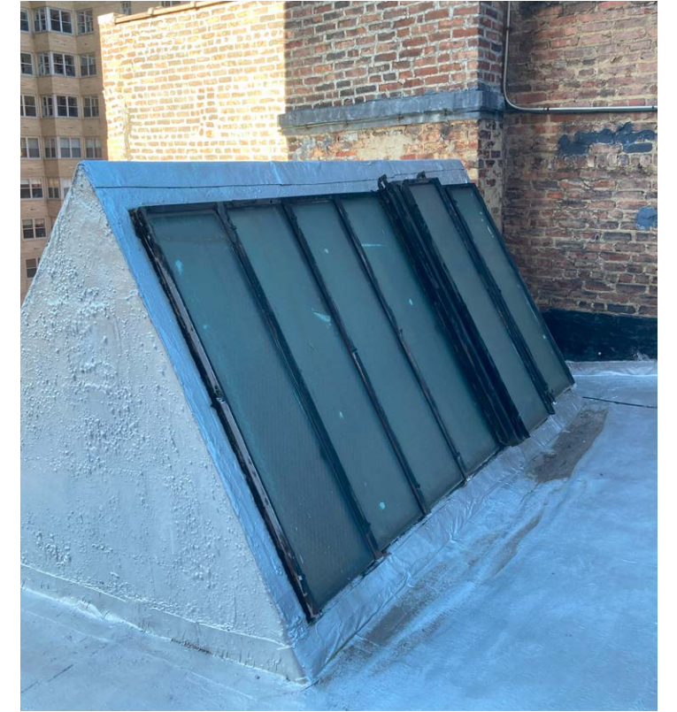
EXISTING SKYLIGHT BULKHEAD
