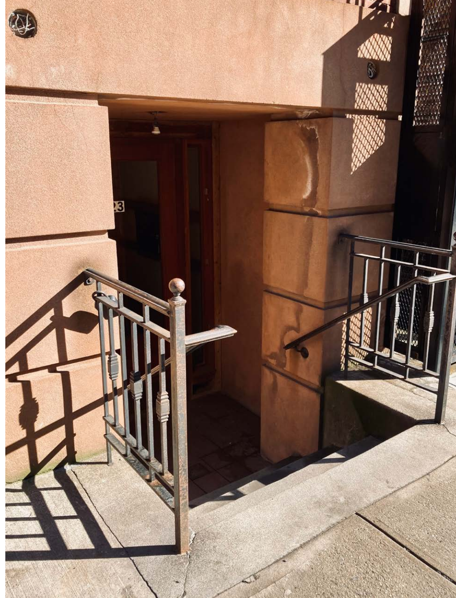
EXISTING ENTRY FROM STREET
