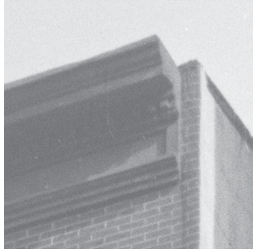
CORNICE DETAIL FROM 1940 TAX PHOTO
