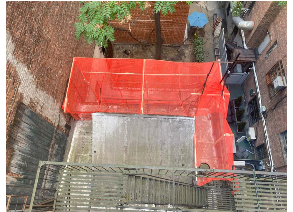
REAR EXTENSION / Looking Down from Roof
