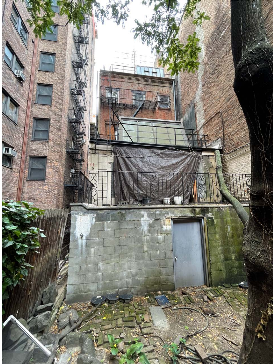
EXISTING CONDITIONS / Basement
