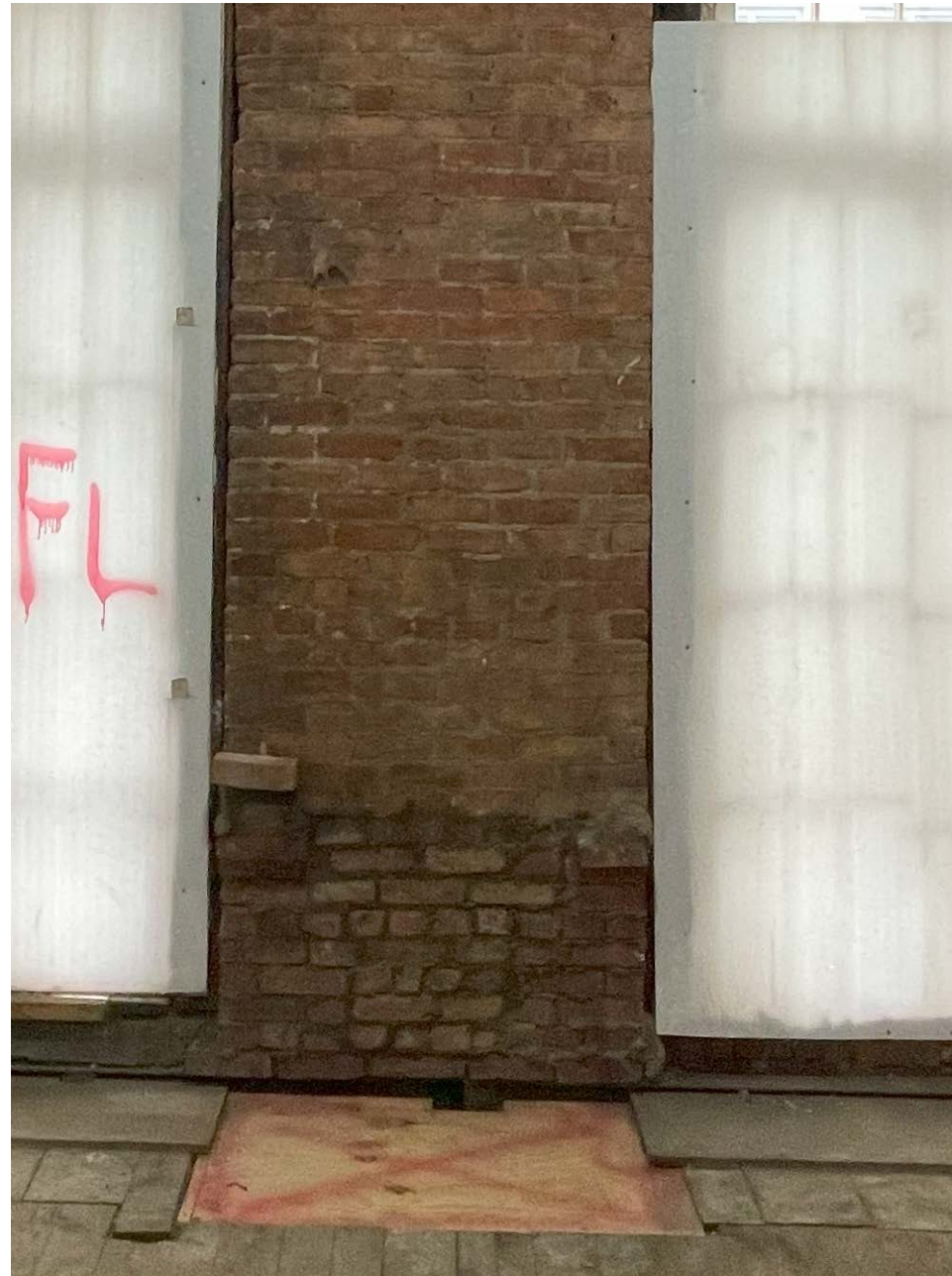
PRIMARY FACADE WALL INTERIOR / First Floor
