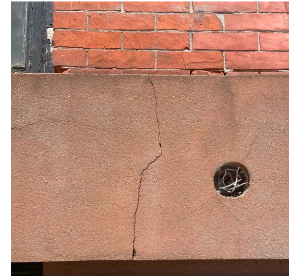
5. Broken brick units and holes are common across the facade
