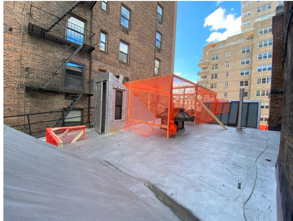
ROOF BULKHEAD AND RAILING / Looking South
