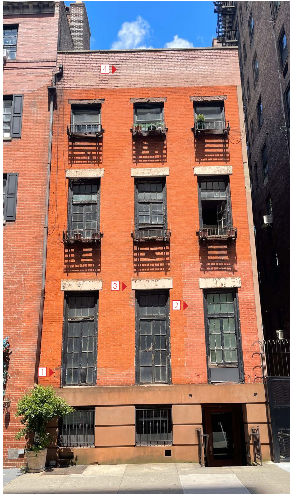
EAST 9TH STREET FACADE
