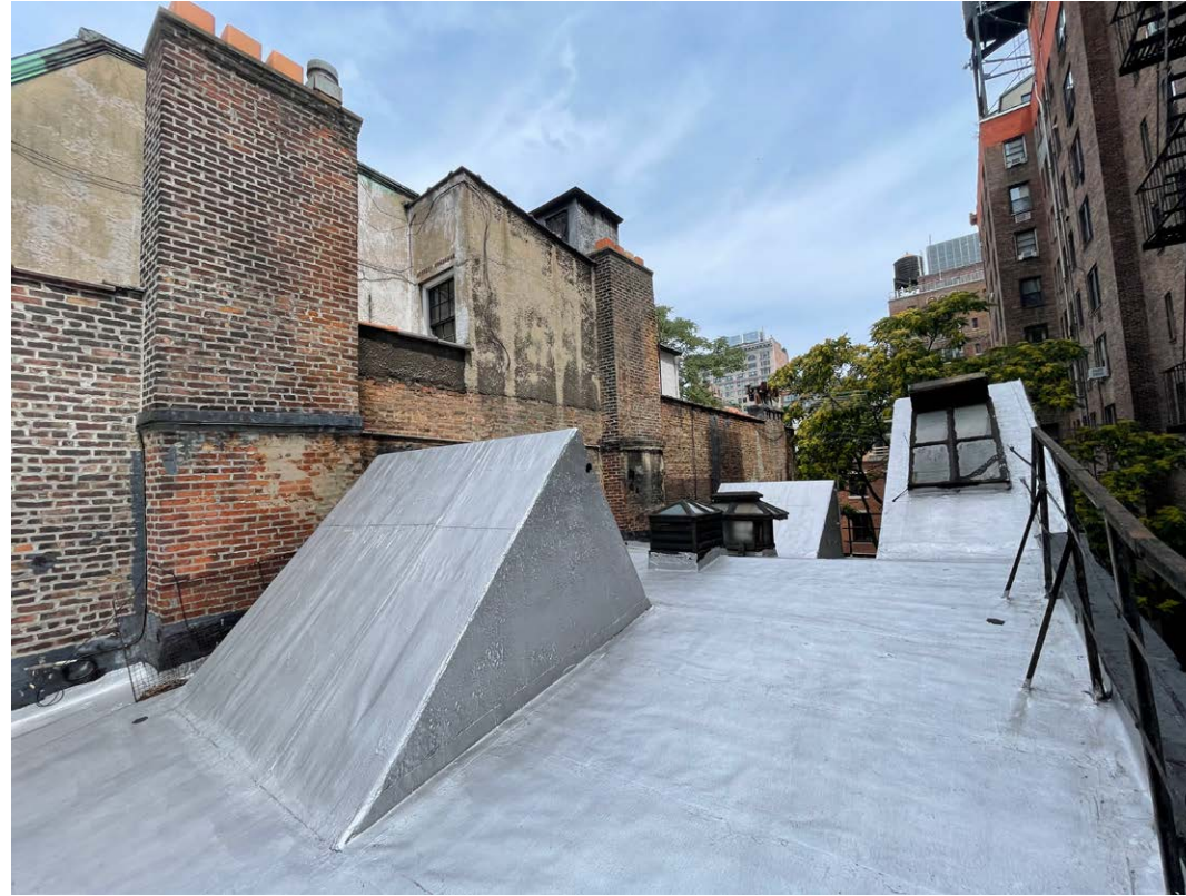
EXISTING SKYLIGHT BULKHEADS / Looking North
