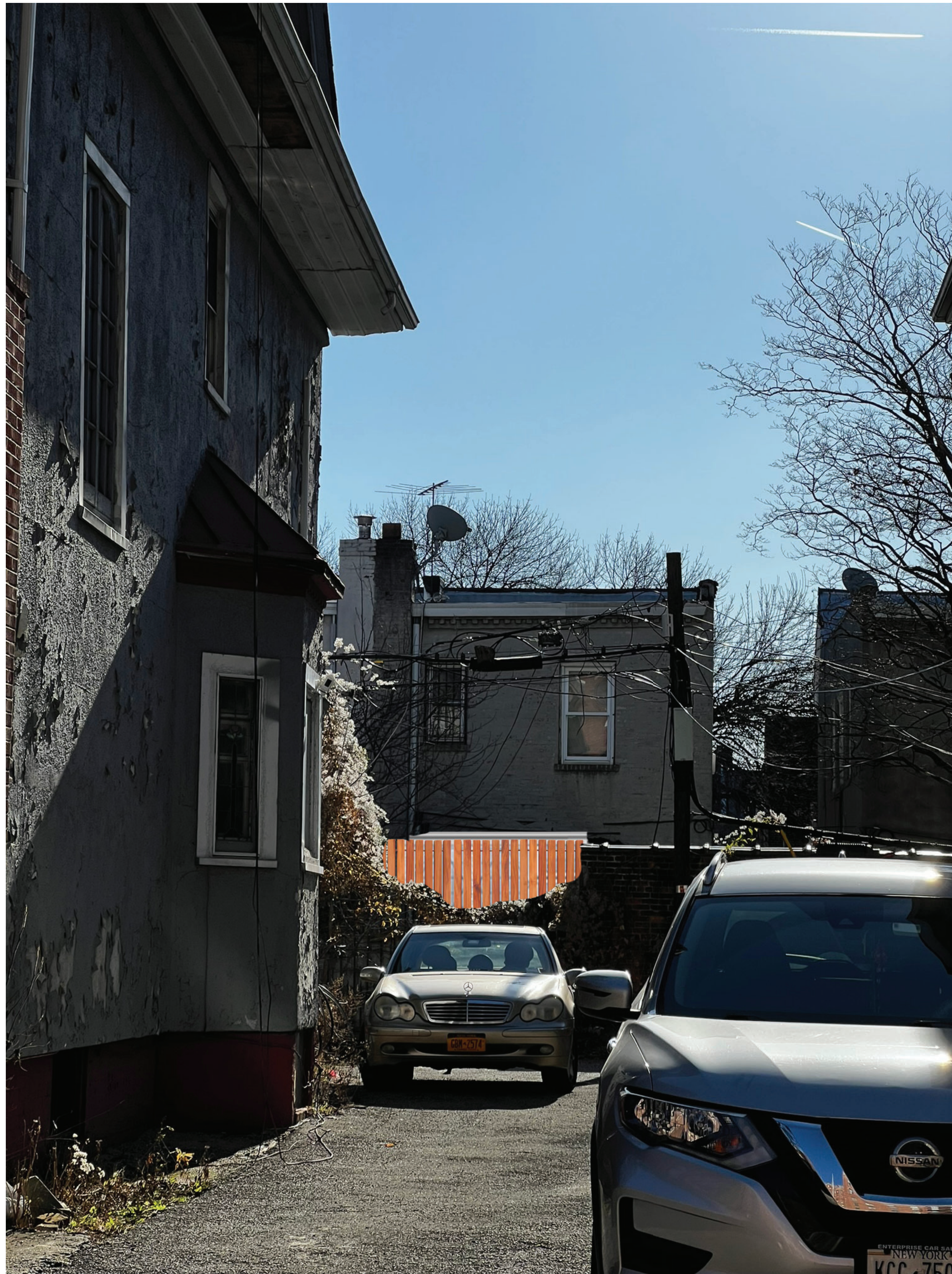
VIEW OF 25 MAPLE STREET REAR FACADE FROM 86 LINCOLN ROAD- PROPOSED 6'-0" HIGH CEDAR FENCE - 105' FEET AWAY
