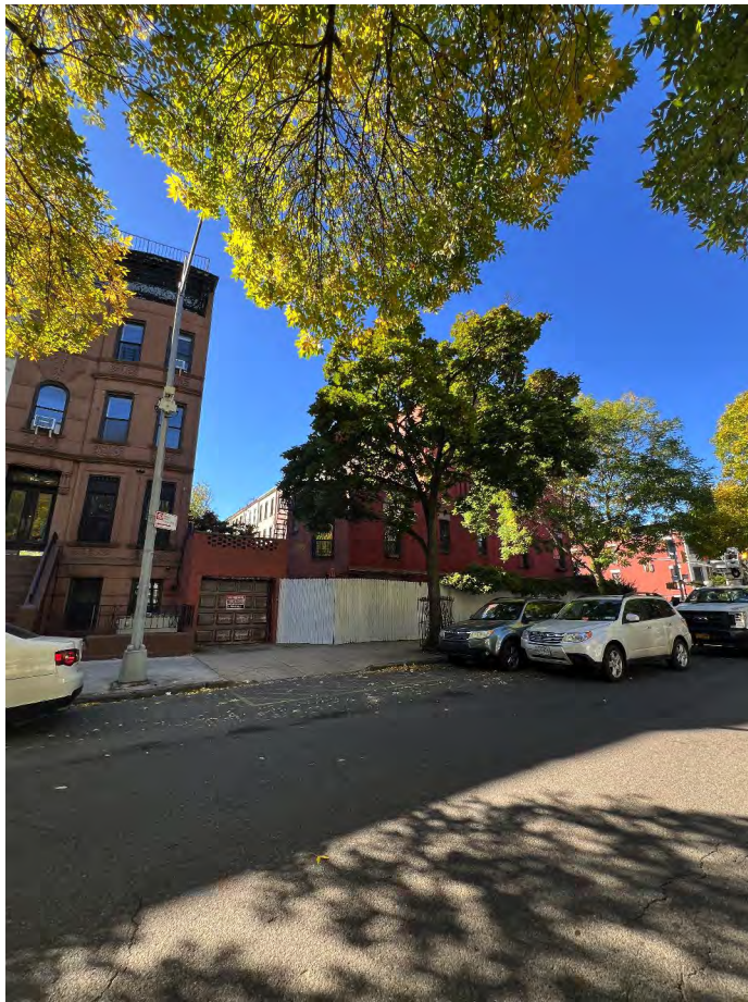
63 UNDERHILL AVE. - CORNER BUILDING
