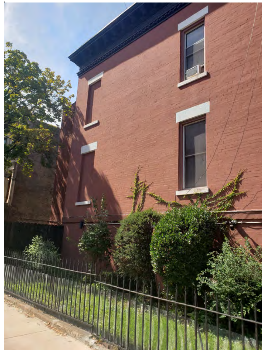
PHOTO OF REAR SIDE OF SIDE ELEVATION (UNDERHILL AVE.) - EXISTING CONDITIONS
