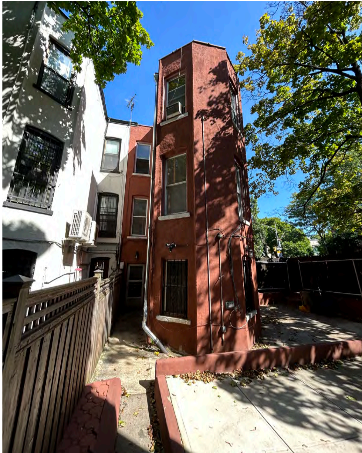
PHOTO OF REAR YARD ELEVATION - EXISTING CONDITIONS
