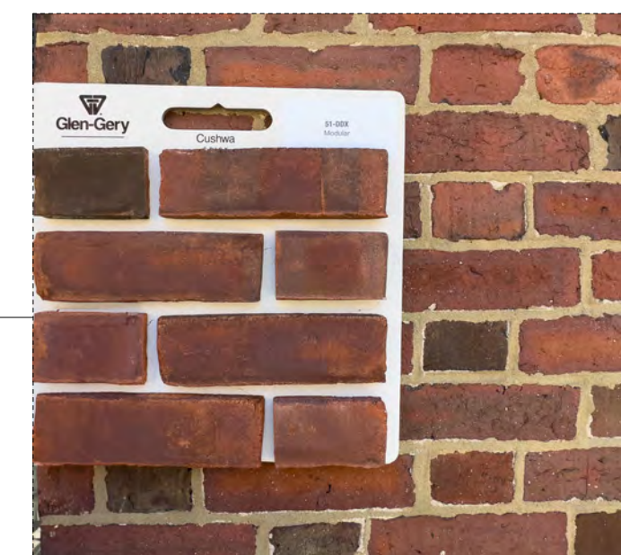
B01- RED BRICK GLEN-GERY CUSHWA 51-DDX MODULAR. TO MATCH EXISTING UPPER FLOORS. FLEMISH BOND PATTERN
