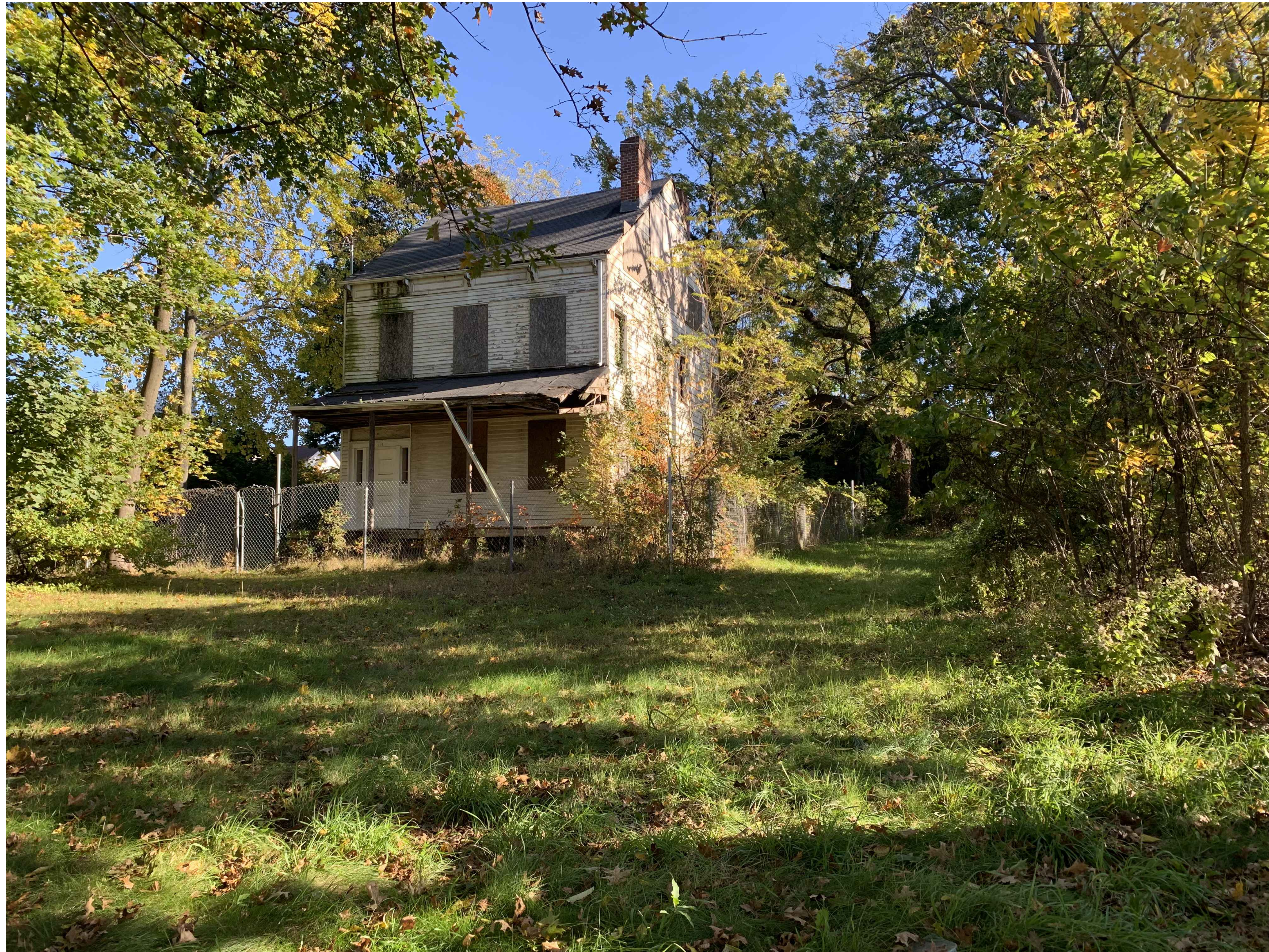
CLOSE UP VIEW JKV HOUSE LOOKING NORTHERLY
