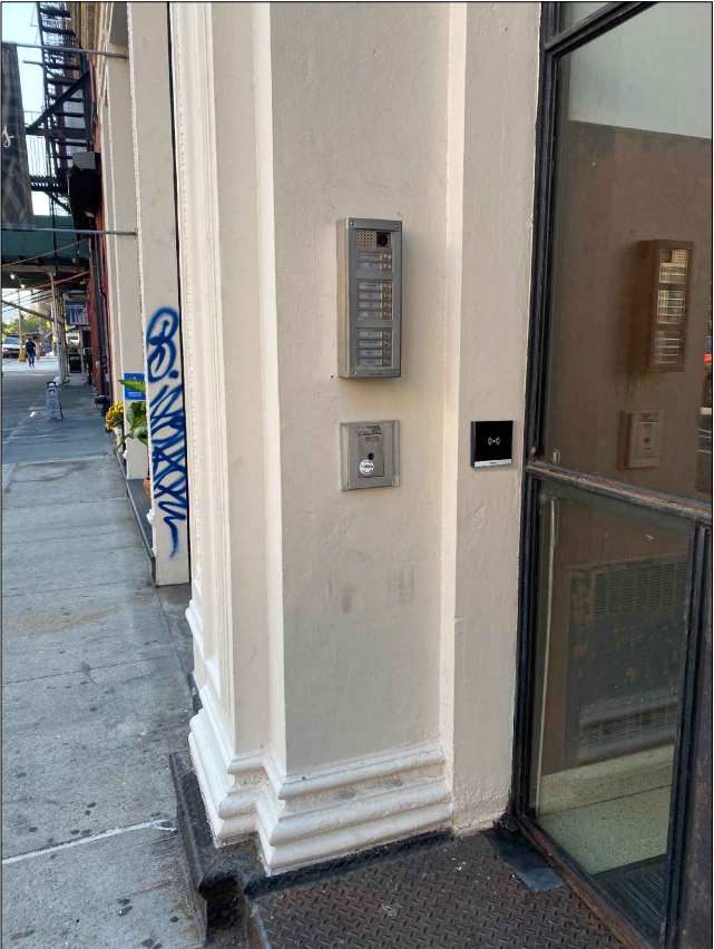
Location of new card reader to be installed at Storefront #4.
