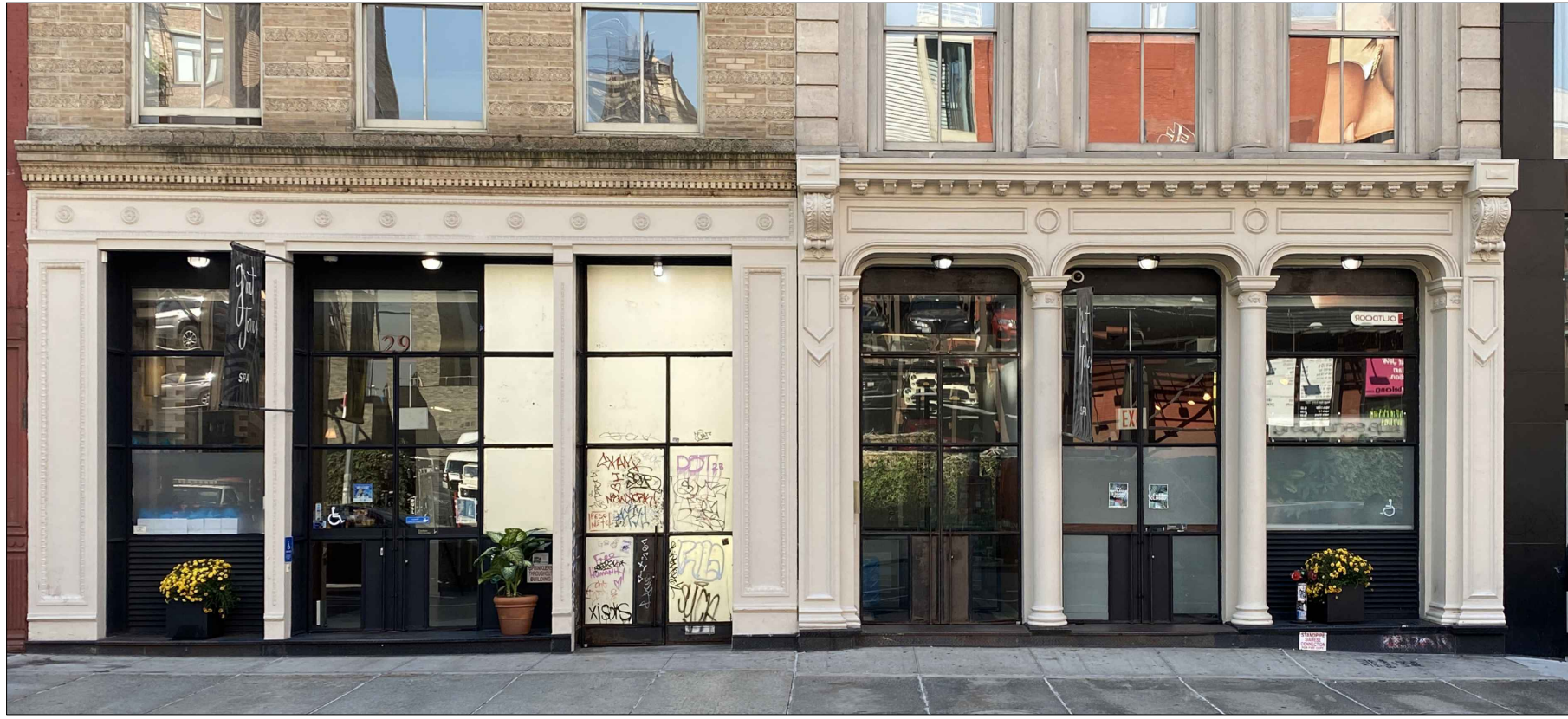
CLOSE UP OF CURRENT CONDITIONS AT FIRST FLOOR 2023
