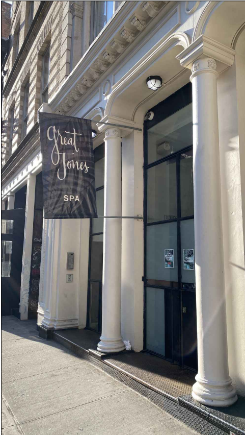
Existing light fixtures.
