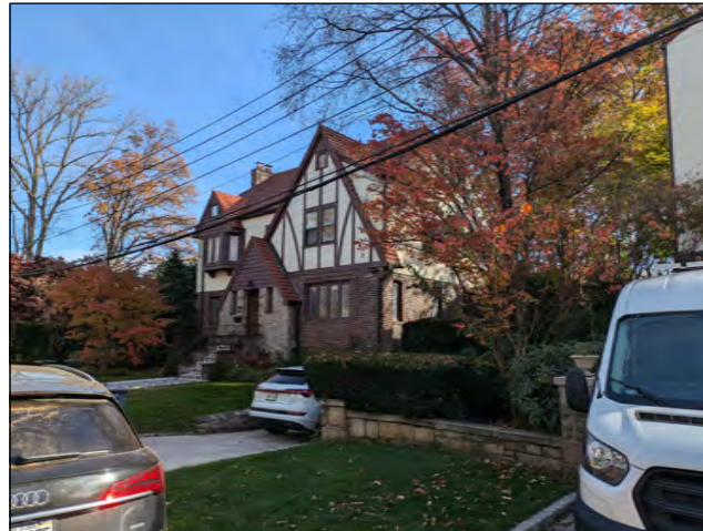
D VIEW NORTH SIDE FACADE NOT VISIBLE
