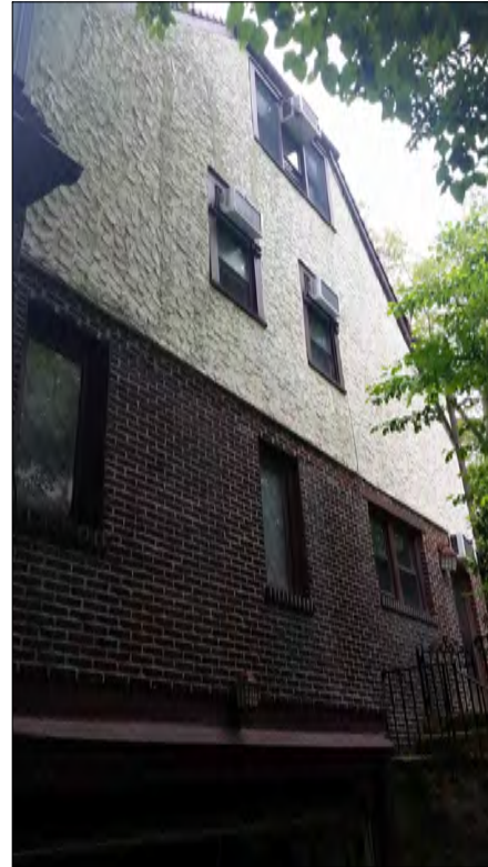
C - SOUTH SIDE FACADE
