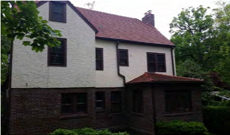
B - EAST REAR FACADE
