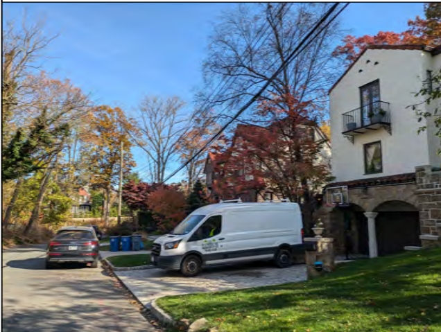
C VIEW NORTH SIDE FACADE NOT VISIBLE
