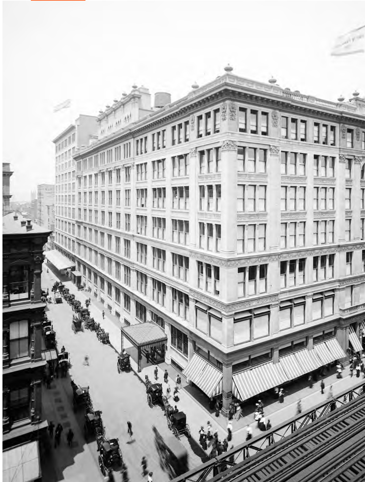
Canopies, vestibule and awnings, 1903 (Museum of the City of New York)
