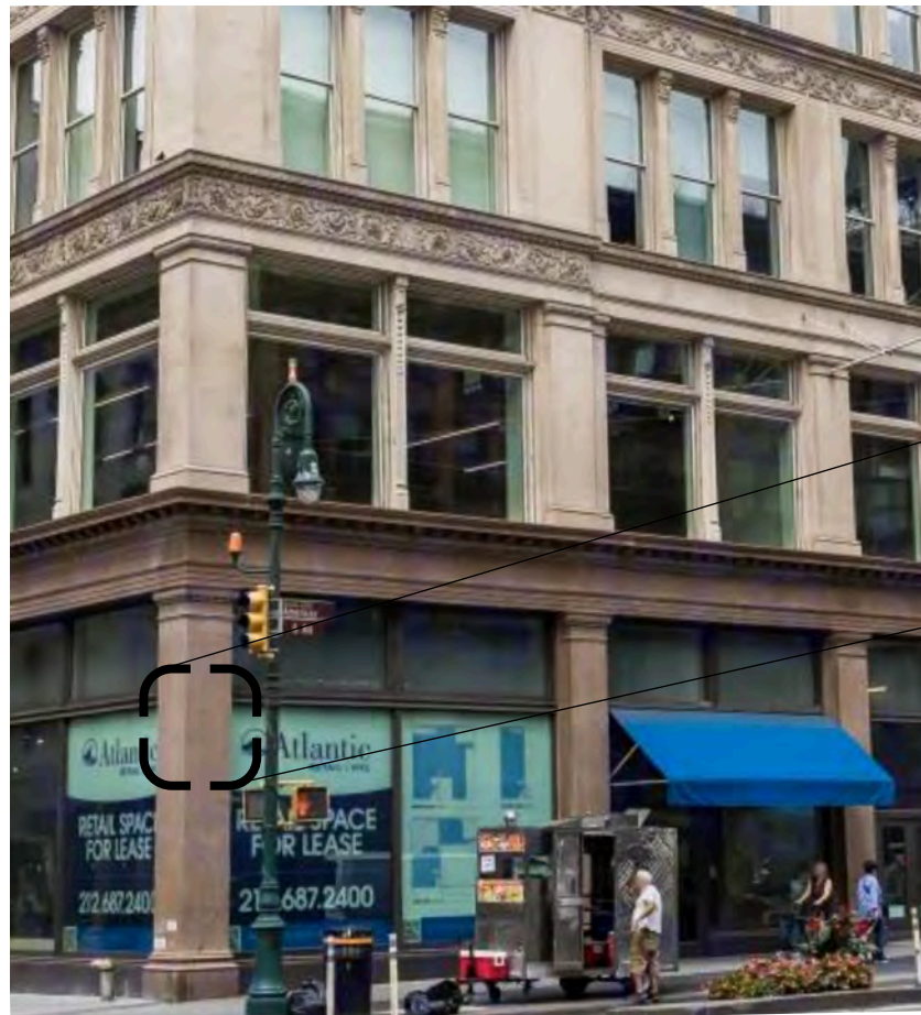
EXISTING CORNER CONDITION
