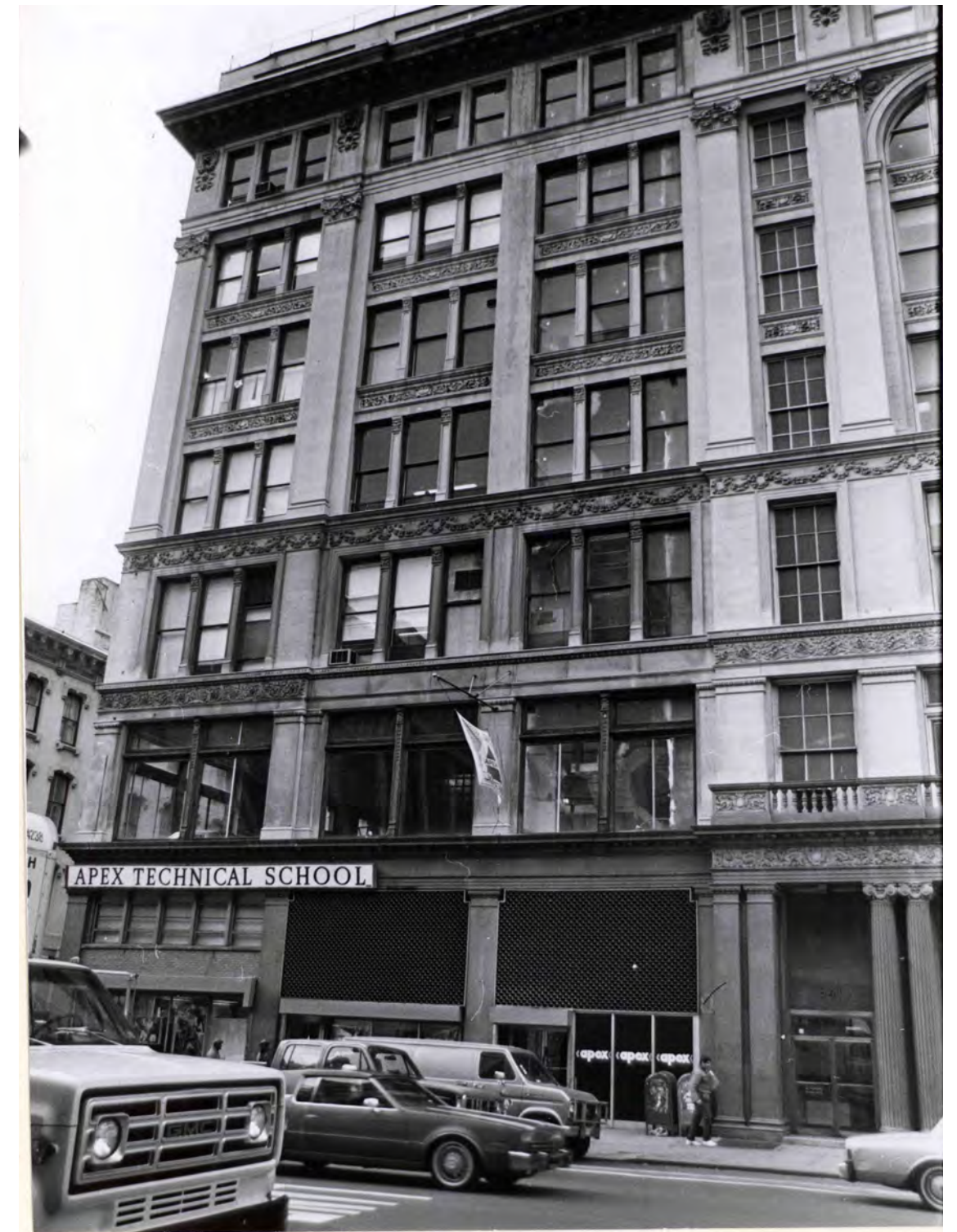
LPC Designation Photo, 1989
