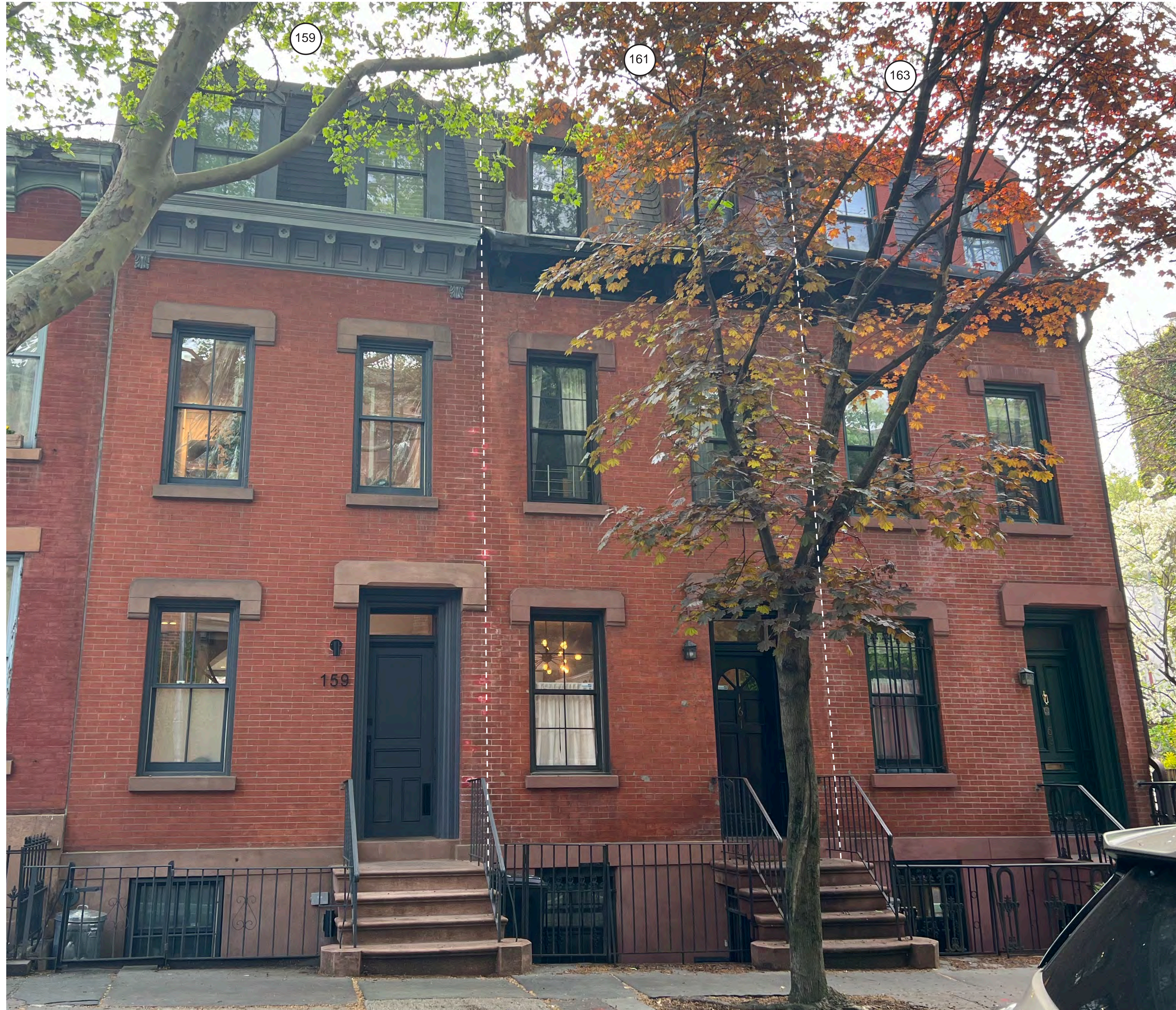
EXISTING FRONT FACADE - LOOKING EAST
