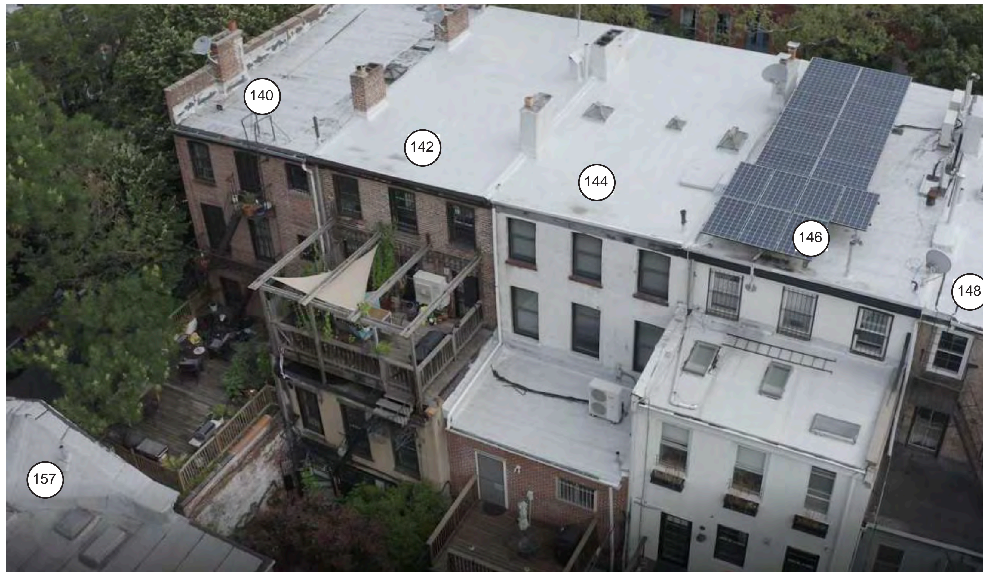
(A) NEIGHBORING REAR FACADES - LOOKING NORTH TOWARDS BERGEN STREET
