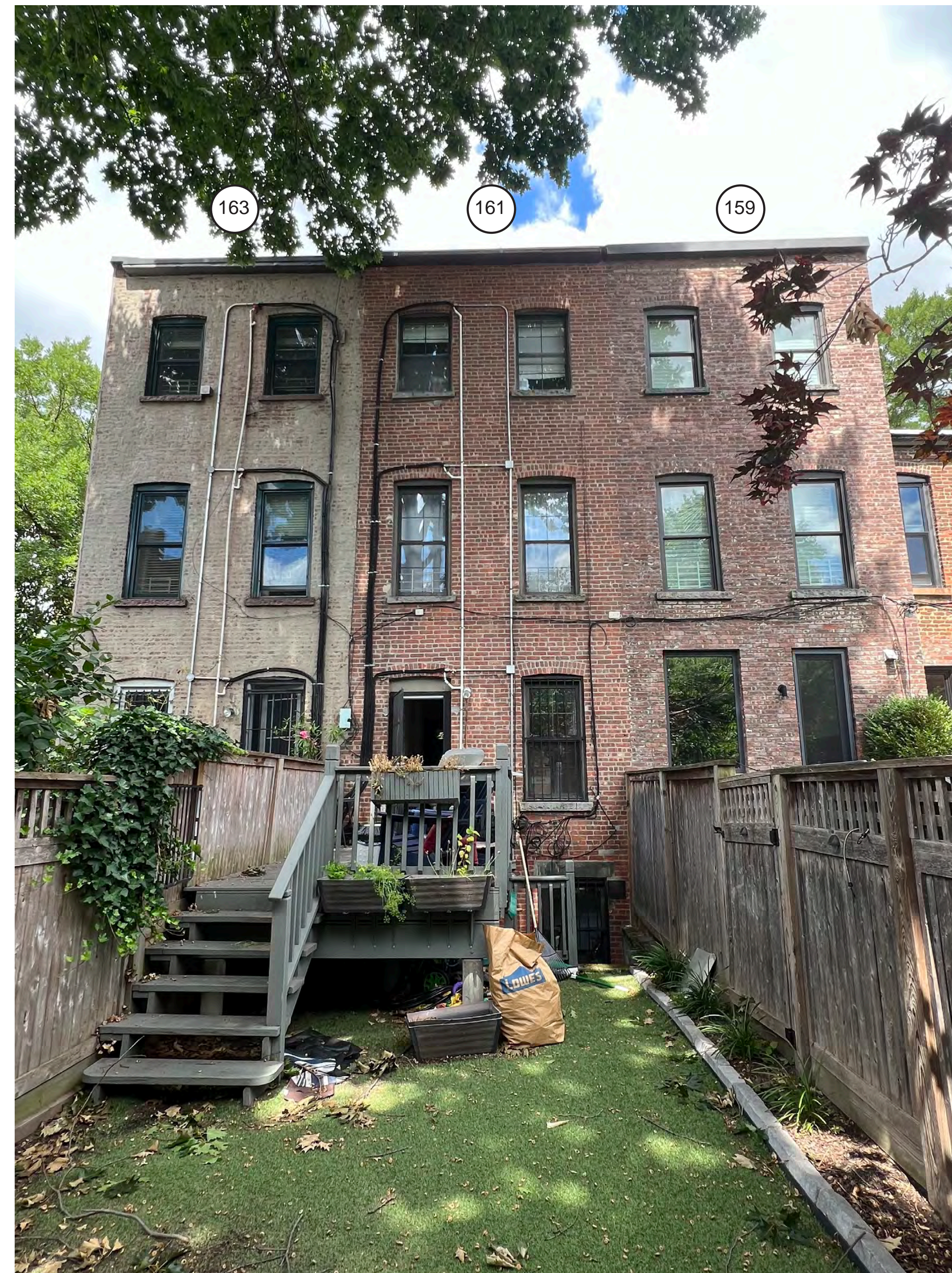
EXISTING REAR FACADE
