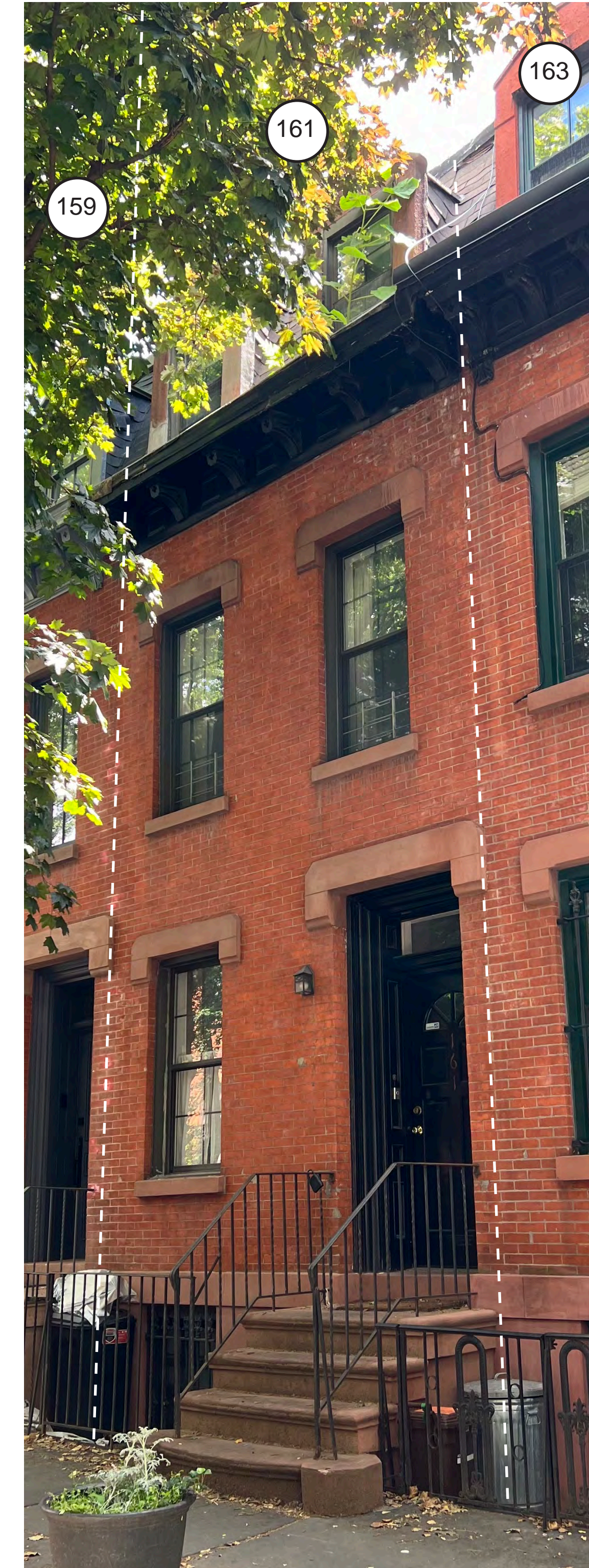
EXISTING FRONT FACADE - LOOKING EAST
