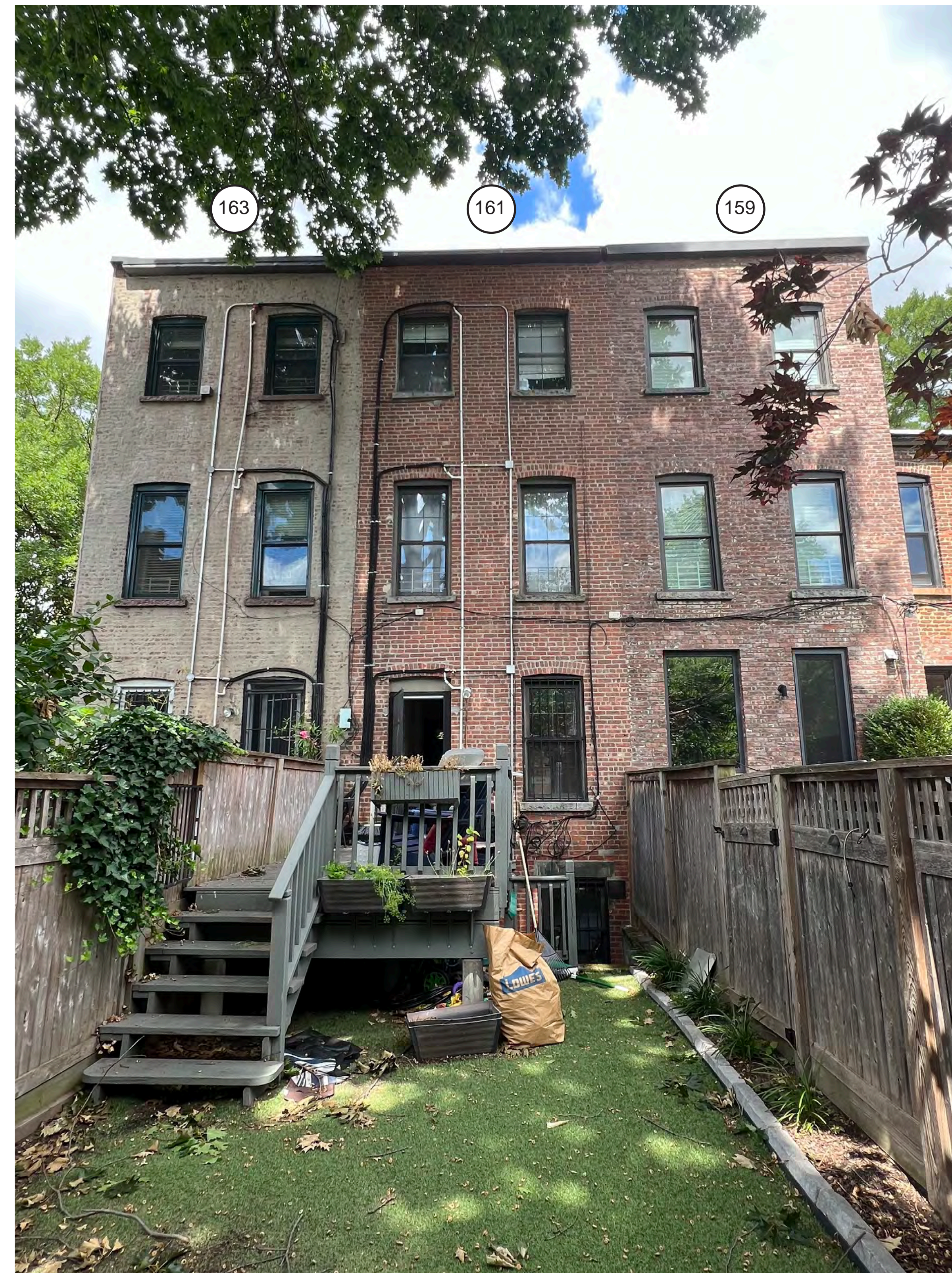
EXISTING REAR FACADE
