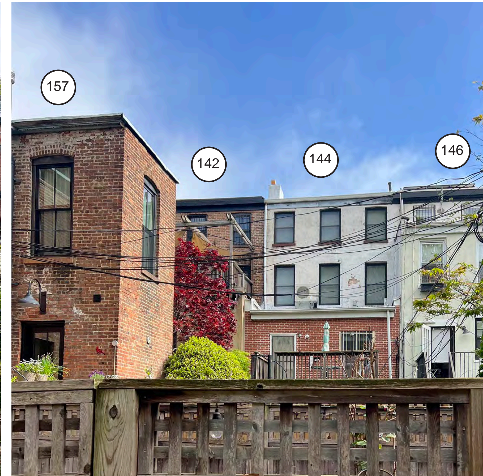
(E) NEIGHBORING REAR FACADES - LOOKING NORTH
