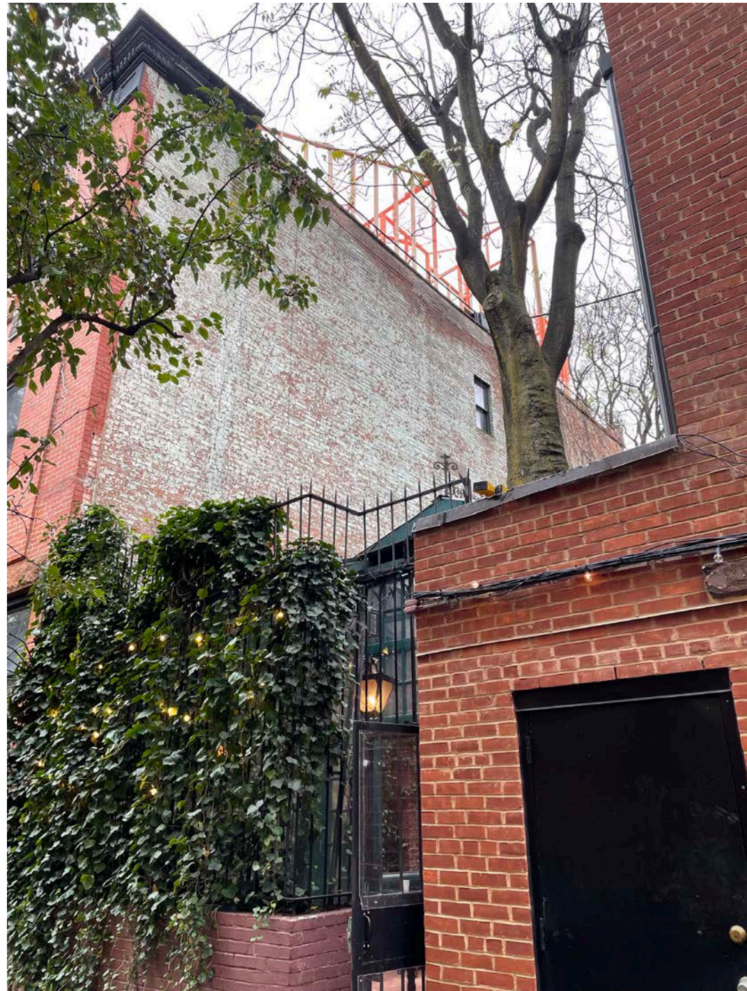
1: View w/ Mockup - View Looking South at Corner of 244 Waverly
