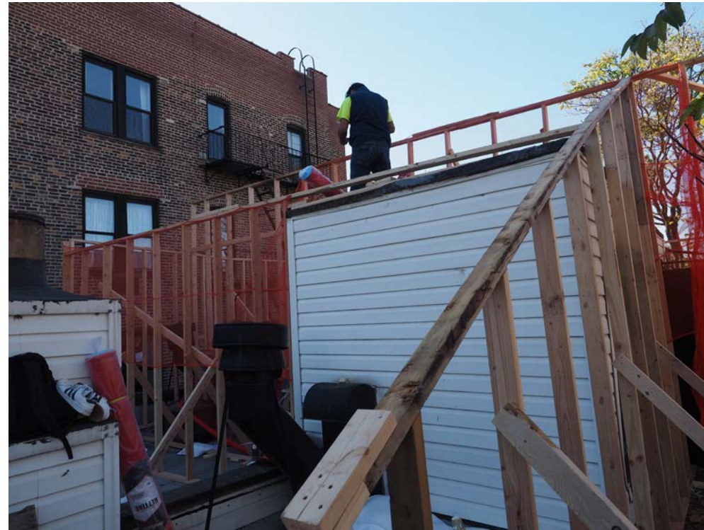
4: View of Mockup at Roof
