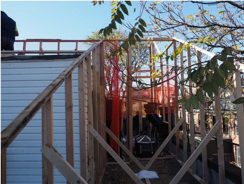
3: View of Mockup at Roof
