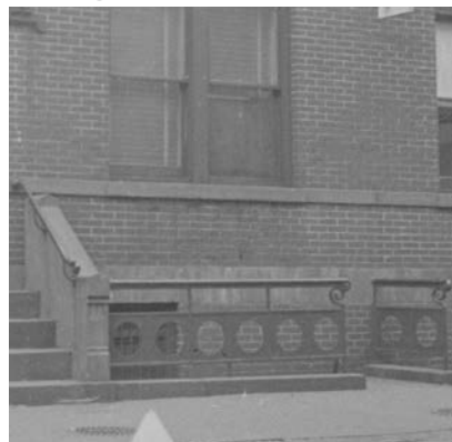
Areaway Gate Used As Model For New Gate
