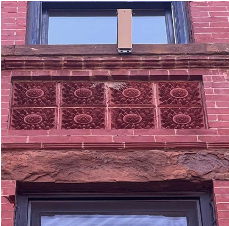
Existing Terracotta Block Panels
