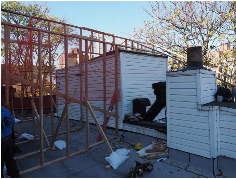
1: View of Mockup at Roof
