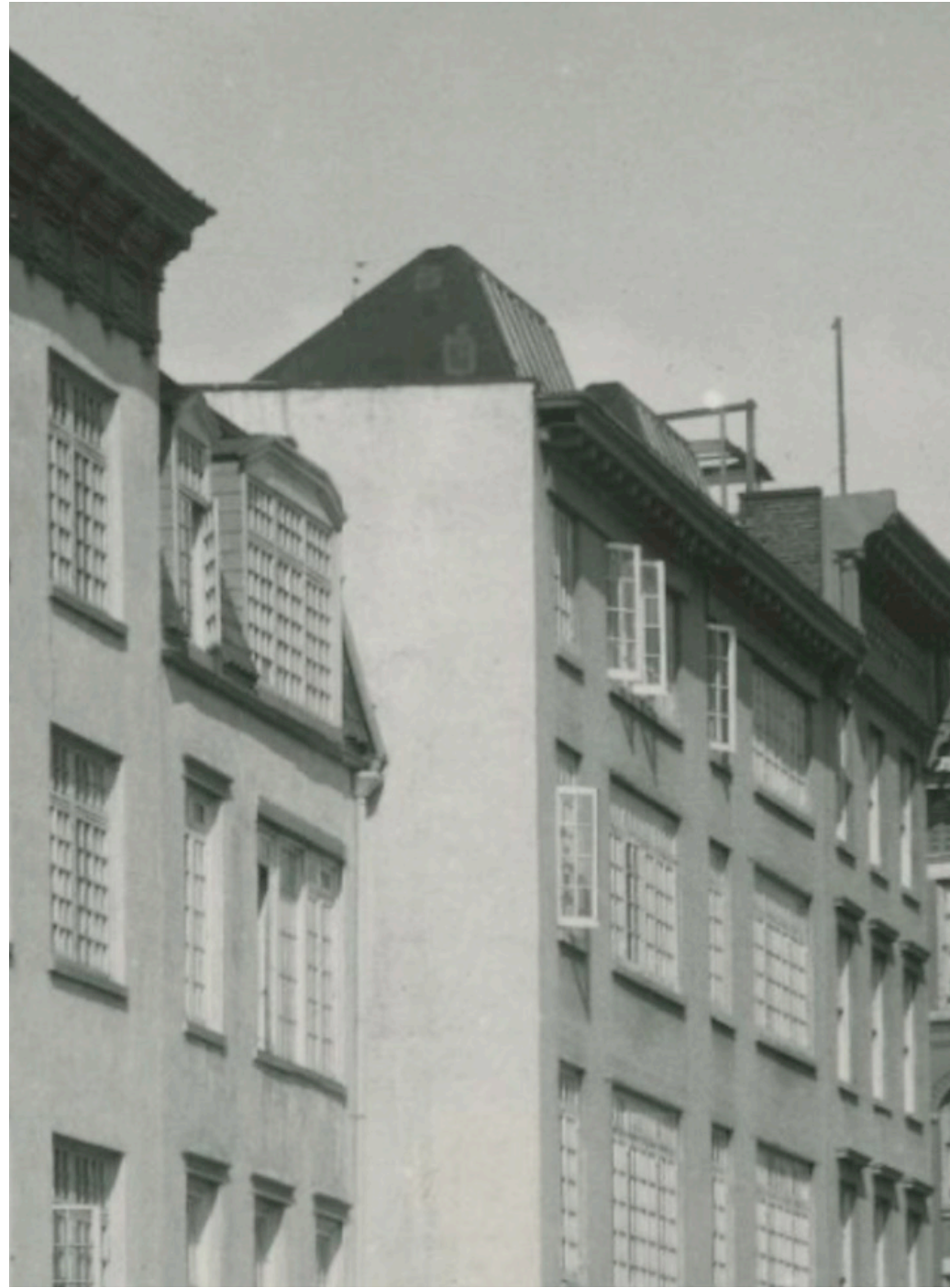
Washington Square South - 1920s Example of Studio Window (NYU Archives)
