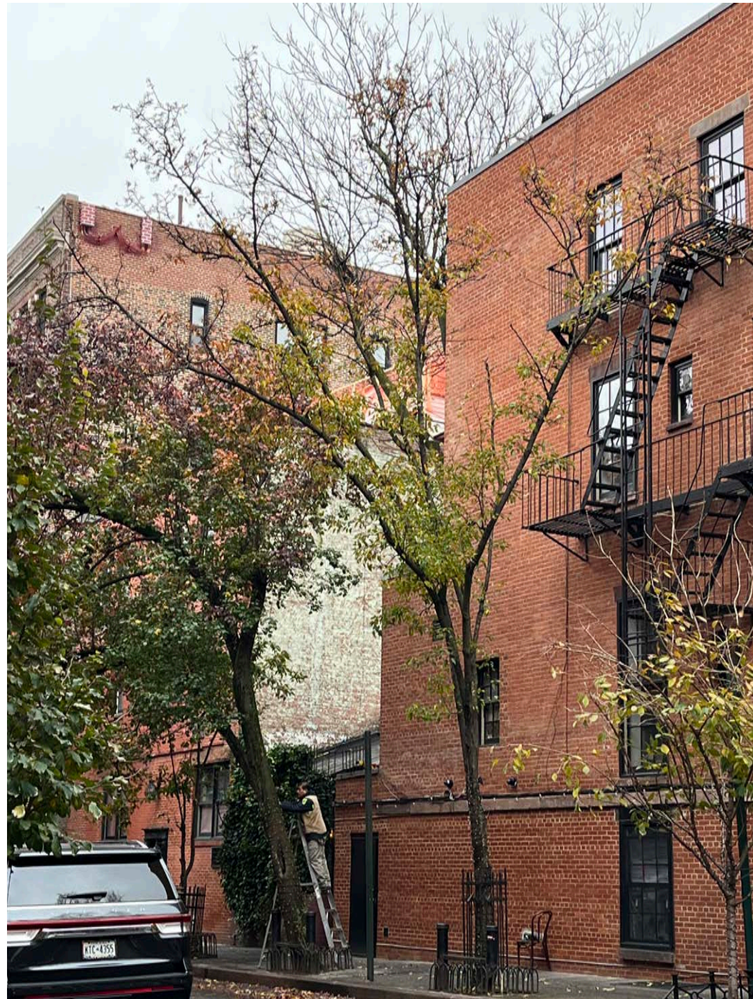
1: View of Mockup - View Looking South From Far Corner of Bank St. & Waverly Place
