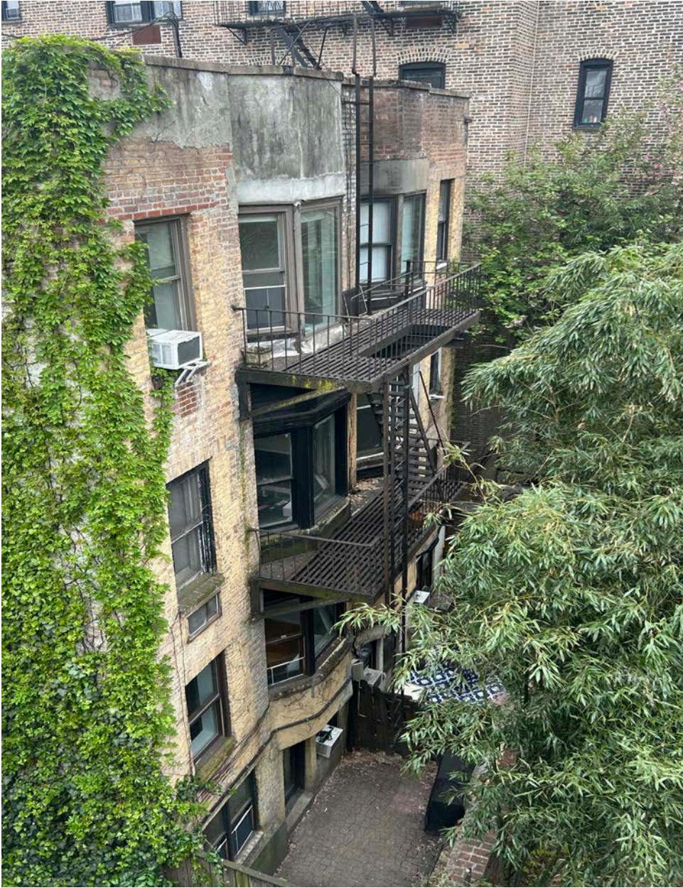
Overall View of Rear Elevation
