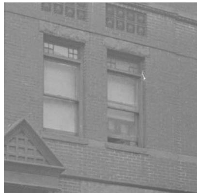
Rough Hewn Lintels And Windows Enlarged to Original Size w/ Divided Lites
