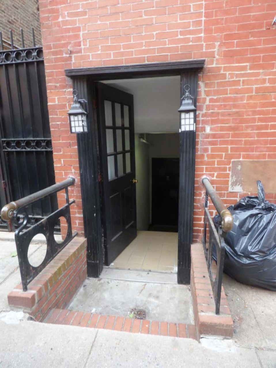
Existing south entrance
