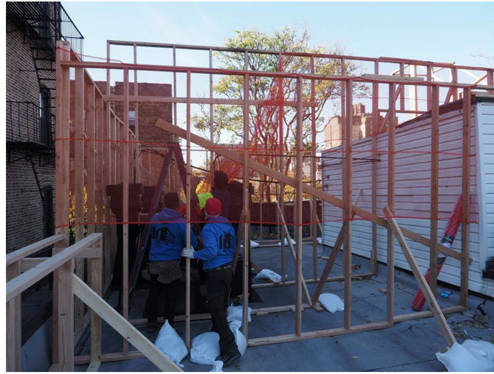
2: View of Mockup at Roof
