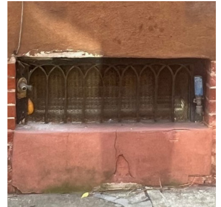
Metal Grate at Original Areaway Openings
