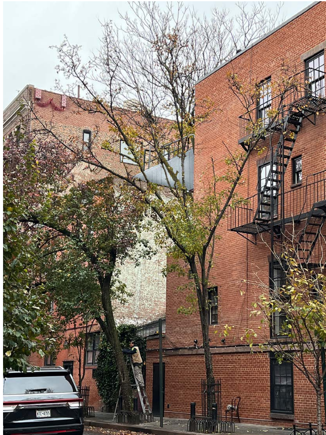
1: View w/ Rendering Over Mockup - View Looking South From Far Corner of Bank St. & Waverly Place
