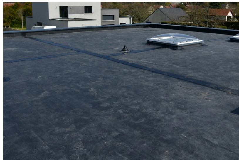
Flat Membrane roof
