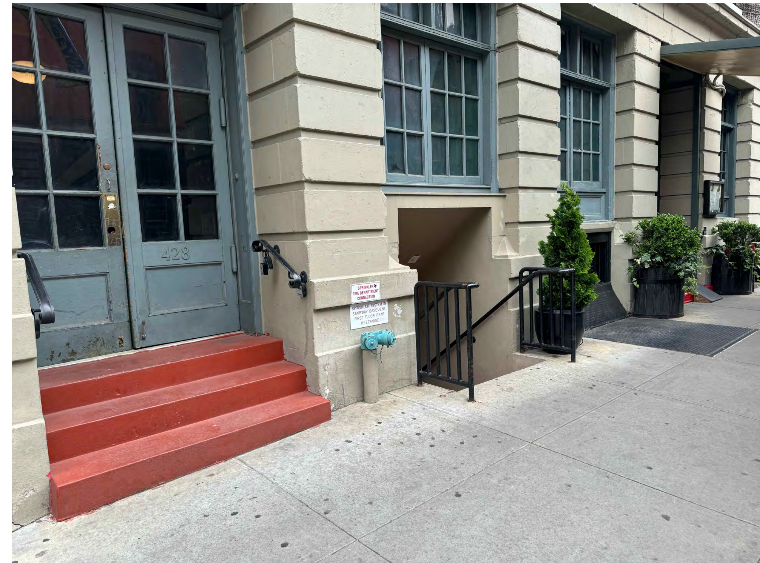
6 EXISTING FACADE SCALE: NTS
