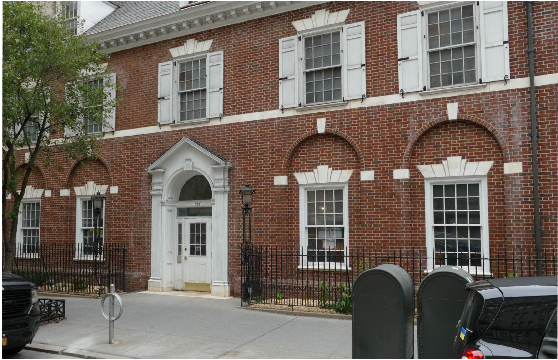
VIEW OF THE MADISON AVENUE FACADE
