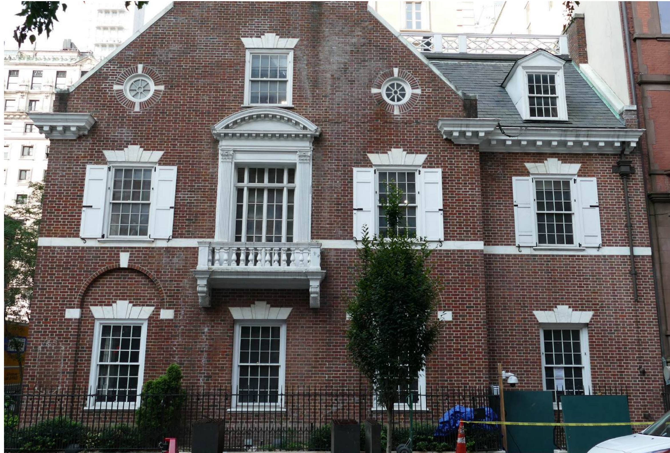
VIEW OF THE EAST 64TH STREET FACADE
