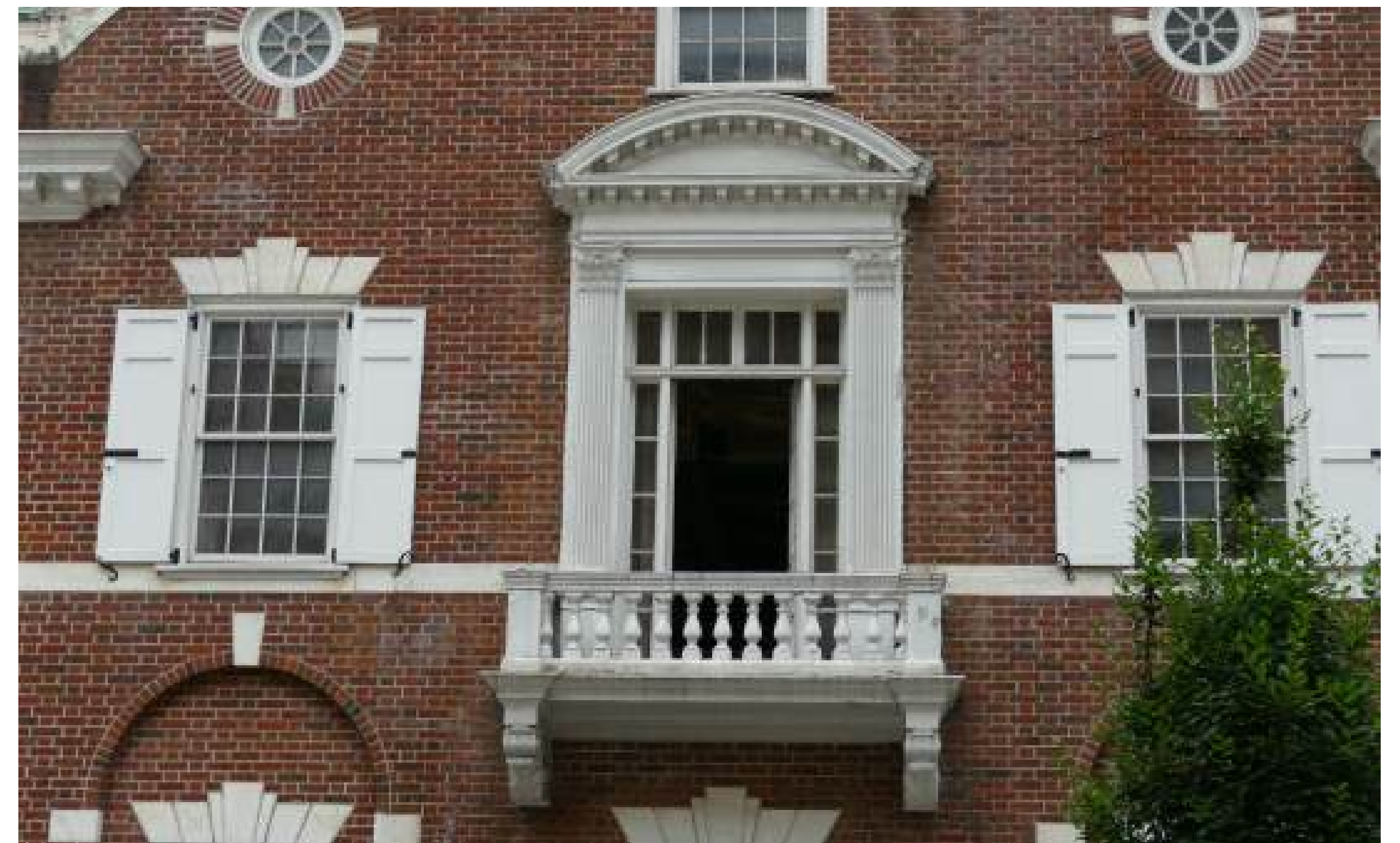
DETAIL VIEW OF WOOD WINDOWS AND JULIET BALCONY ON EAST 64TH STREET
