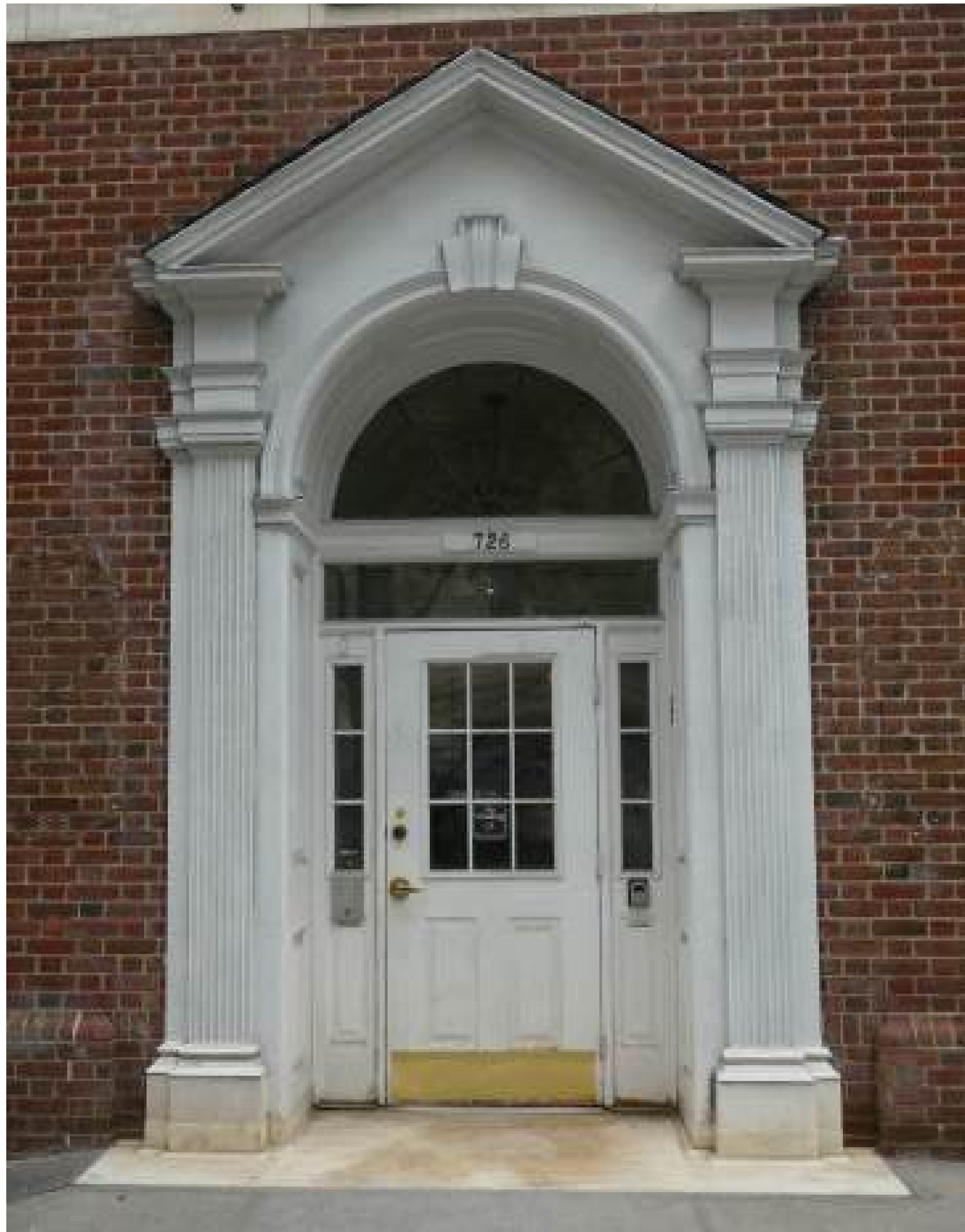
MAIN ENTRANCE DOOR MADISON AVENUE
