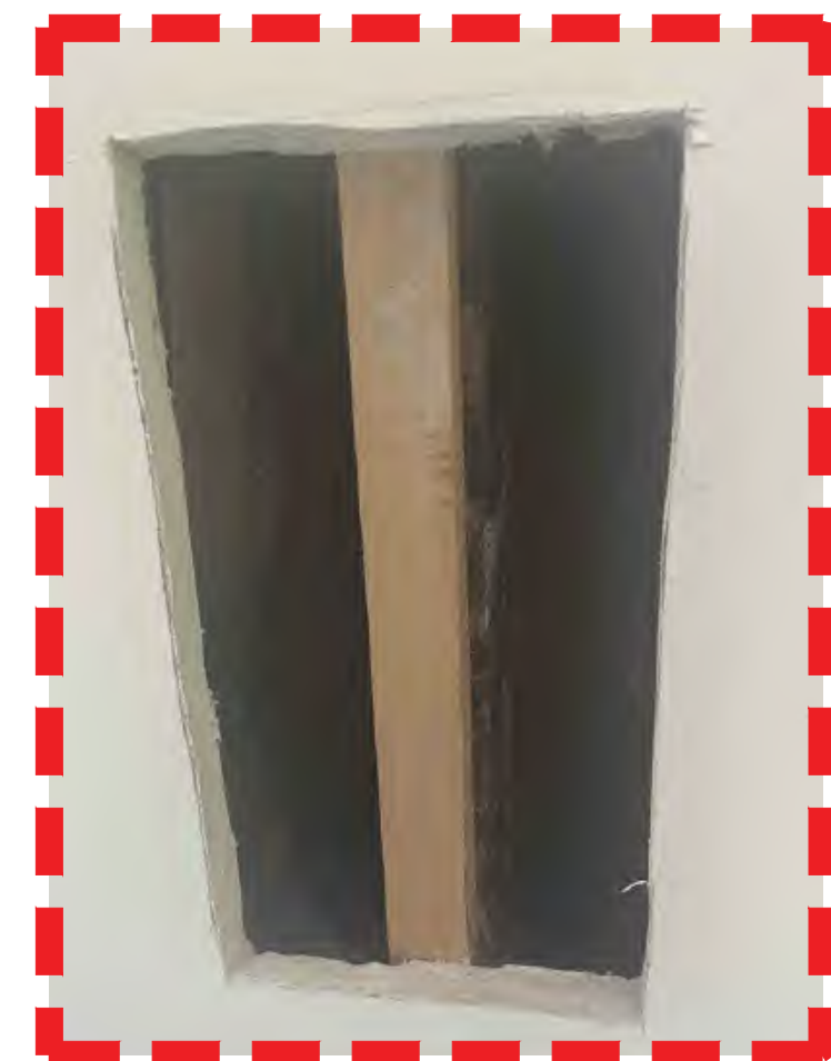
PHOTO OF PROBE OF REAR WALL AT FIRST FLOOR
