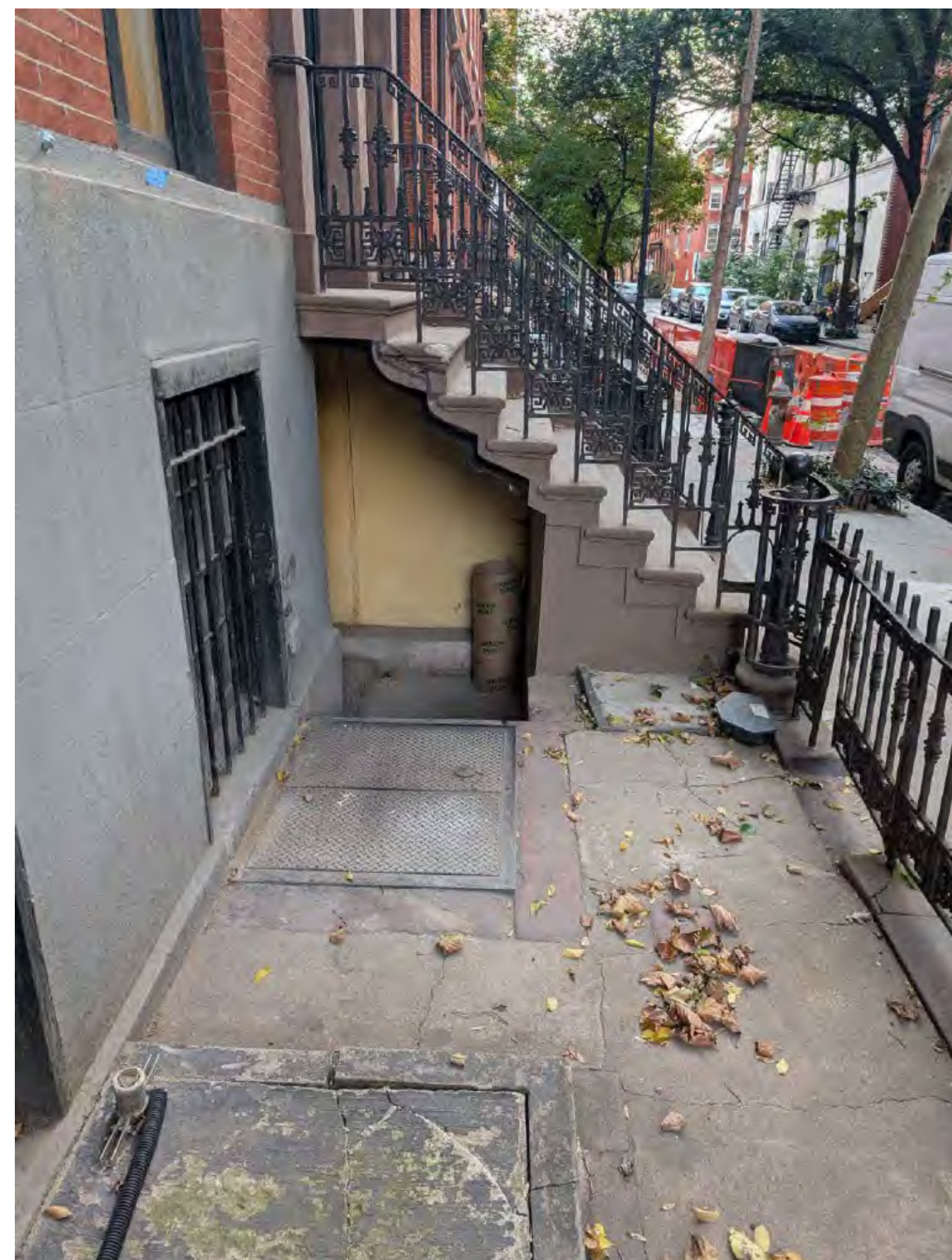
3 PHOTO OF EXISTING AREAWAY AT 81 JANE LOOKING EAST NOT TO SCALE
