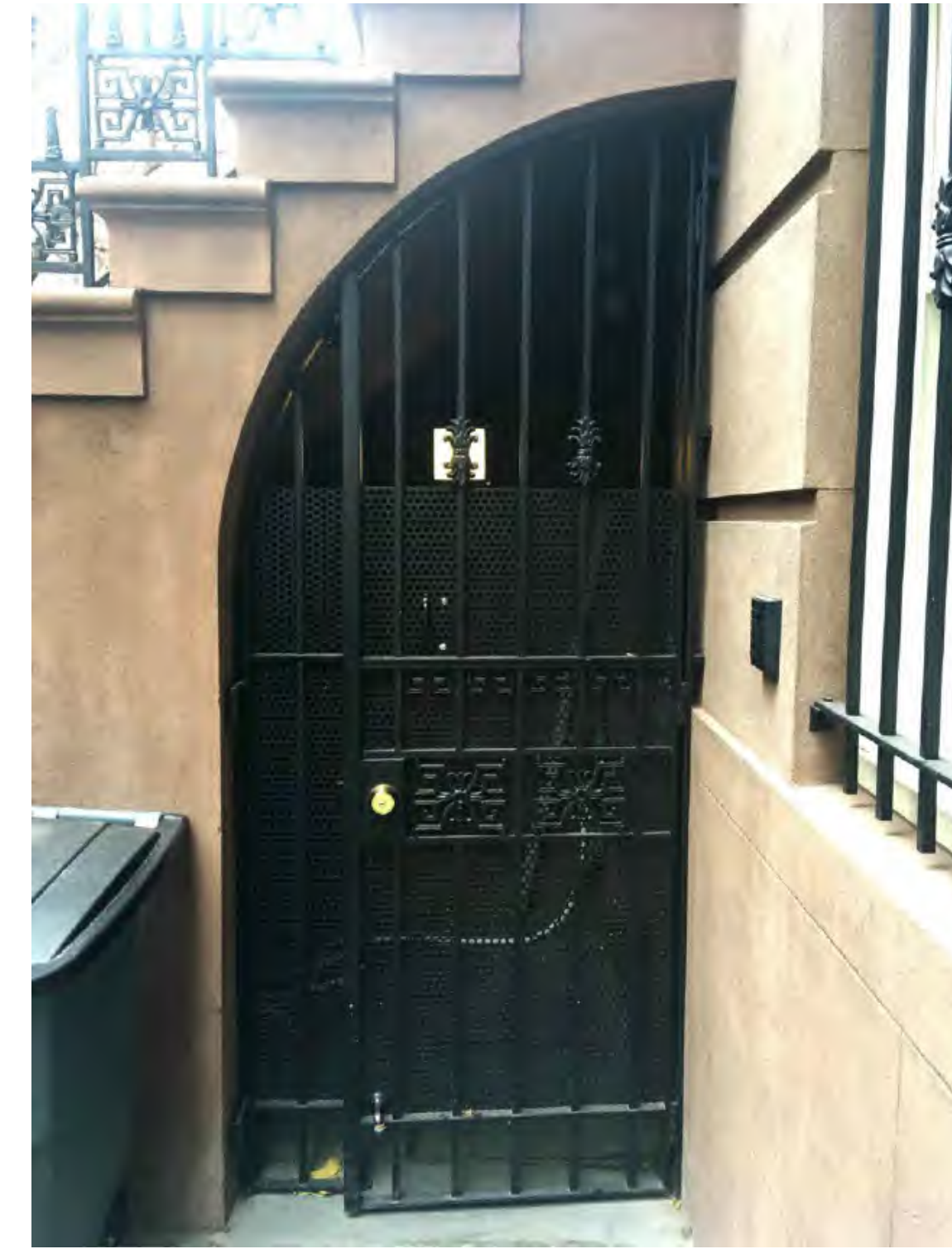
EXISTING AREAWAY DOOR & STOOP AT 75 JANE STREET
