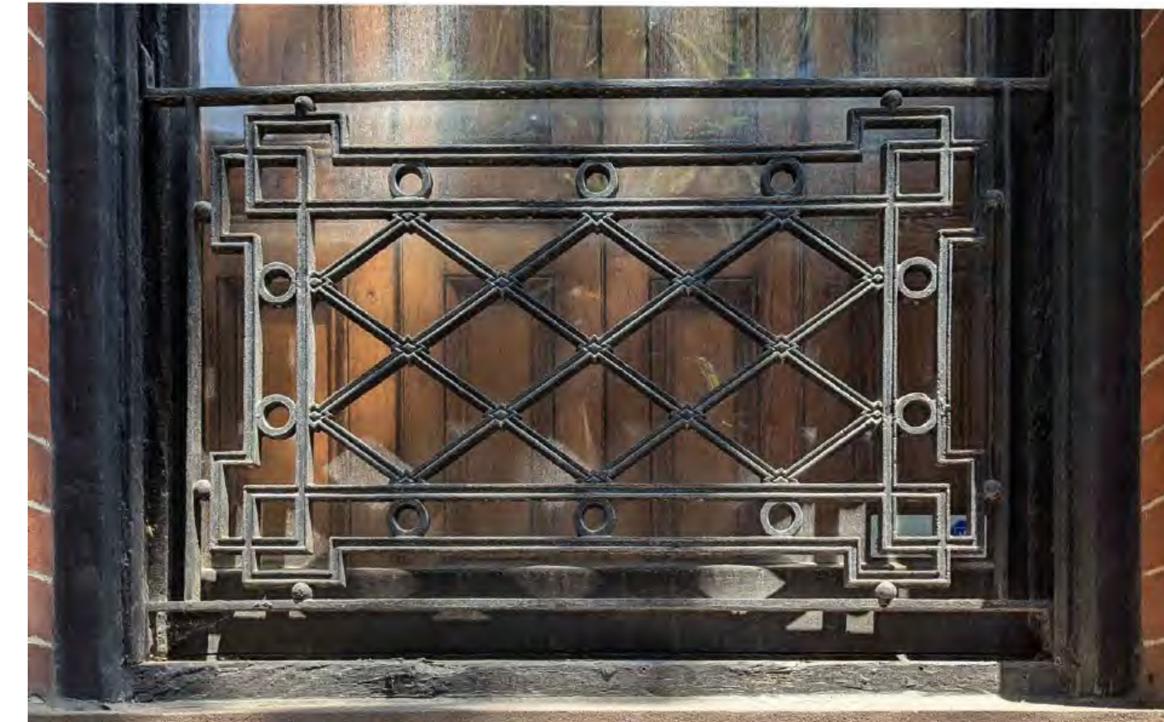
5 EXISTING WINDOW GRILLE AT FIRST FLOOR - 79 JANE SCALE: NTS
