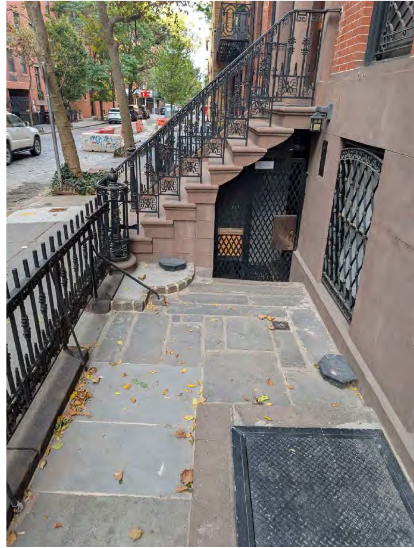
1 PHOTO OF EXISTING AREAWAY AT 79 JANE LOOKING WEST NOT TO SCALE
