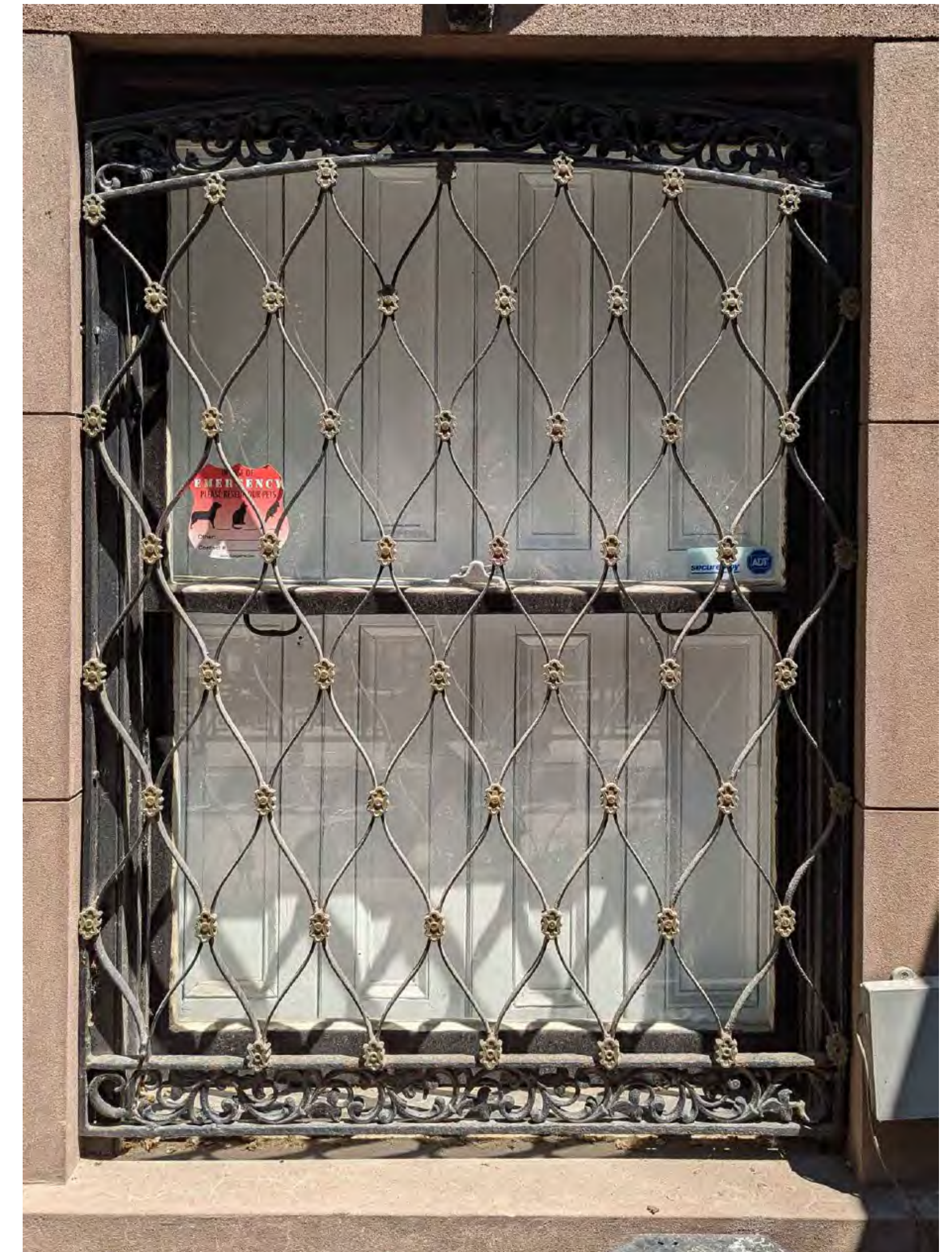
6 EXISTING WINDOW GRILLE AT BASEMENT - 79 JANE SCALE: NTS
