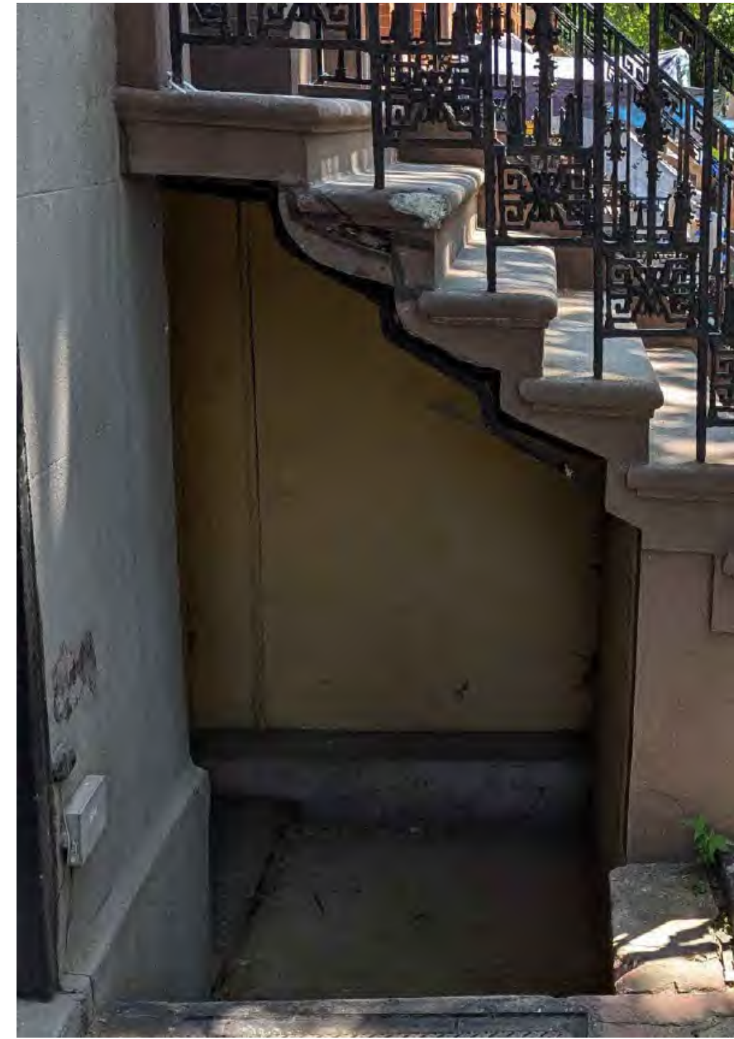
PHOTO OF EXISTING AREAWAY ENTRY & STOOP
