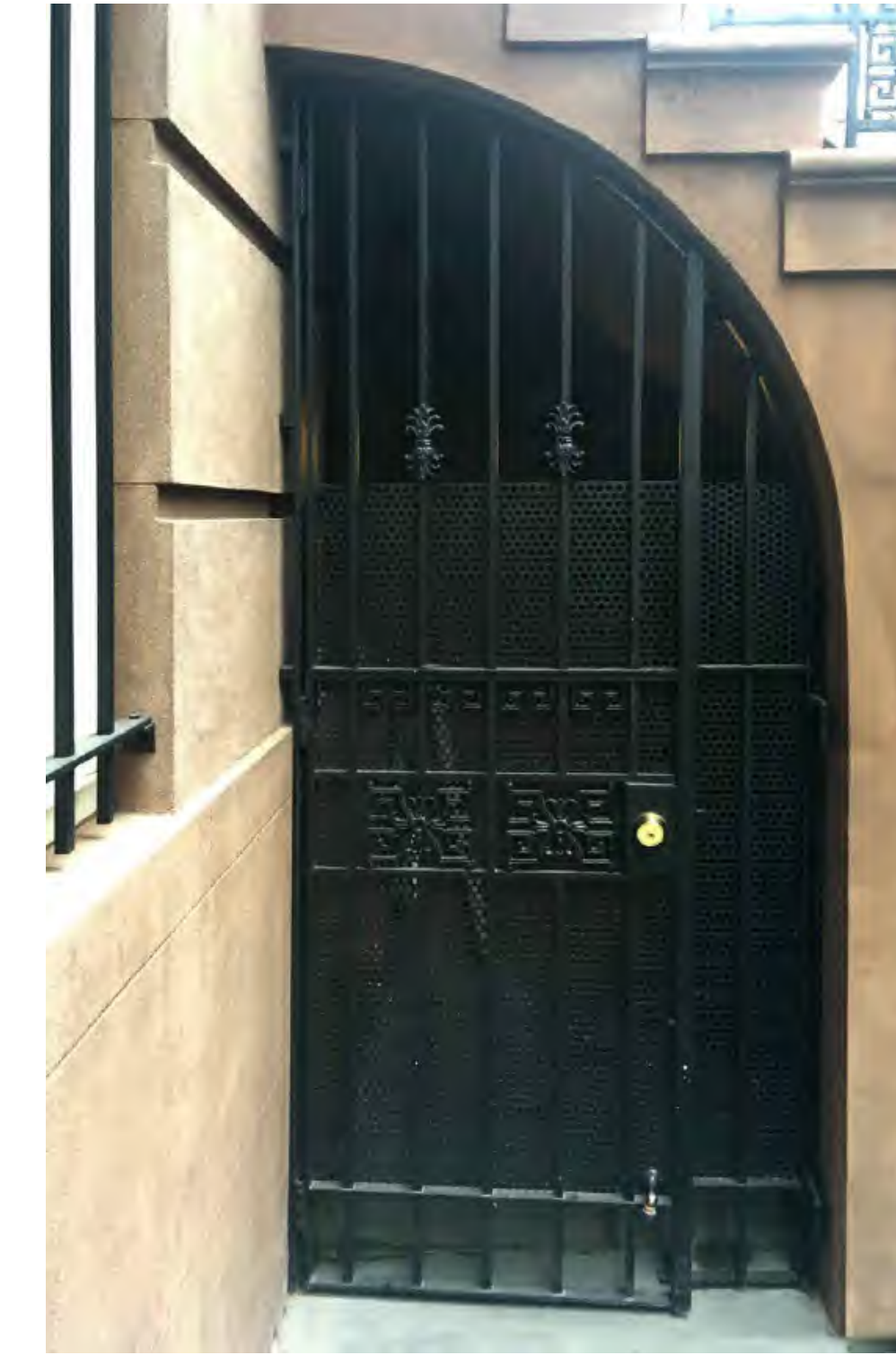
EXISTING AREAWAY DOOR & STOOP AT 77 JANE STREET
