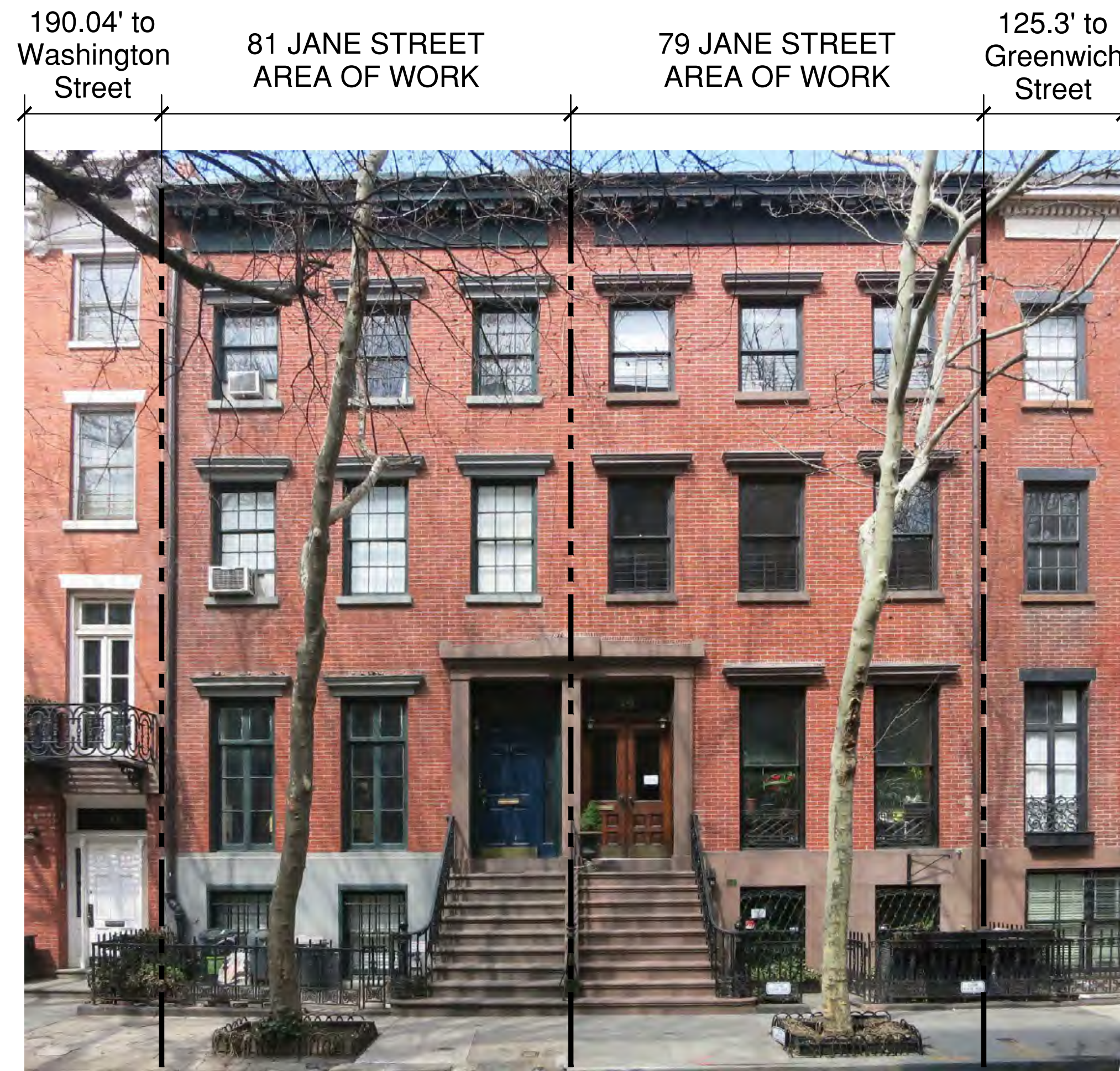
1 79-81 JANE STREET- EXISTING FRONT FACADE (SOUTH) - LOOKING NORTH NOT TO SCALE
