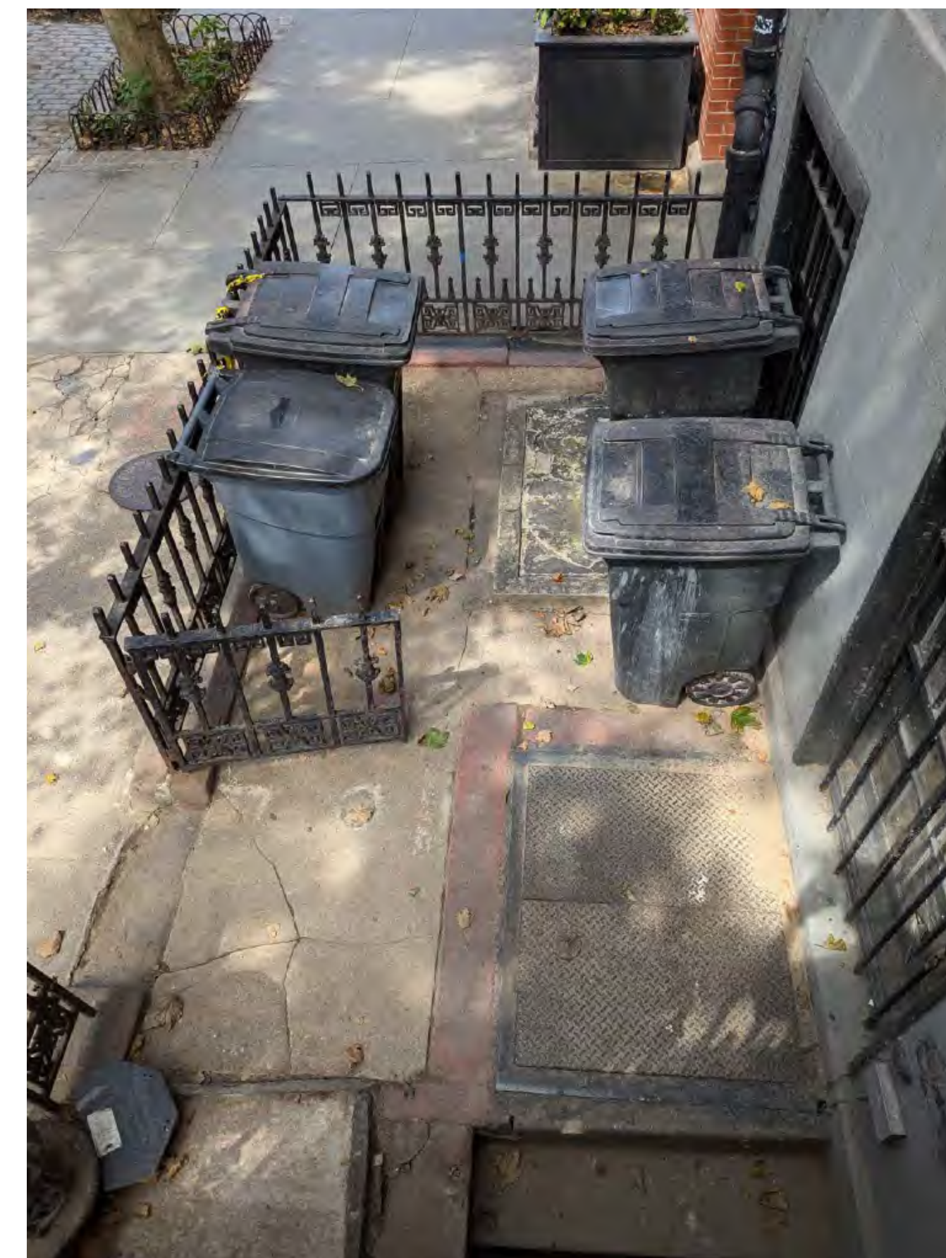
4 PHOTO OF EXISTING AREAWAY AT 81 JANE LOOKING WEST NOT TO SCALE
