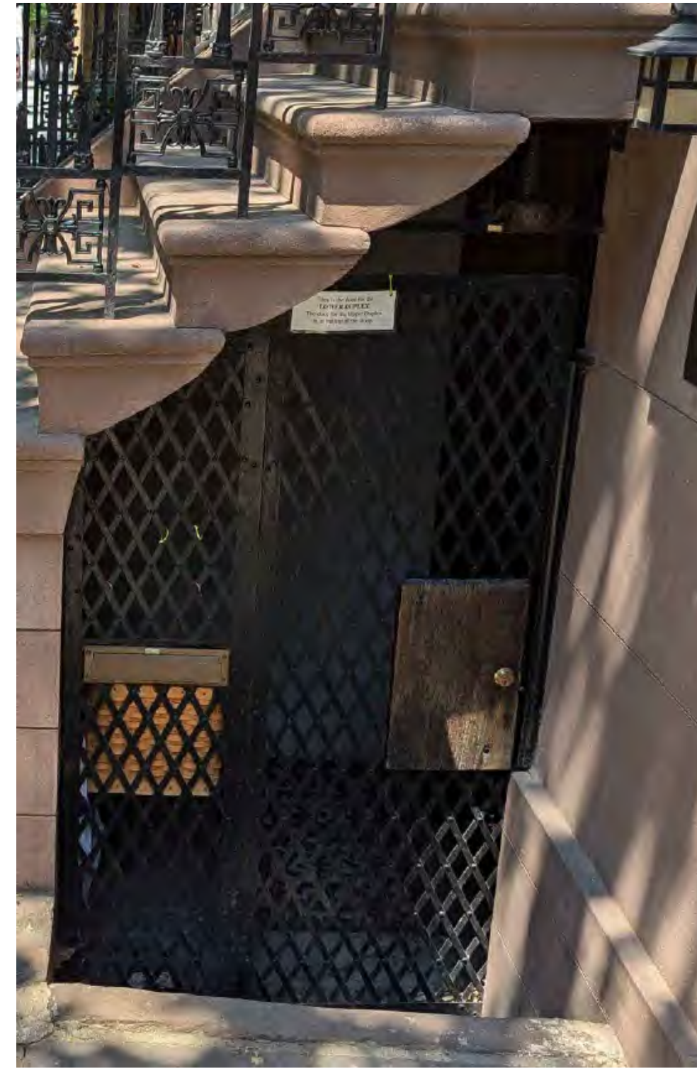
PHOTO OF EXISTING AREAWAY ENTRY & STOOP
