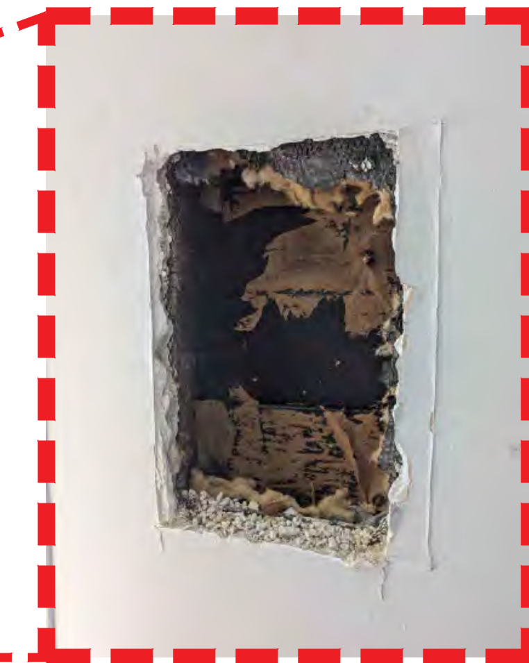
PHOTO OF PROBE OF REAR WALL AT SECOND FLOOR
