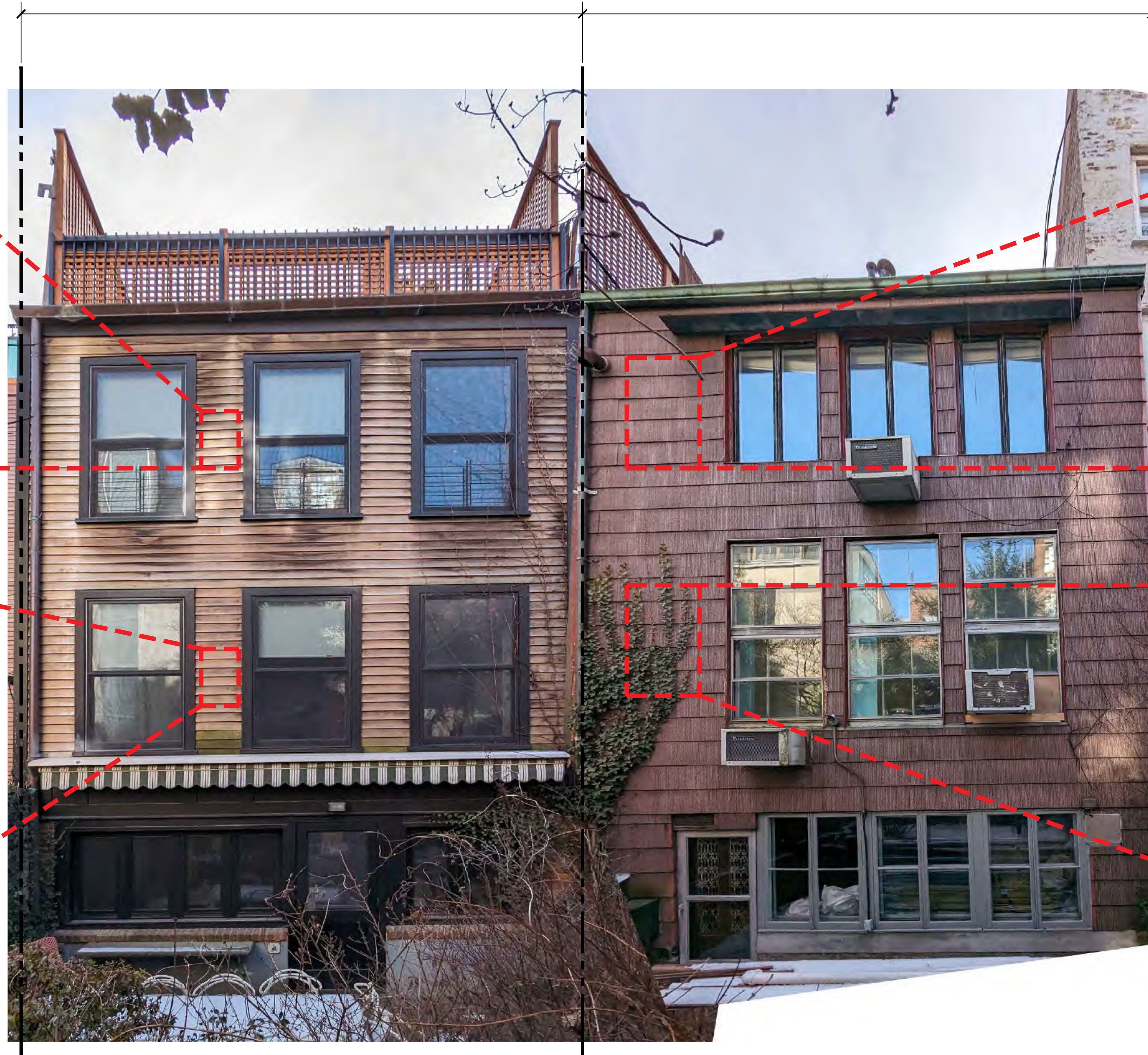
1 PHOTO OF EXISTING REAR FACADE 79 - 81 JANE SCALE: NTS
