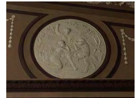
Balcony detail on ceiling rib
