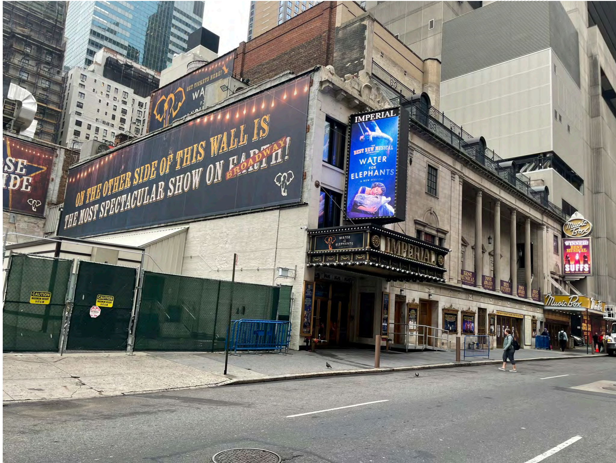
View of 45th Street Lobby Building & Temporary Toilet Trailer
