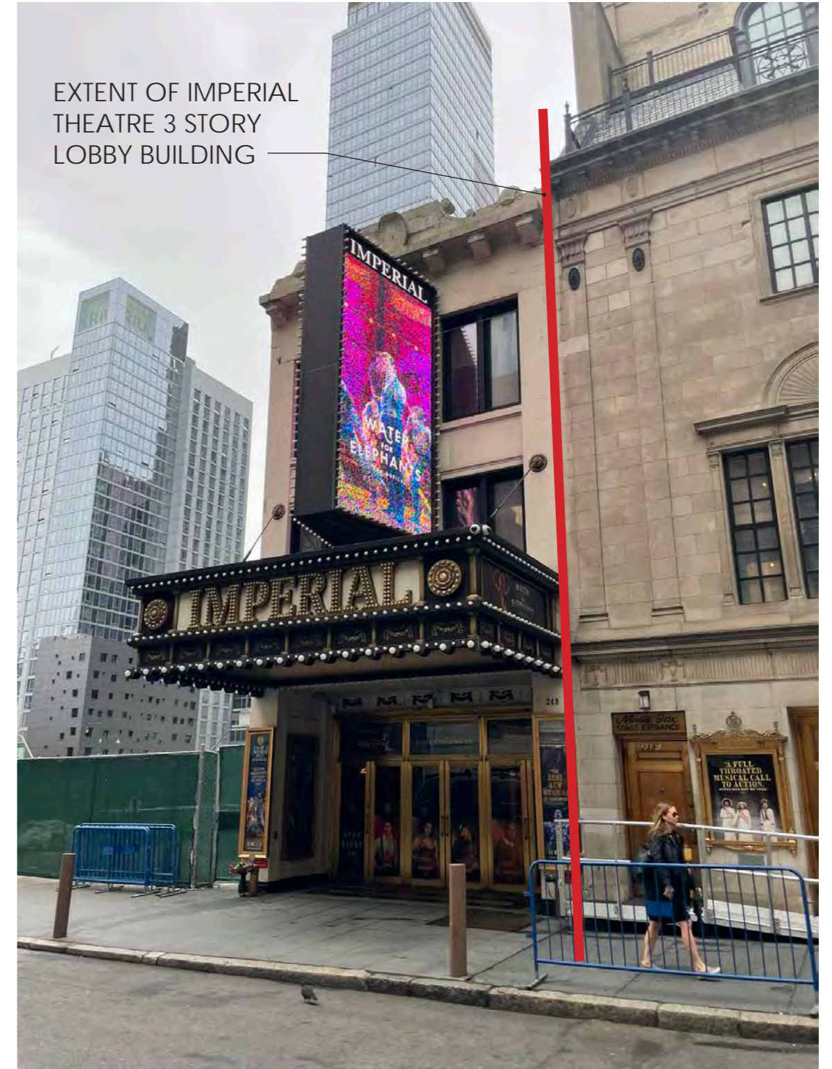
View of 45th Street Lobby Building & Temporary Toilet Trailer
