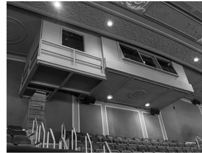
Existing Tech Booth
