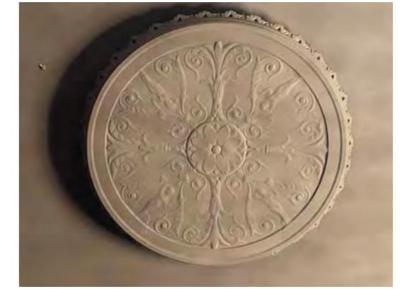
Mechanical duct cover (non-original)
