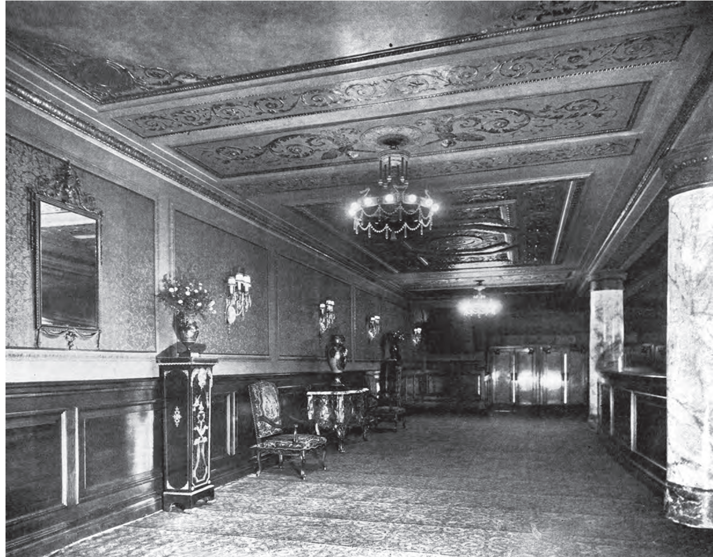
Historic photo of Rear Orchestra Promenade looking towards House Left Sound & Light Lock
