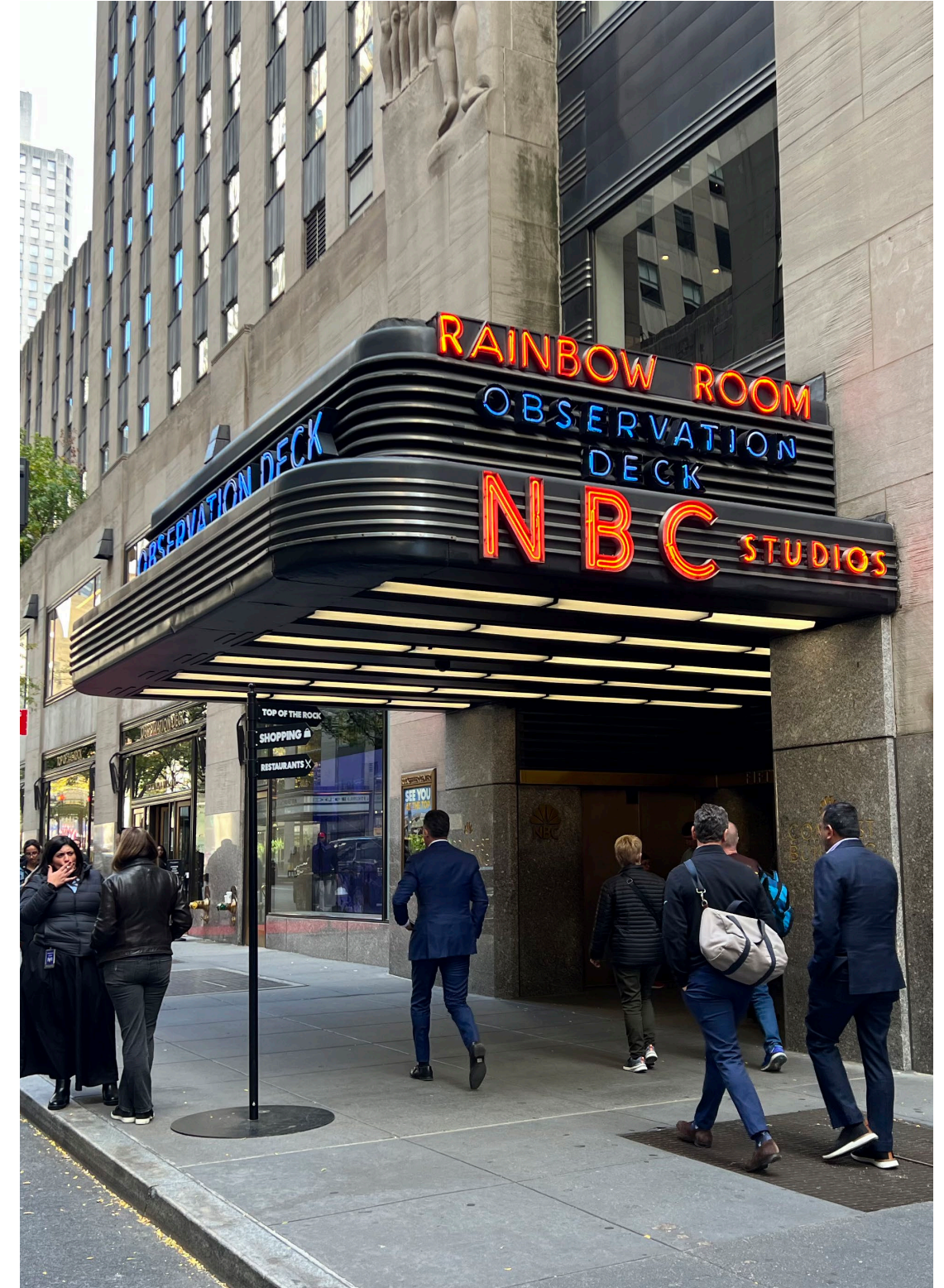
WEST 50TH STREET MARQUEE, EXISTING CONDITIONS
