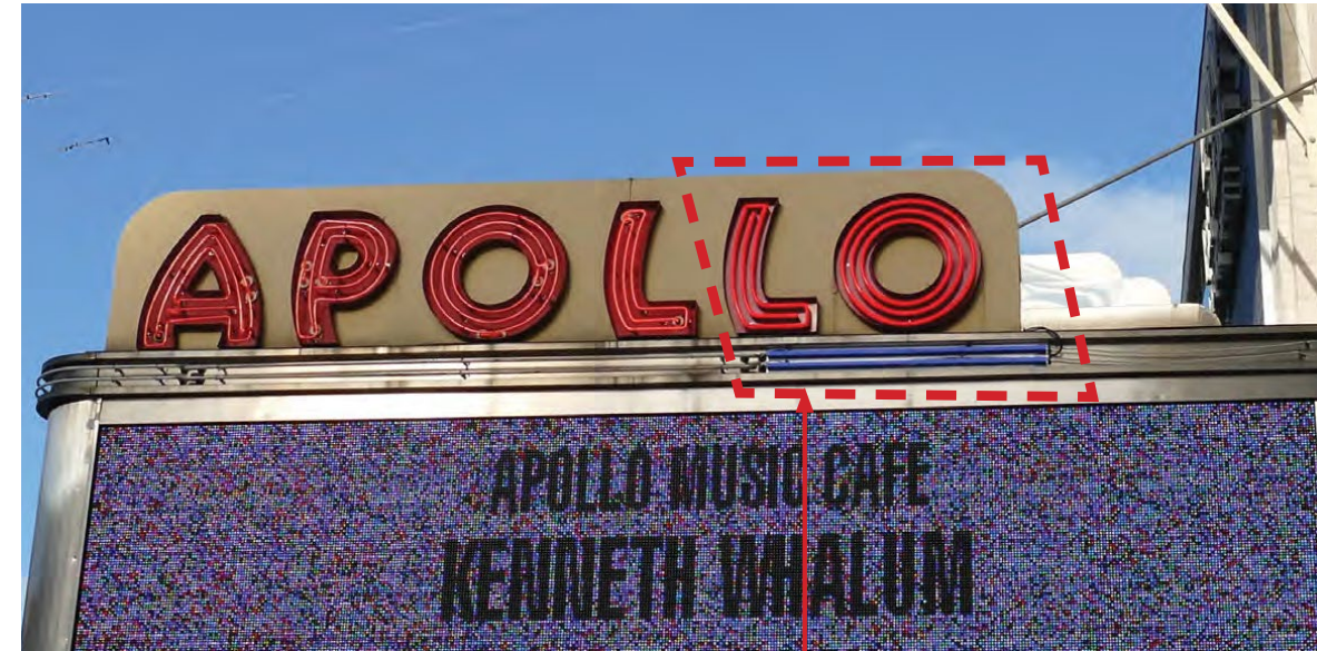
MOCK-UP OF LED NEON LETTERS & BLUE LED NEON STRIPES SHOWN AT DAYTIME
