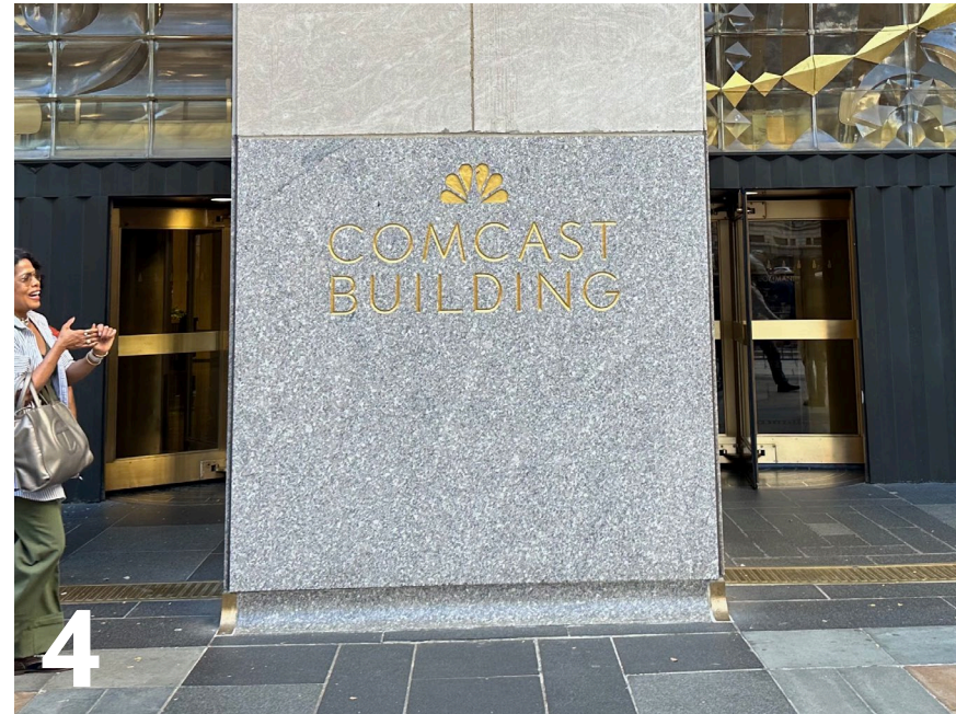
4 PLAZA ENTRANCE, DETAIL OF EXISTING CARVED CORNERSTONE
