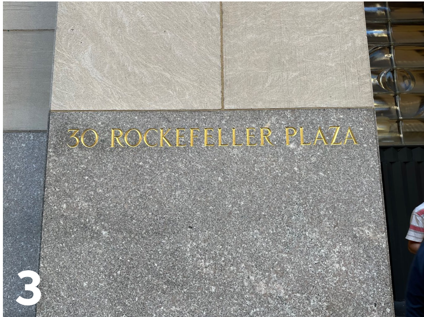
3 PLAZA ENTRANCE, DETAIL OF EXISTING ADDRESSING
