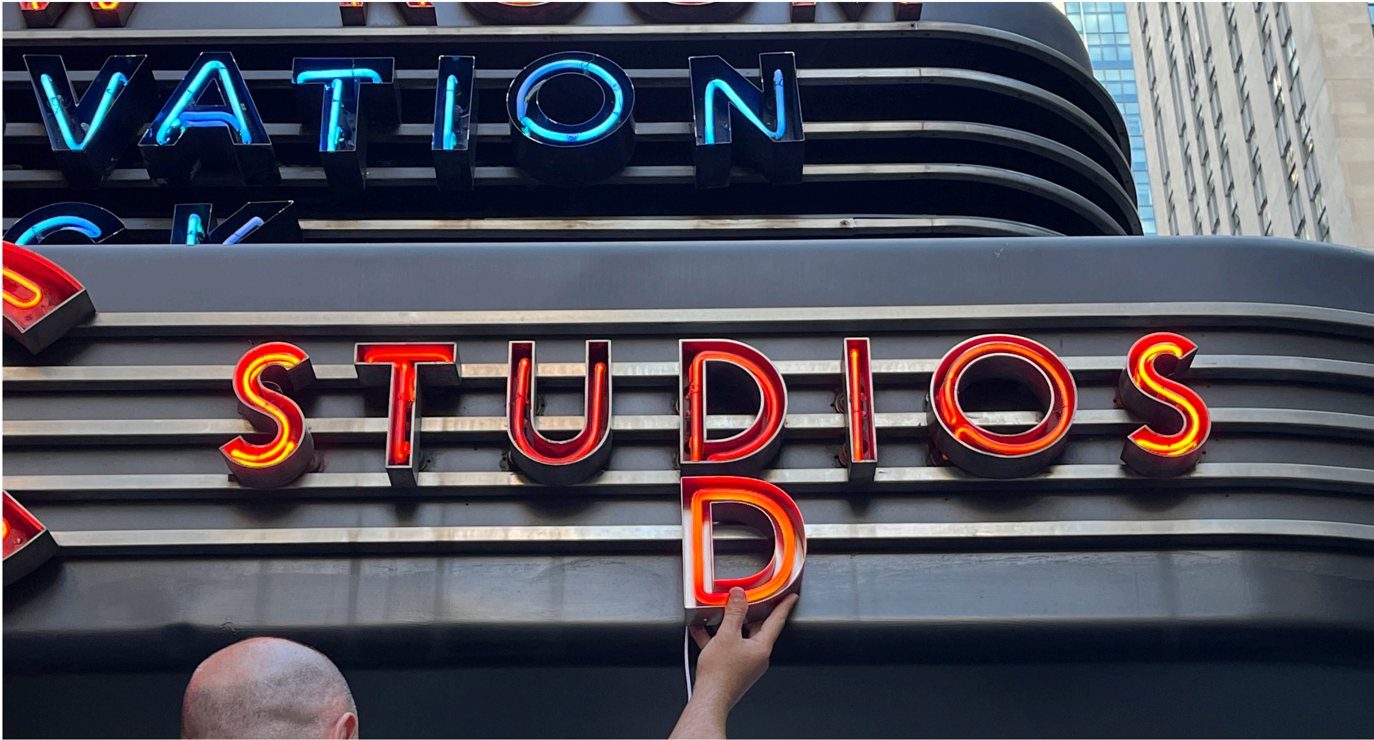
DETAIL OF THE SINGLE-TUBE LED LETTERING MOCK-UP
