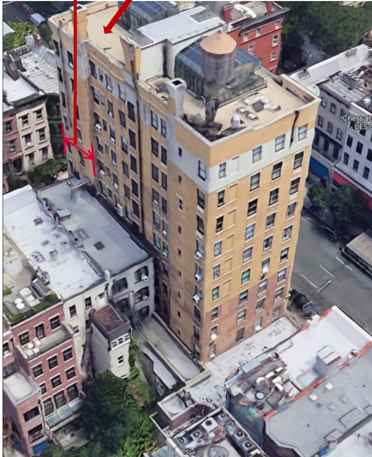
Aerial view showing no accessible yard area at 1312 Madison Ave.
