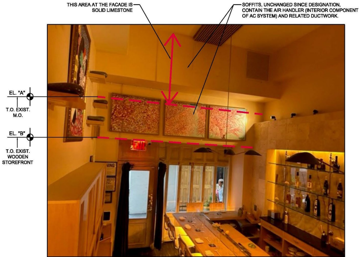
View looking towards storefront. Fully finished interior to remain.
