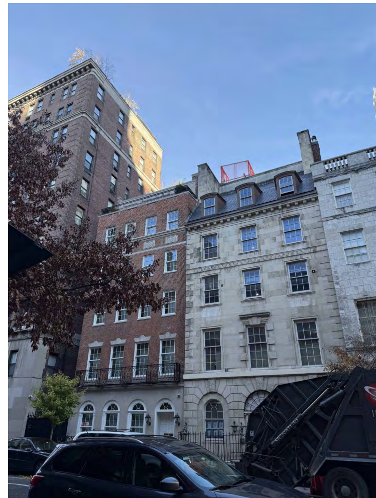
VIEW B: FROM OPPOSITE SIDE OF 70TH STREET
