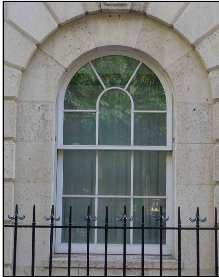
± 6'-11 1/2" NEW WINDOW IN EXISTING MASONRY OPENING
