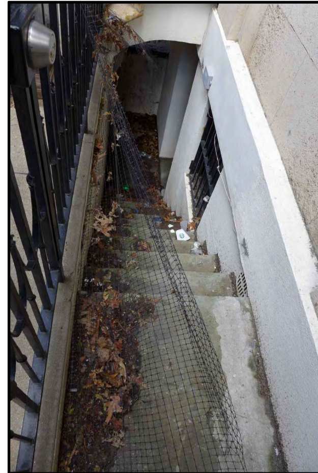
EXISTING 43 EAST 70TH STREET AREAWAY LOOKING WEST
