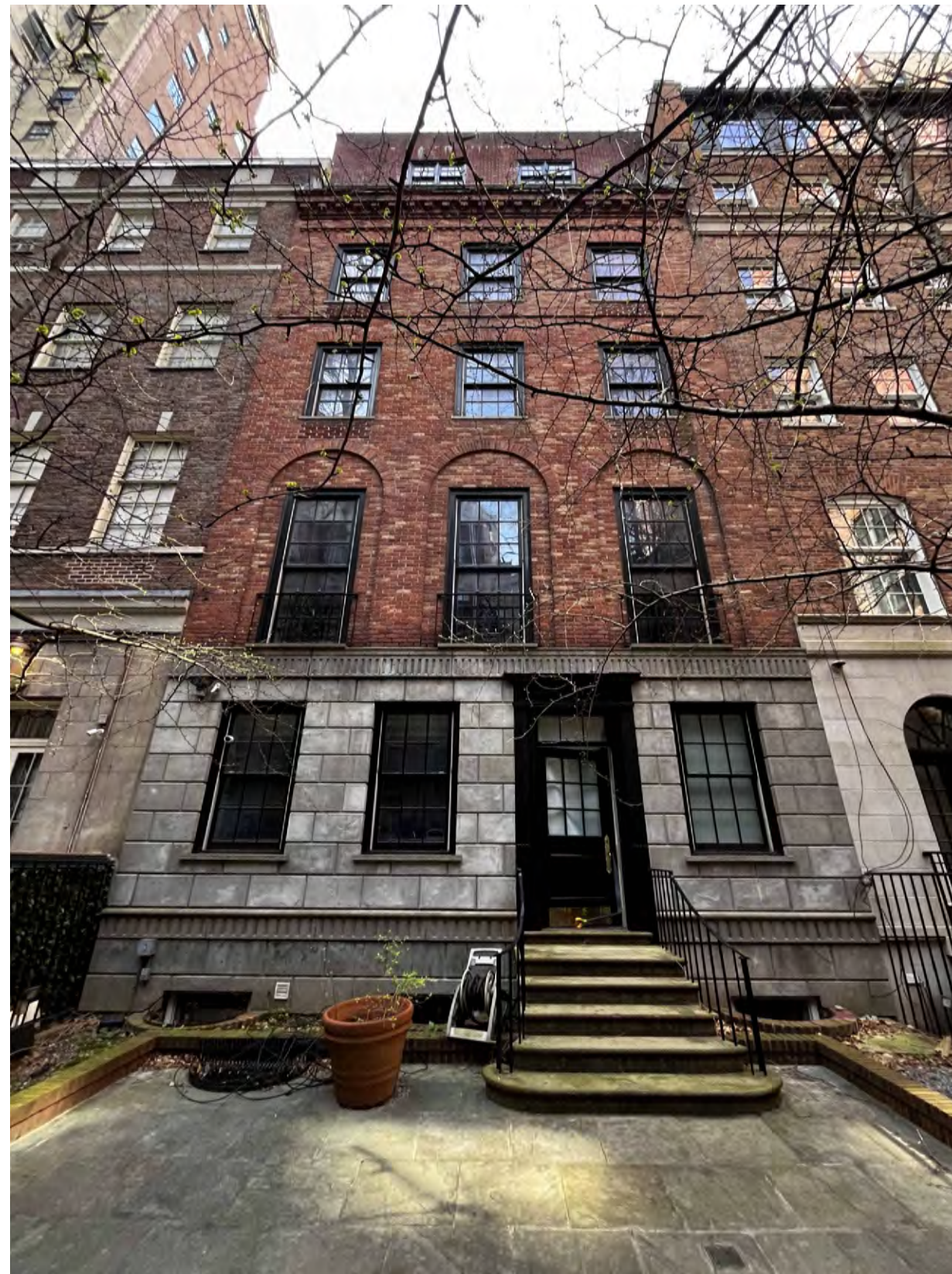
43 EAST 70TH STREET: EXISTING CONDITIONS NORTH FACADE
