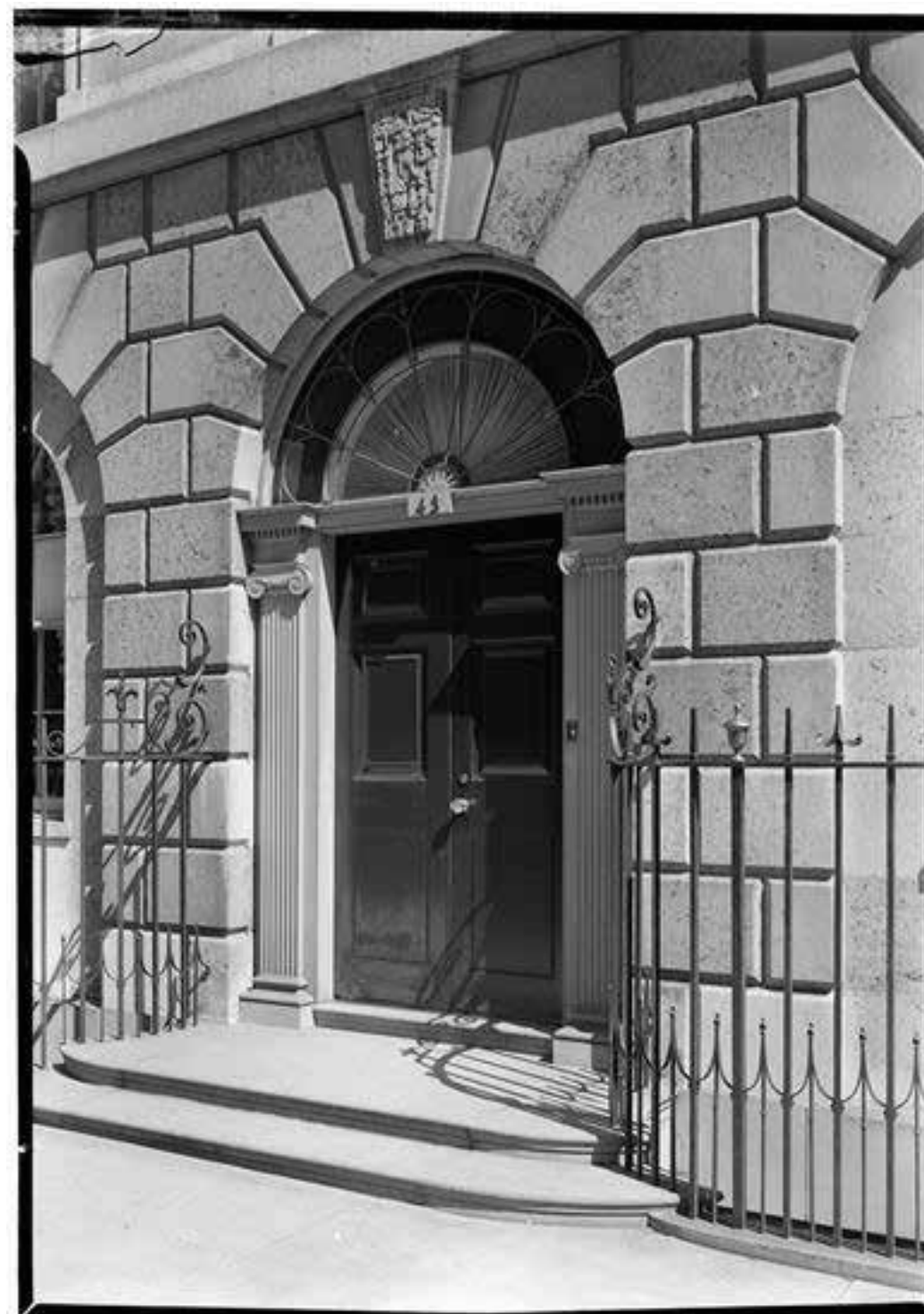
43 EAST 70TH STREET: ENTRY DOOR, 1938 (MUSEUM OF THE CITY OF NEW YORK ARCHIVES)
