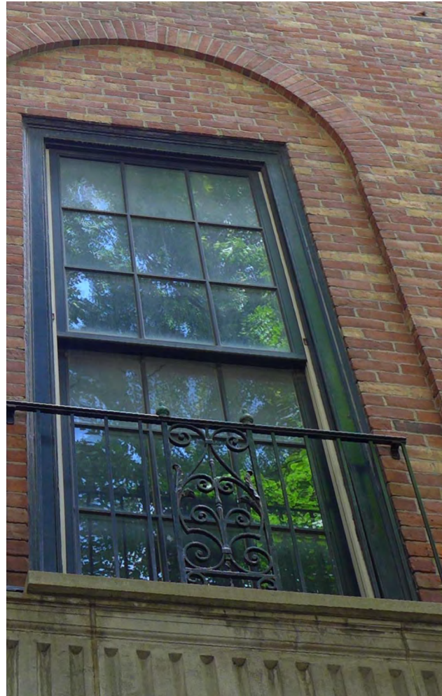
± 9'-4 1/4" NEW WINDOW IN EXISTING MASONRY OPENING
