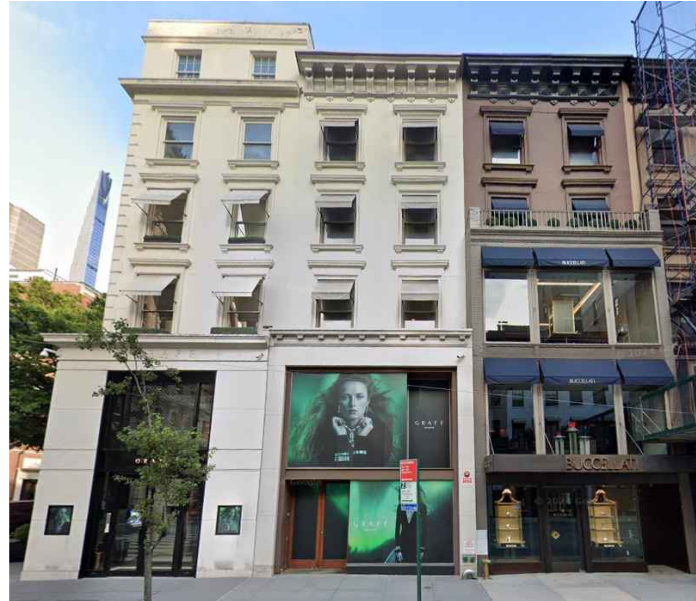
CONDITION @ 710-714 MADISON AVE. 3 NTS
