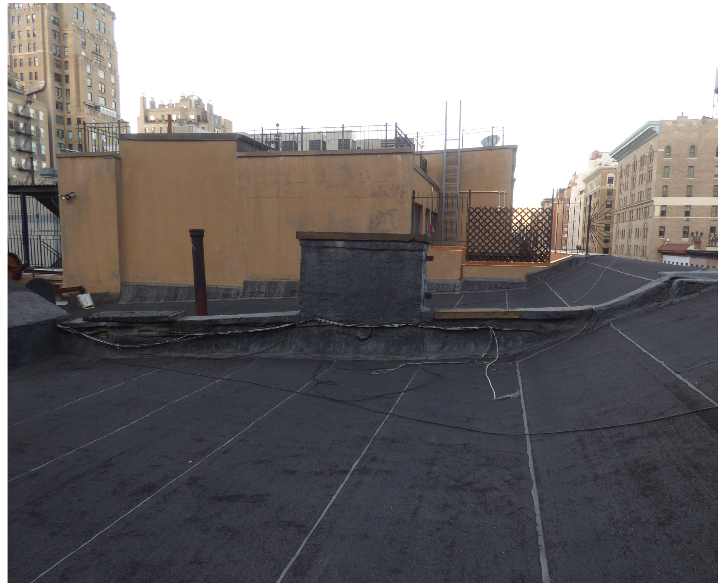
View of the roof looking north.
