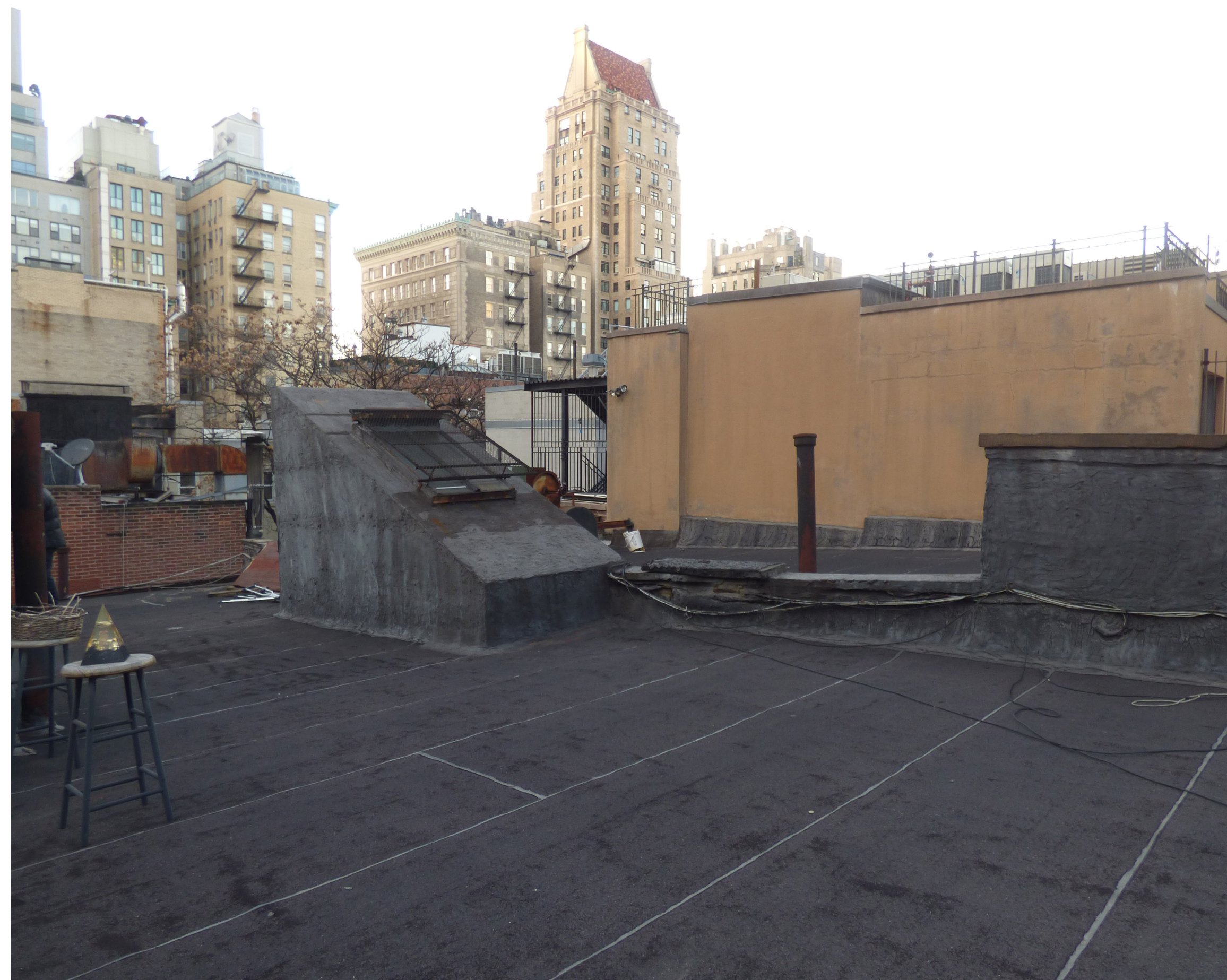
View of the roof looking northwest towards 696 Madison roof.
