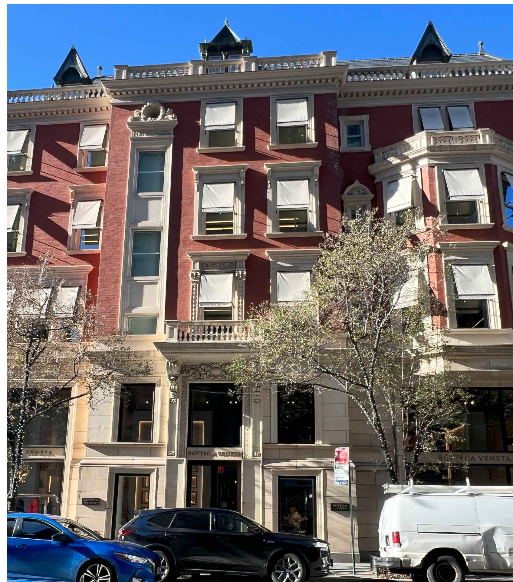
CONDITION @ 740 MADISON AVE. 3 NTS
