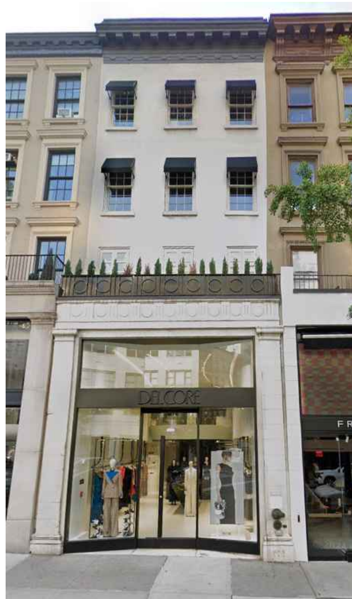
CONDITION @ 789 MADISON AVE. 3 NTS
