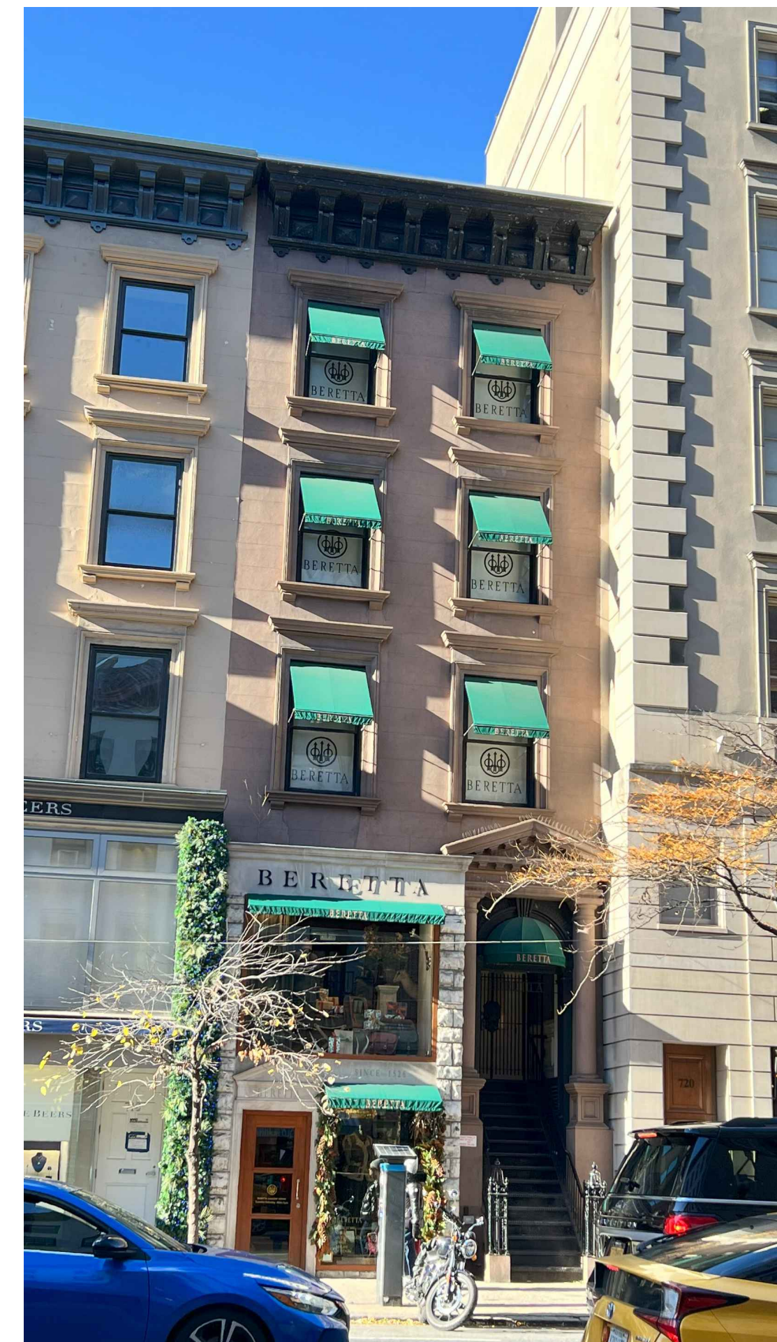
CONDITION @ 718 MADISON AVE. 1 NTS
