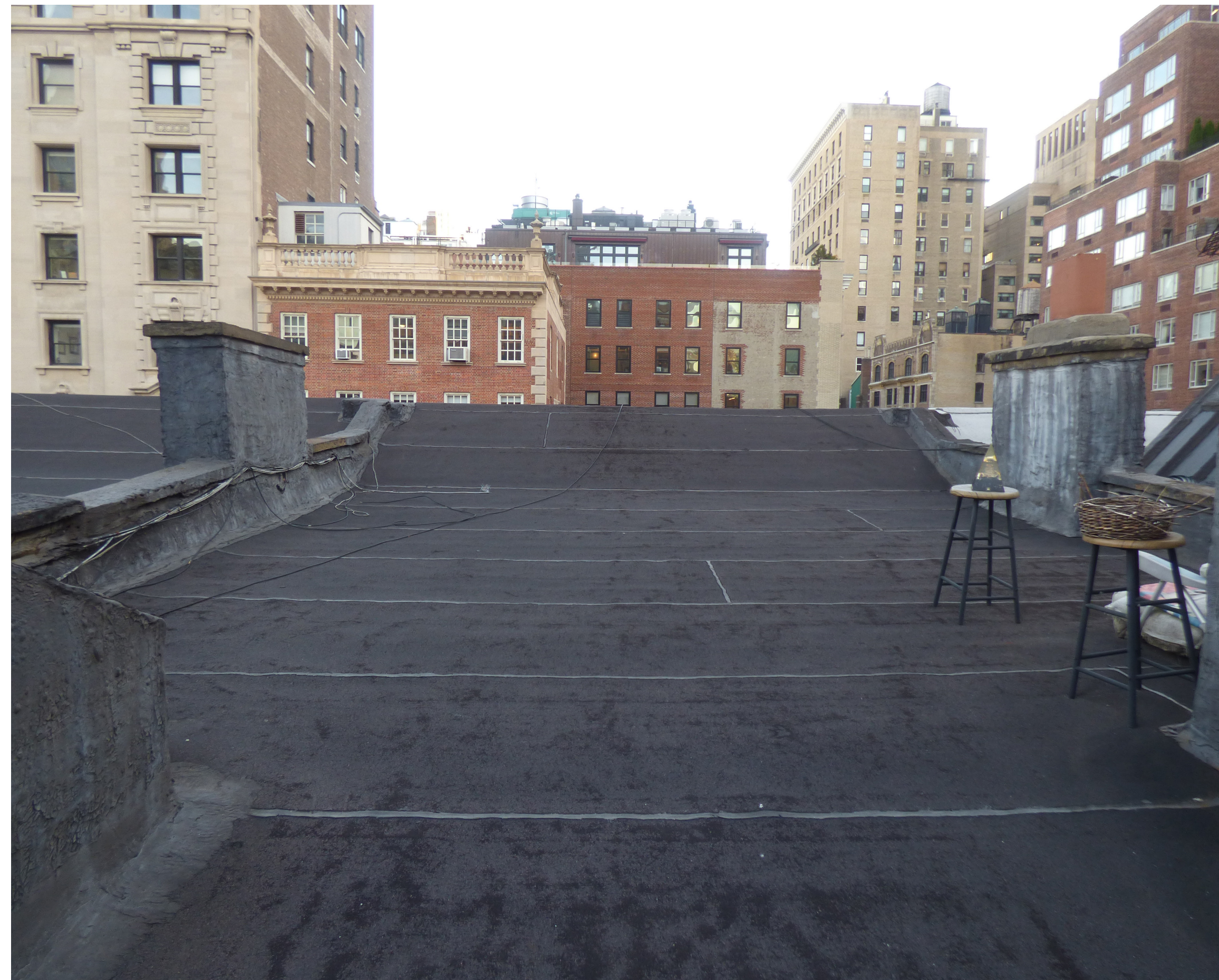
View of the roof looking east.
