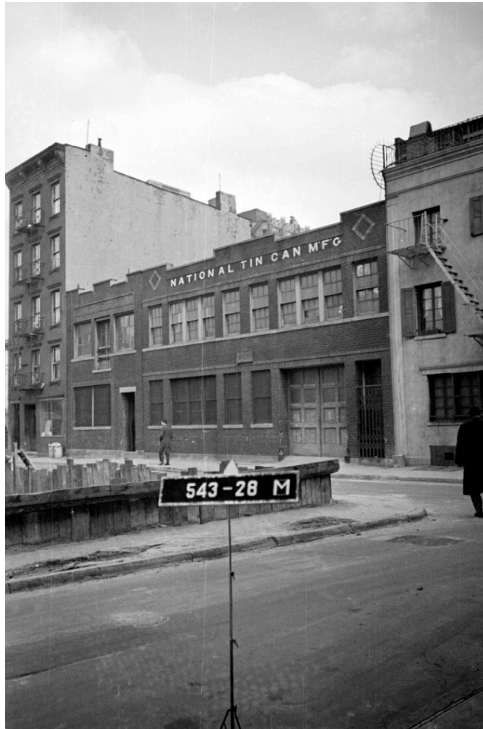
18 Minetta Lane Factory, 1919-23
