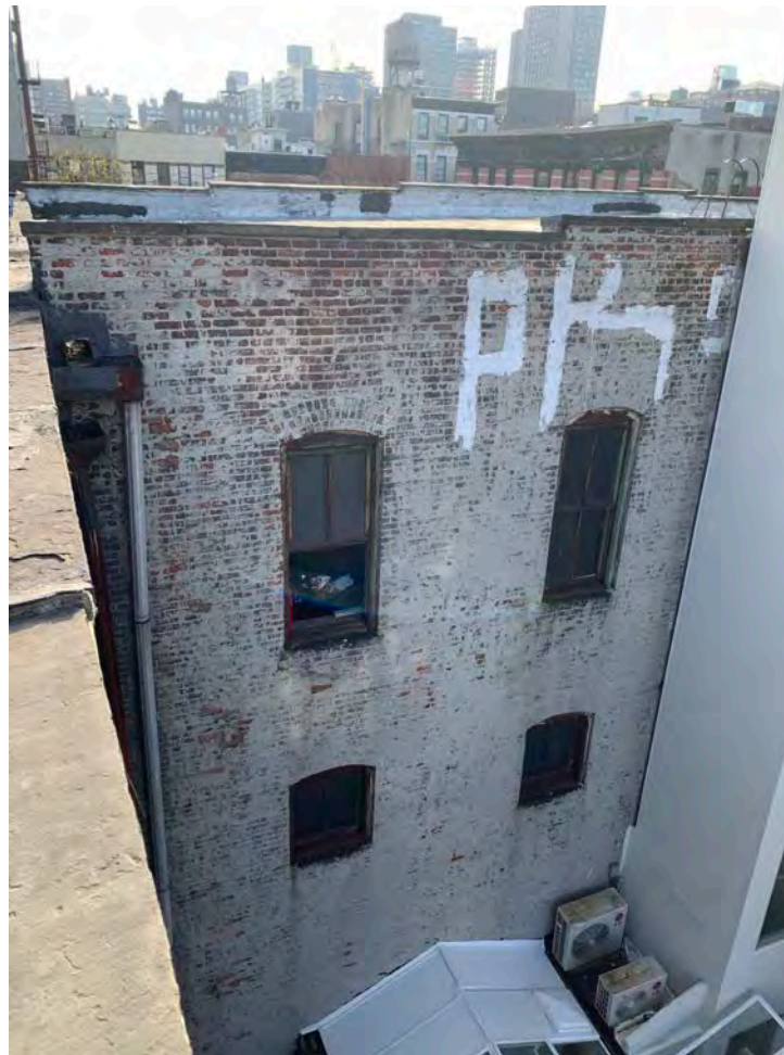
1. Rear Facade looking South-East
