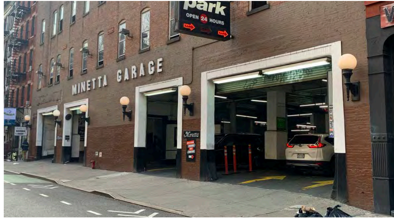
Detail View of Building Base Including Garage Entrances and Cast-Iron Globe Bracket Lamps
