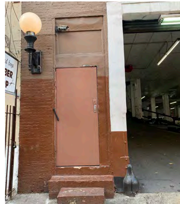
Entry Door, Stairs and Cast-Iron Globe Bracket Lamp
