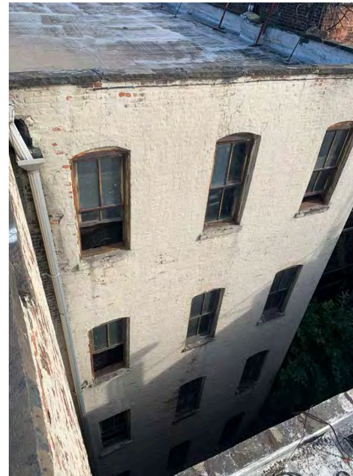
3. Rear Facade looking North-East
