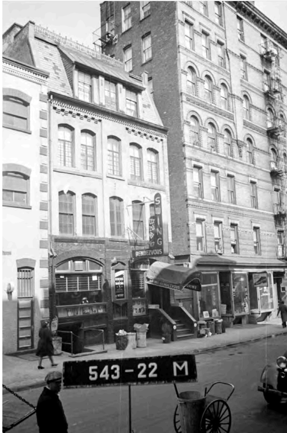
117 MacDougal St Stable, c. 1864
