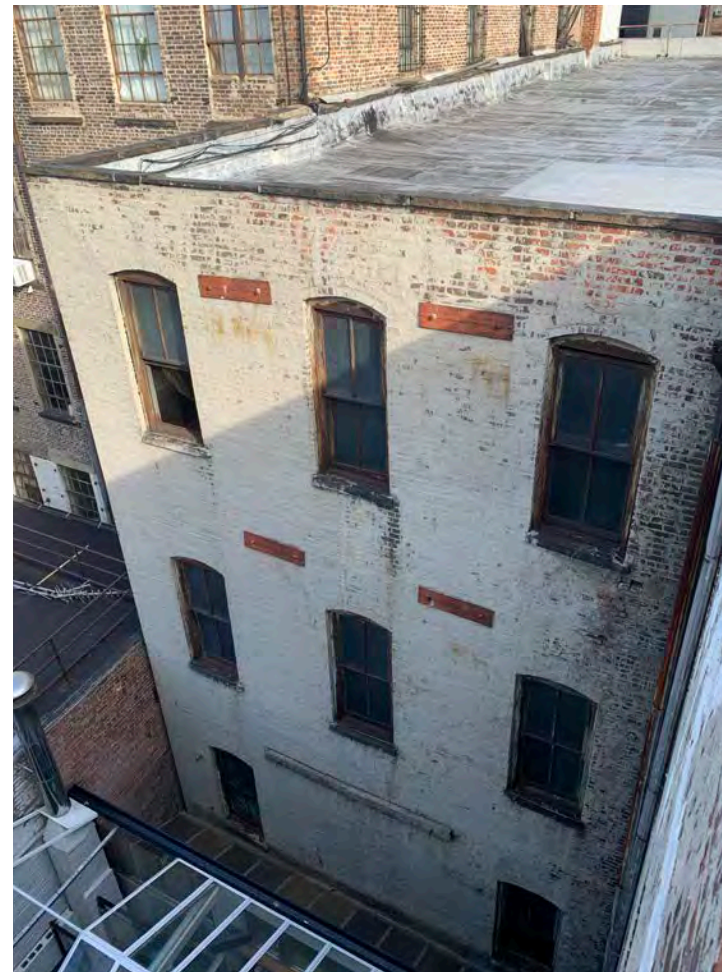
2. Rear Facade looking North-West
