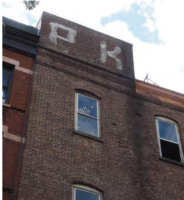
Northeastern Bulkhead, Windows, and Corbelled Cornice
