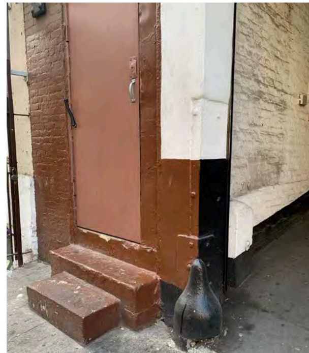
Garage Entry Bumpers, Stairs and Entry Door
