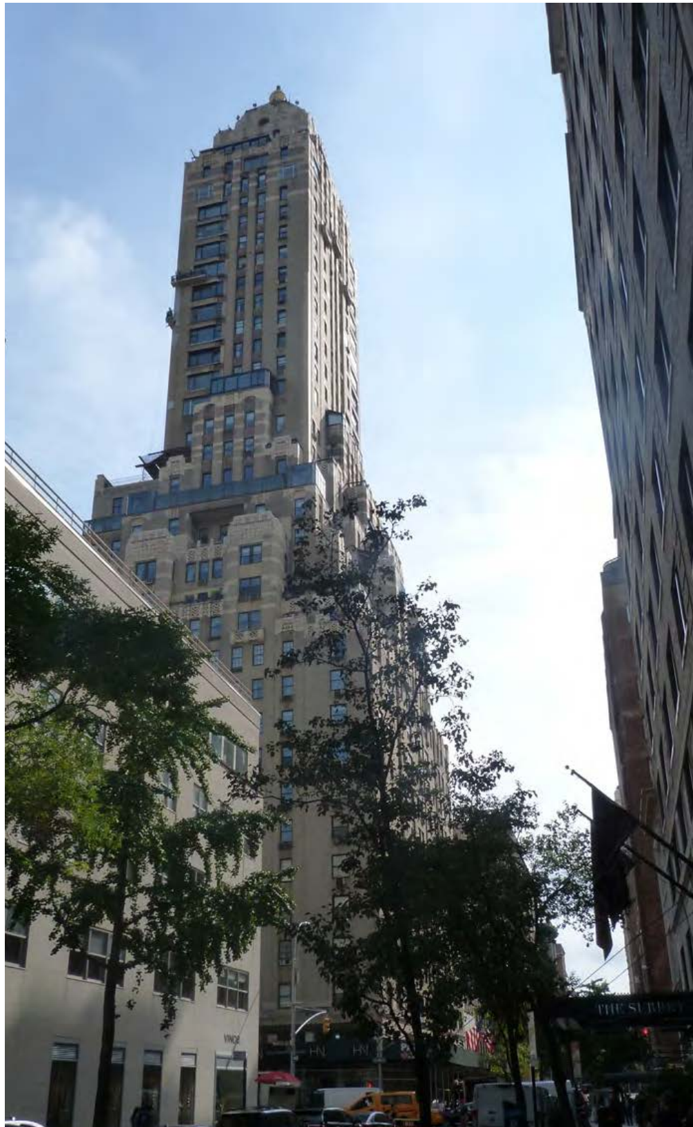
THE CARLYLE HOTEL: 1998 LPC APPROVED GREENHOUSE IMAGE CREDIT: LEE LEDBETTER & ASSOC. ARCHITECTURE
