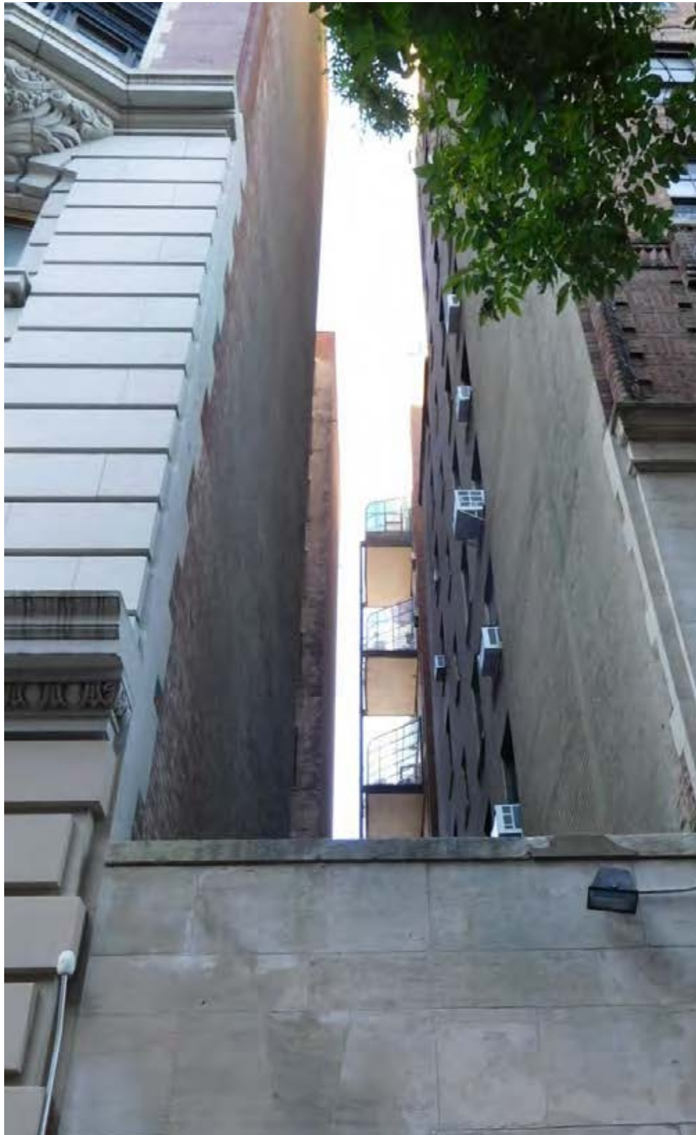
330 WEST END AVE: 2021 EXISTING ENCLOSED BALCONIES
