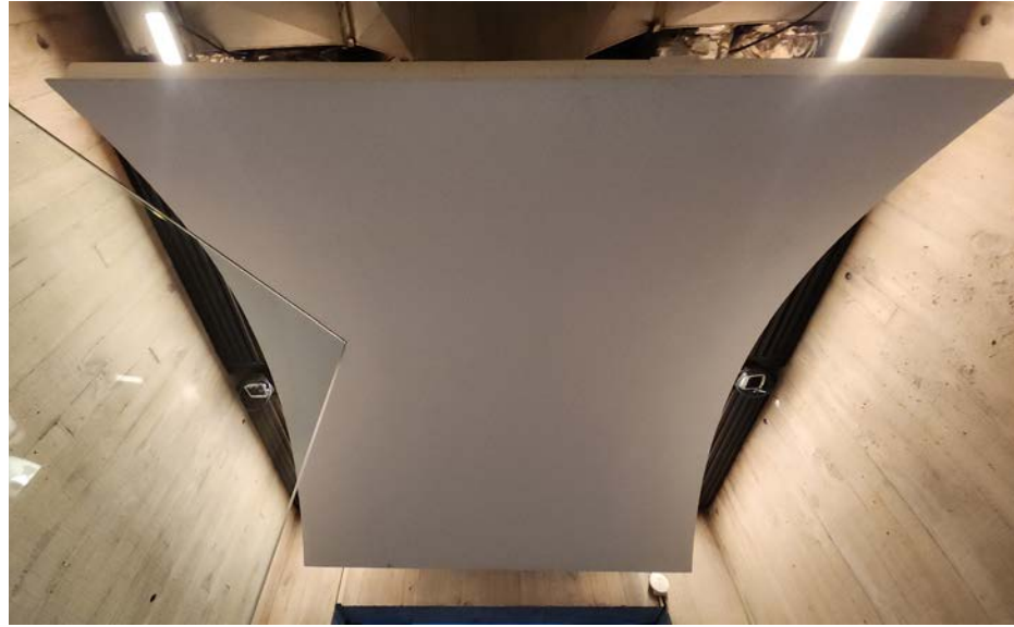
EXISTING VESTIBULE ENTRY: FLOATING WHITE PANEL
