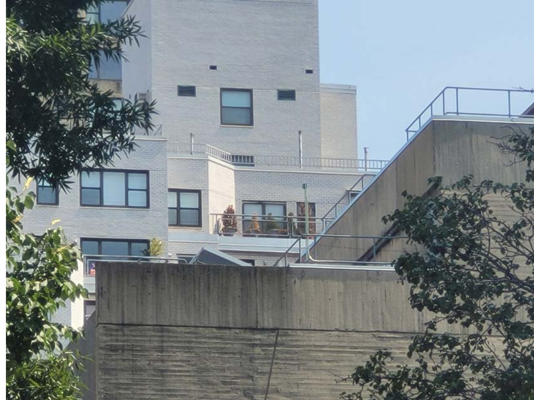
South party wall termination (facing north) Photograph by: PBDW Architects
