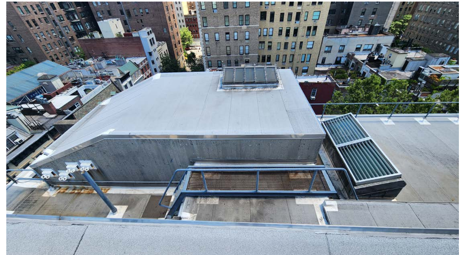
3: Stair bulkhead (facing east) Photograph by: Herzog & DeMeuron
