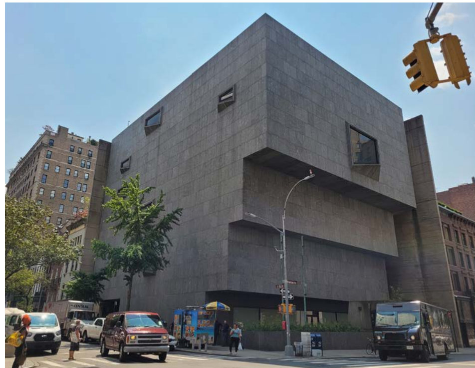
View from Madison Ave and 75th St. (facing southeast) Photograph by: PBDW Architects
