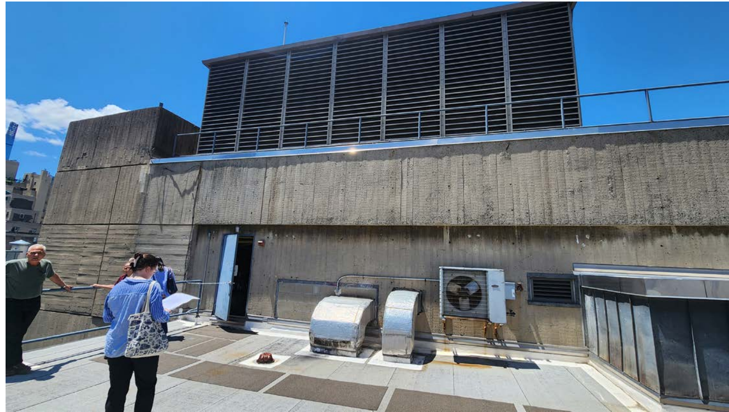
1: Mechanical bulkhead elevation (facing west) Photograph by: Herzog & DeMeuron
