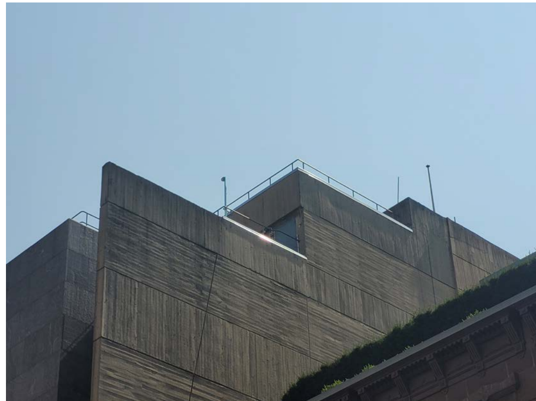
South party wall enlarged (facing north) Photograph by: PBDW Architects
