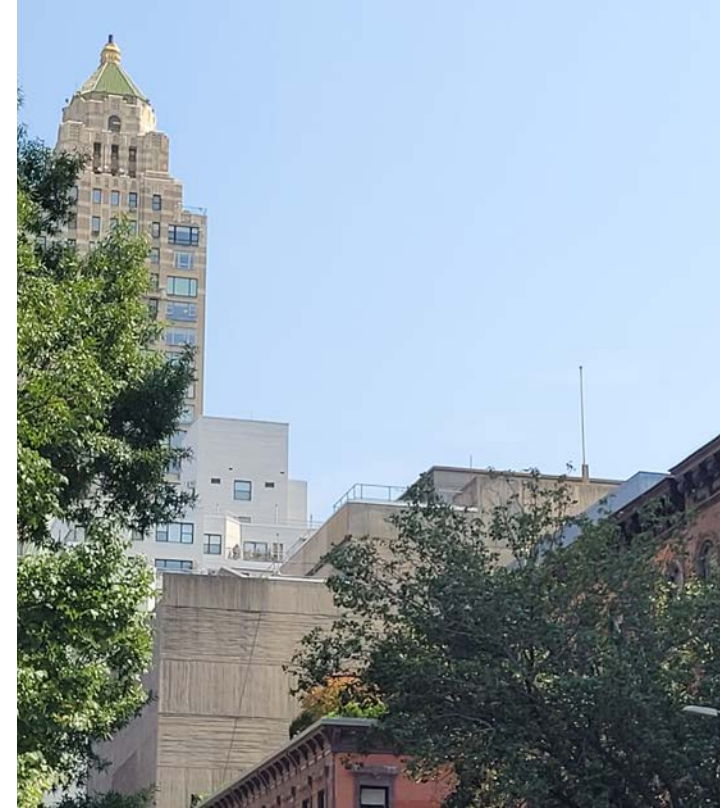
South party wall (facing north) Photograph by: PBDW Architects
