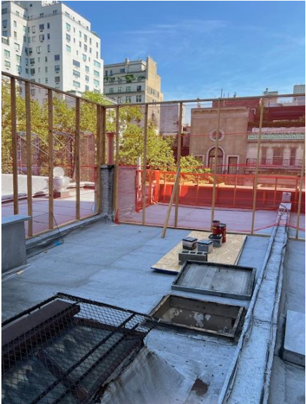
Rooftop with mockups, looking north.
