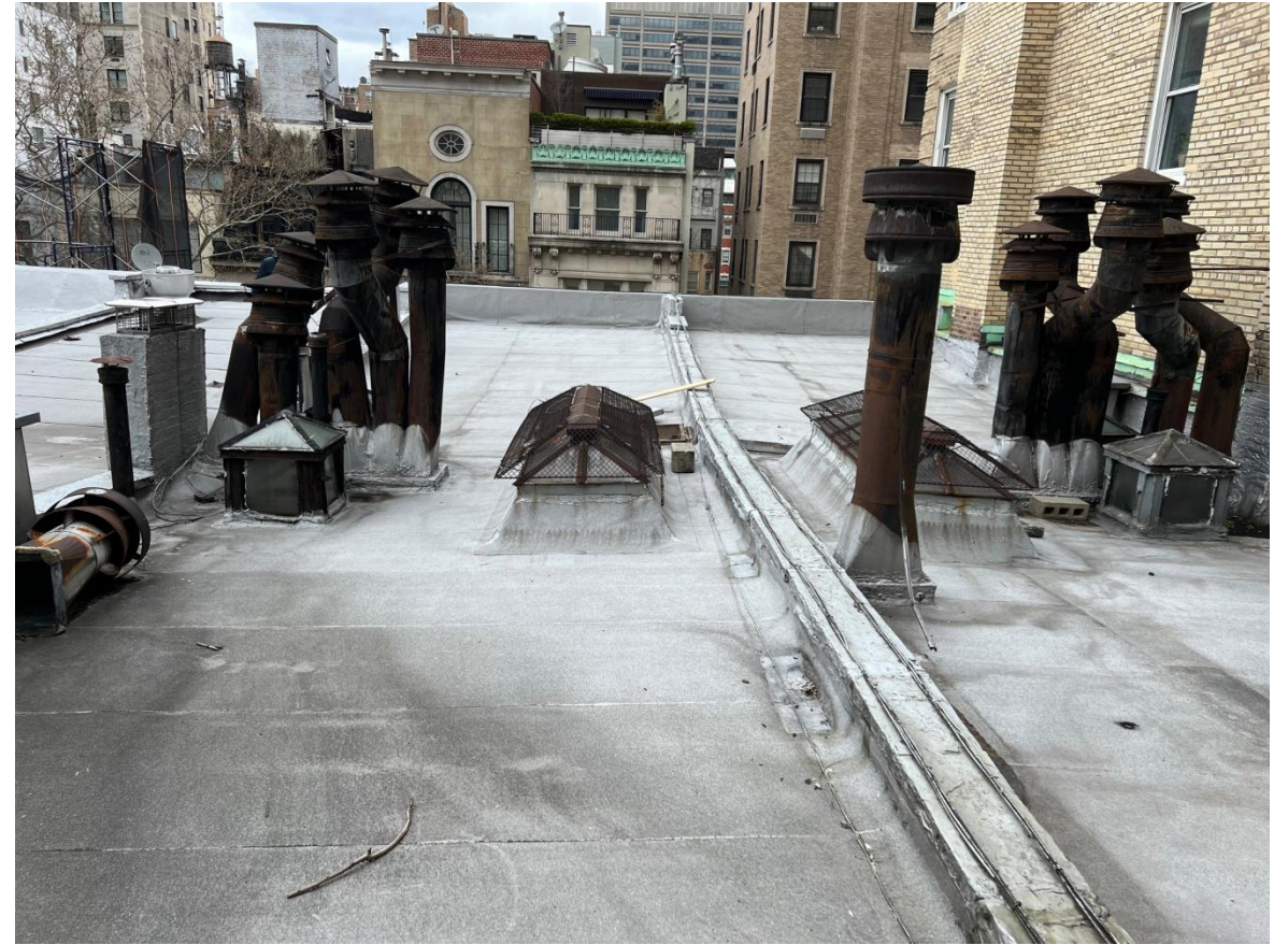
Existing roof, looking north.
