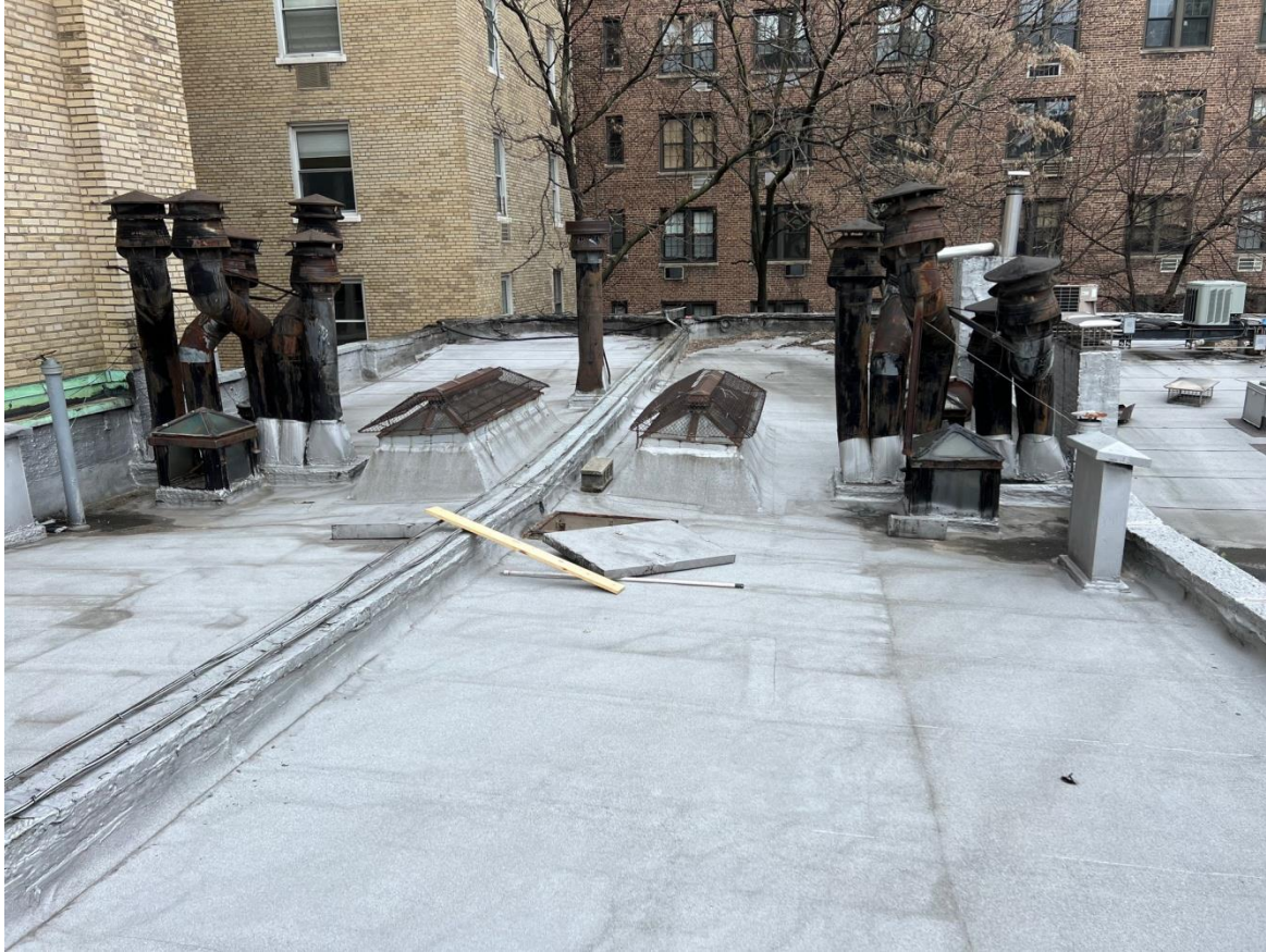
Existing roof, looking south.
