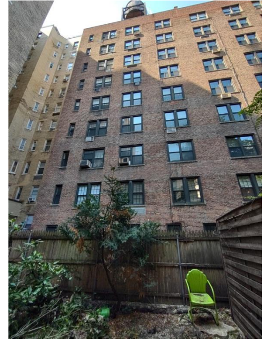
Rear yards looking south.
