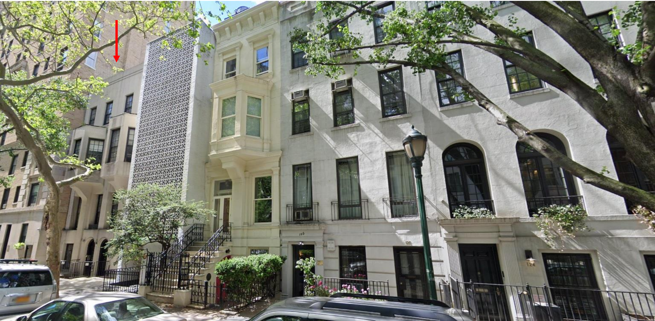
Streetscape looking east, 2019. (Google)
