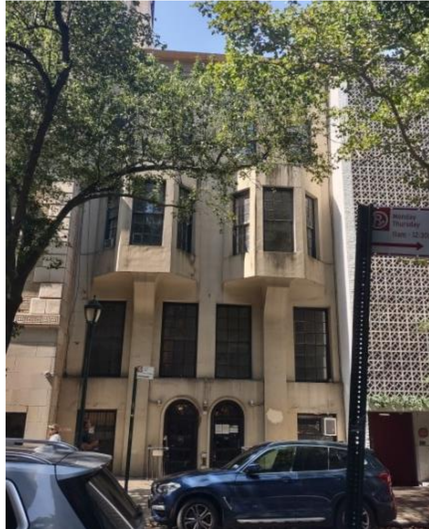
132 & 134 East 64 th Street, current condition.
