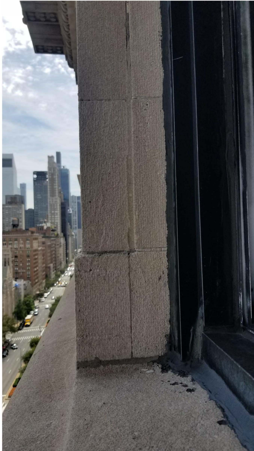
VIEW LOOKING SOUTH AT DEEP FENESTRATION OF EXISTING ALUMINUM REPLACEMENT WINDOWS
