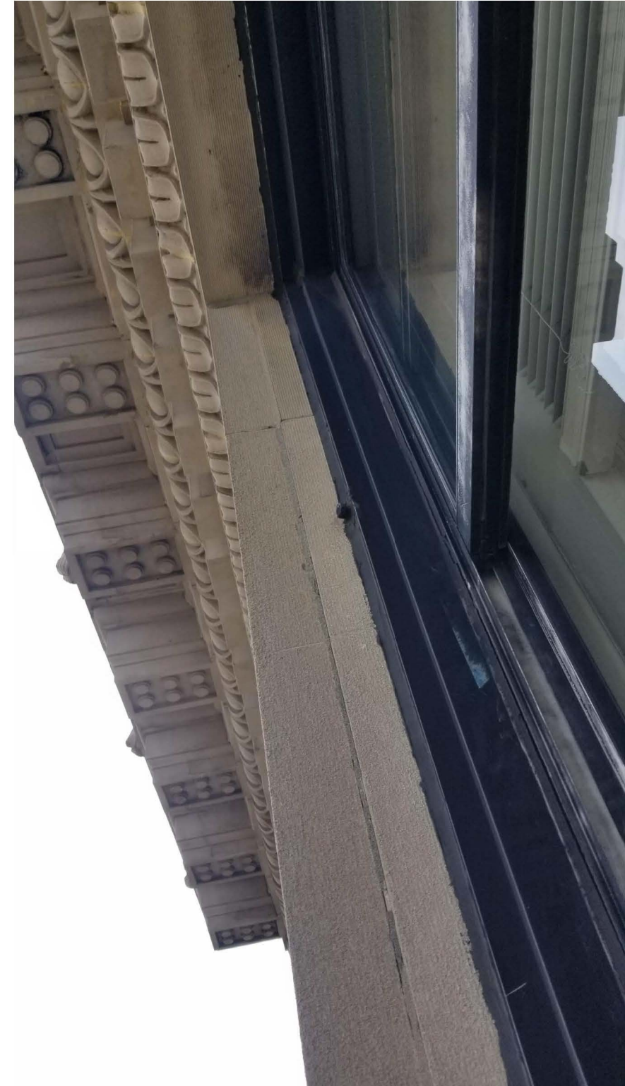
VIEW UP TOWARDS STRIKE & HEAD OF EXISTING ALUMINUM REPLACEMENT WINDOWS
