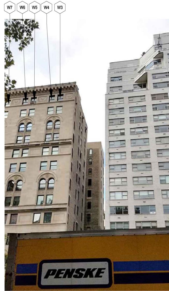
VIEW B : LOOKING AT NORTHEAST CORNER
