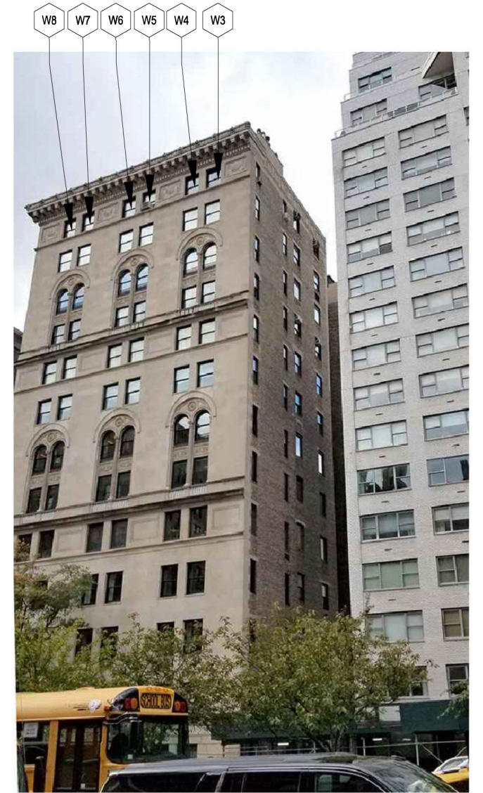
VIEW A : LOOKING AT NORTHEAST CORNER
