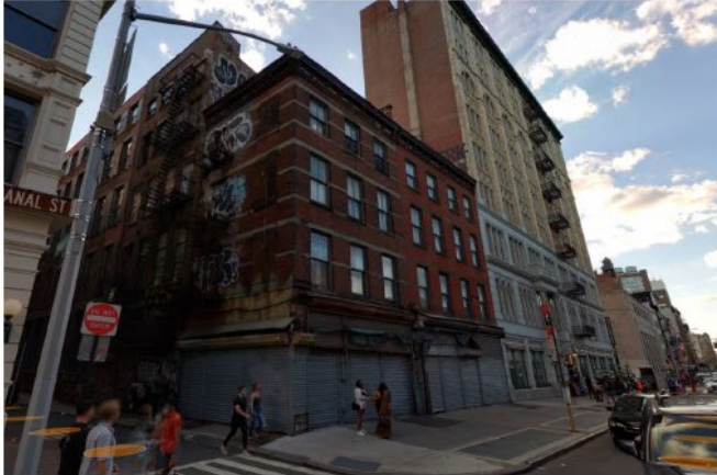
EXISTING PHOTO VIEW FROM CANAL STREET AND CORTLANDT ALLEY 1
