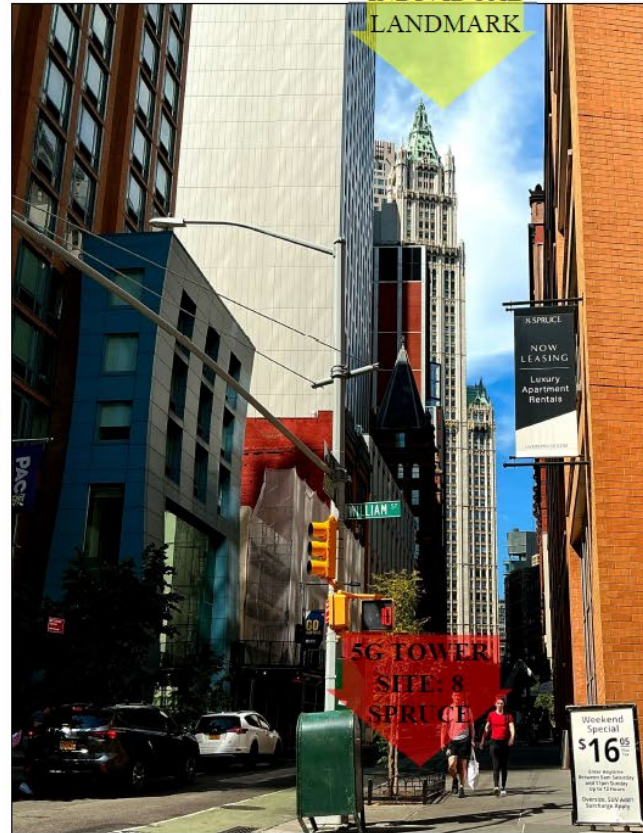
8 SPRUCE STREET LOOKING SOUTHWEST TOWARDS PROPOSED TOWER ON SEPTEMBER 21, 2024
