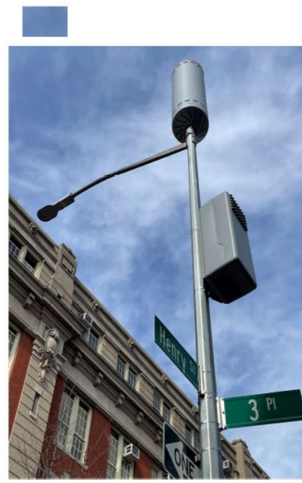
5G Poletop Installation (Existing Light Pole)
