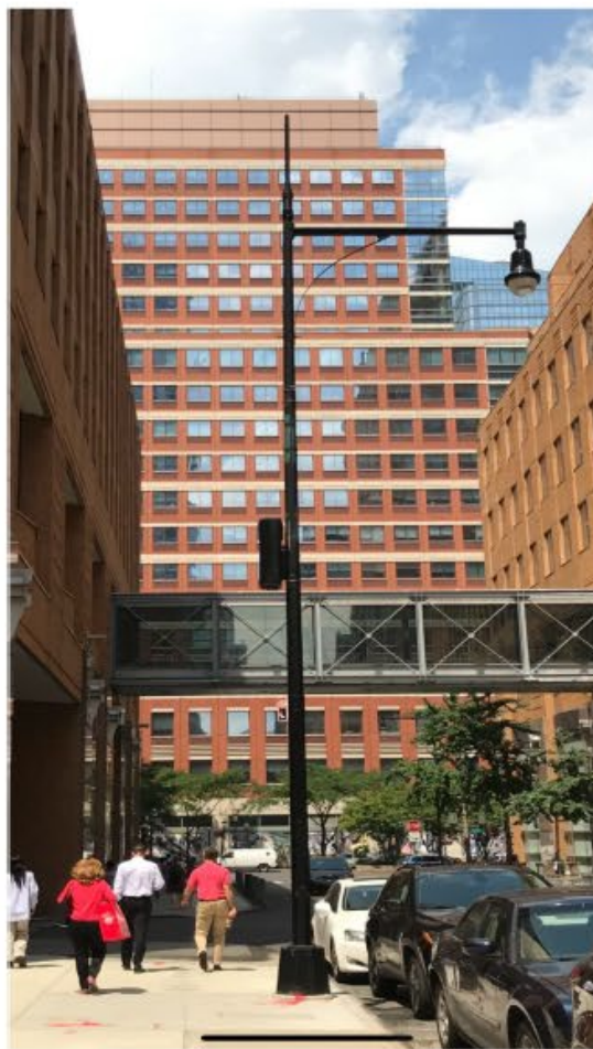
4G Poletop Installation (Existing Light Pole)
