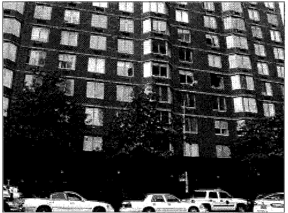
750 Columbus Avenue, view looking west 18
