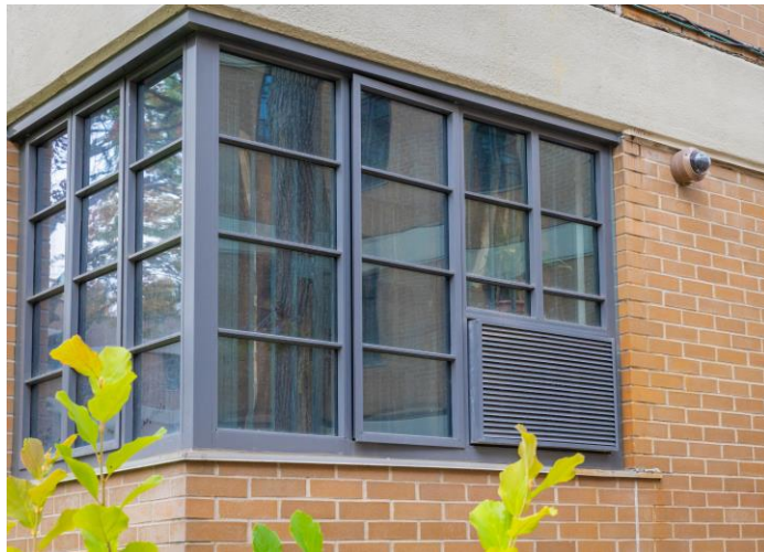
New windows, Williamsburg Houses
