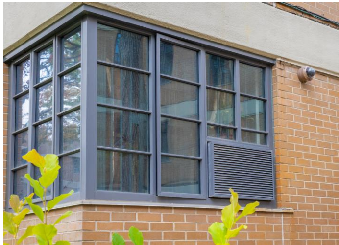
New windows, Williamsburg Houses
