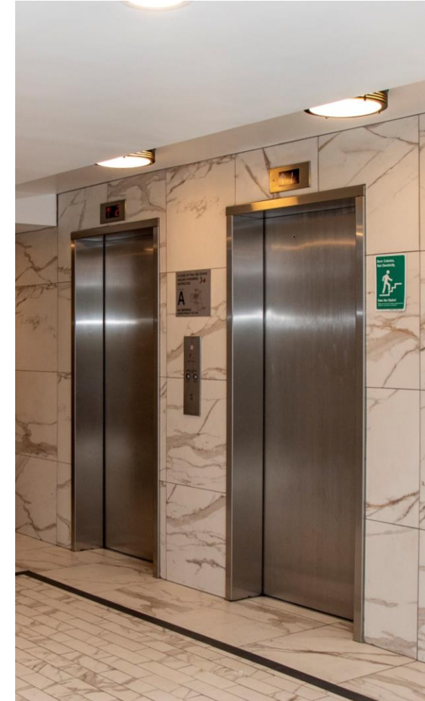
Upgraded elevators, Independence
