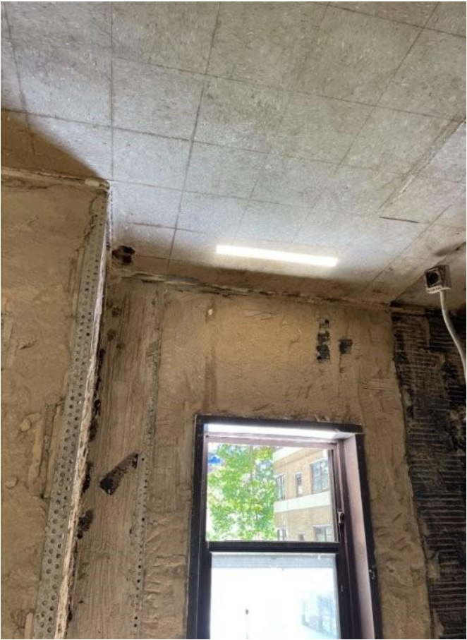
Abatement via full removal at Williamsburg Houses
