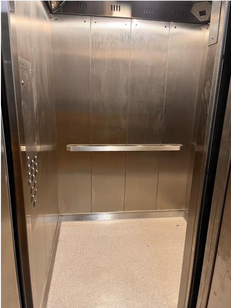
New elevators at Richmond Terrace
