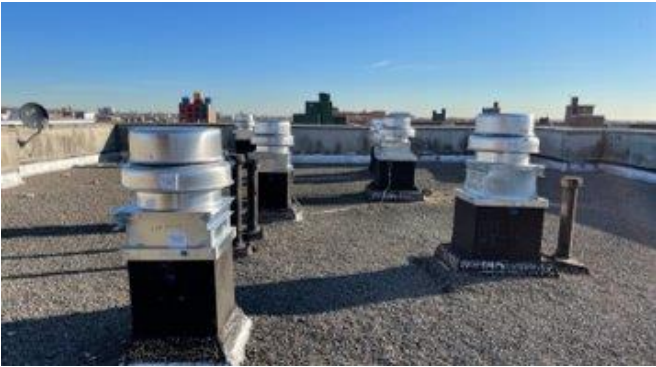
New roof fans
