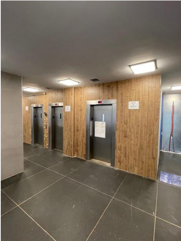
New elevators at 344 East 28 th Street
