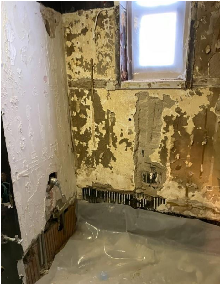
Abatement via full removal at Harlem River Houses
