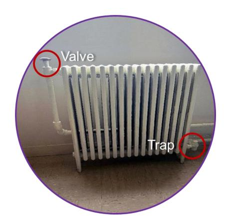
Replacement of the steam trap and valve to provide consistent and reliable heat to apartments
