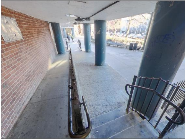
Existing Building #7 porch
