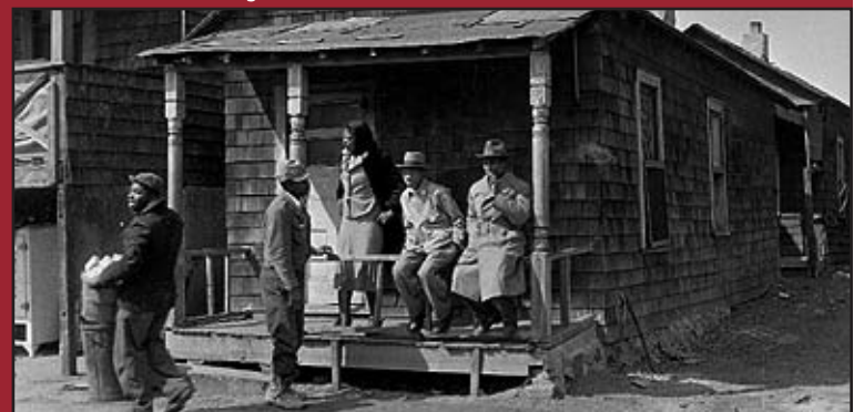
People resting on the porch of 1124 Dabney Avenue in Rockaway, Queens, March 1950. This was part of the 19 acres cleared to build Redfern Houses.
