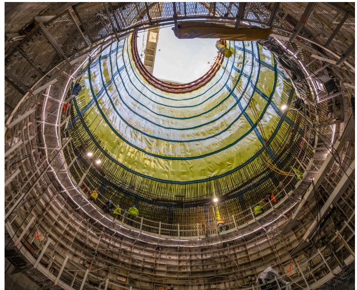
Tunnel No. 3 shaft construction
