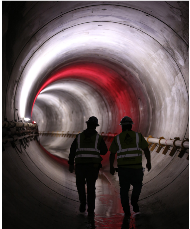
Rondout-West Branch bypass tunnel
