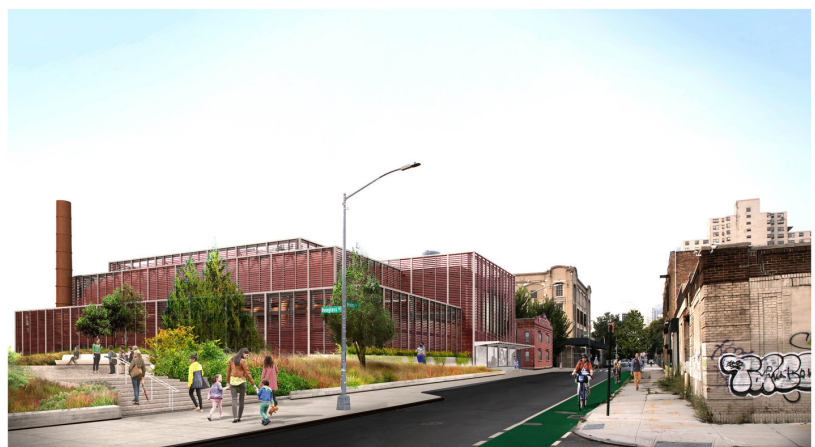
Gowanus Canal Combined Sewer Overflow Facility
