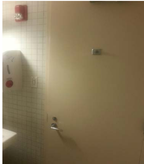
Service center bathroom door painted after CORE inspection
