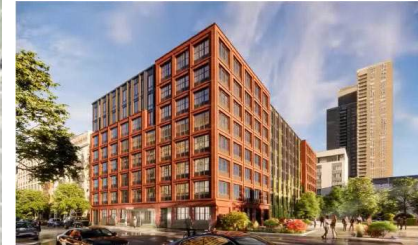
705 10th Avenue: DEP Site
