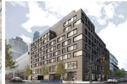
806 9th Avenue: MTA Site
