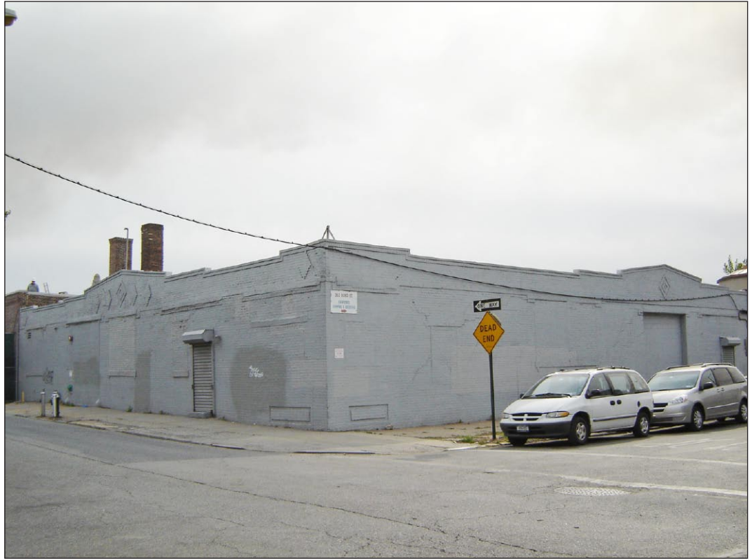
View from Bond Street at First Street looking northeast towards Building 2.
