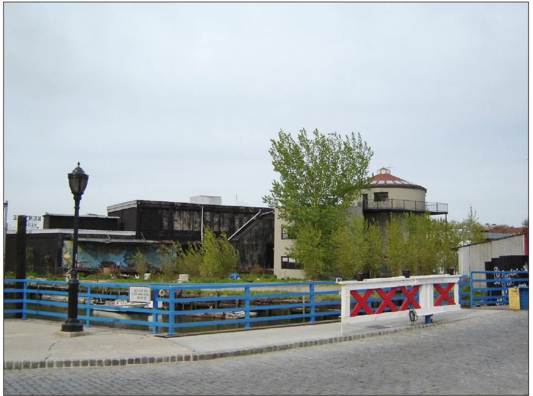
View from the east side of the Carroll Street Bridge looking west towards the project site.
