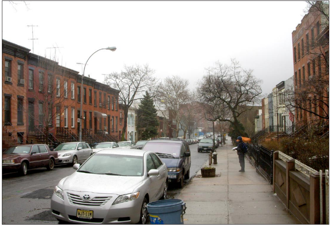
View from Second Street between Bond and Hoyt streets, looking east towards the project site and the Gowanus Canal. The project site and the Brooklyn Rapid Transit Power House can be seen in the center background.
