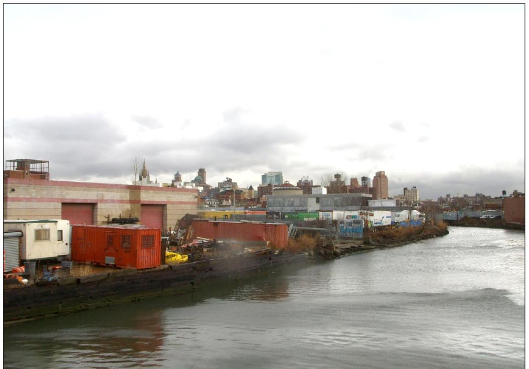
View from the Third Street Bridge over the Gowanus Canal, a view looking northwest towards the project site. St. Agnes' Church, identified as a visual resource, is visible in the background.
