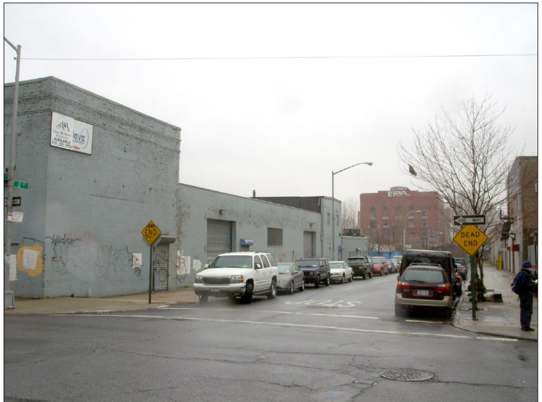
View looking northeast on Second Street towards the Gowanus Canal, a portion of Building 1 is pictured on the left. 2
