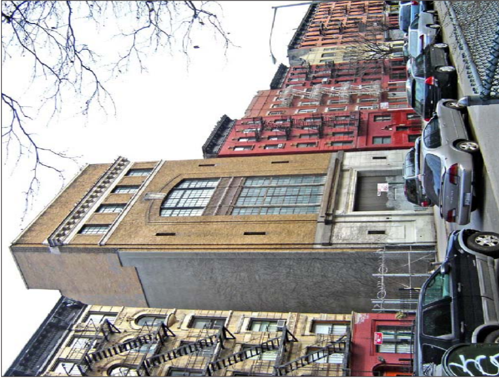
Substation at 421 East 6th Street (121) 122
