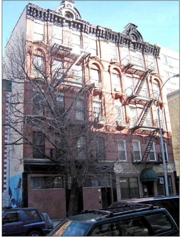
Tenements at 517-519 East 11th Street (126) 128
