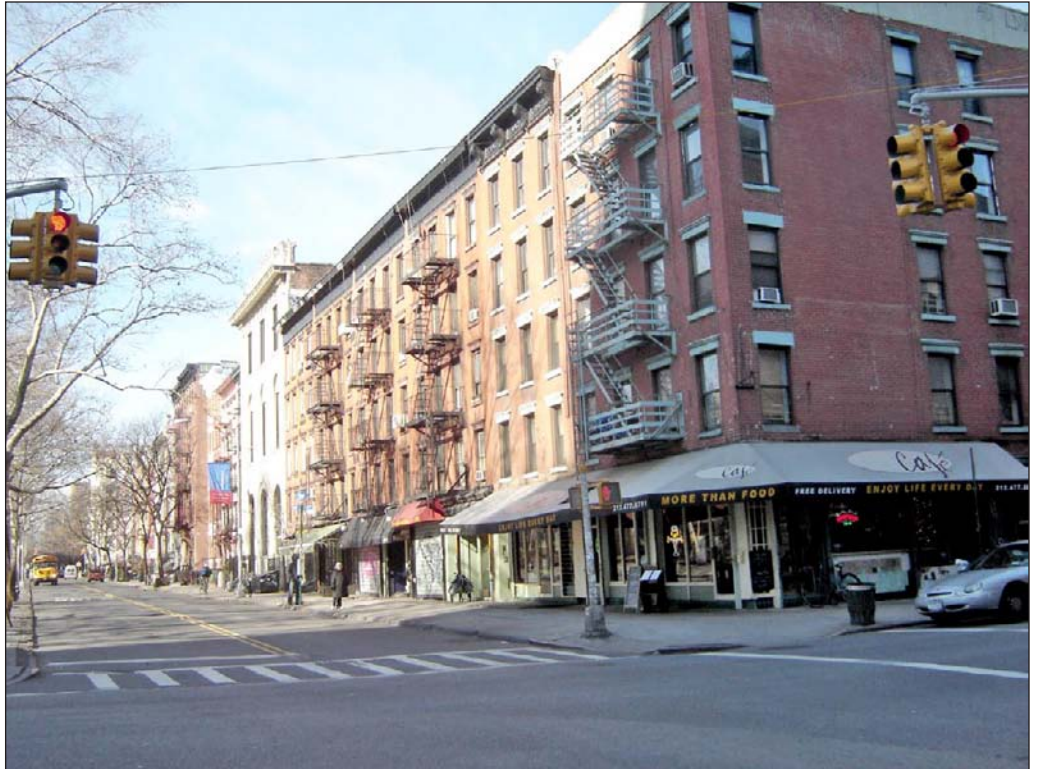
293-345 East 10th Street. View west from Avenue B 69
