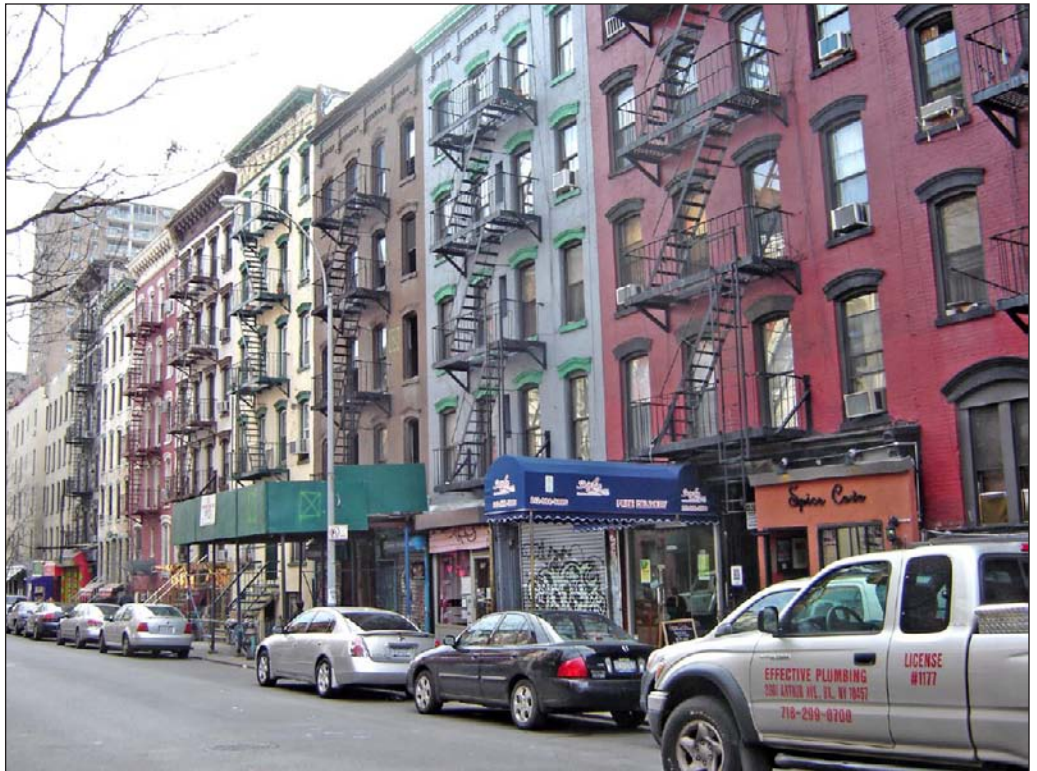
310-340 East 6th Street. View east from midblock 84
