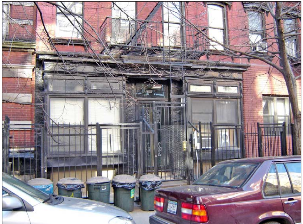
Tenement at 236 East 7th Street (149). 153 Detail of storefront
