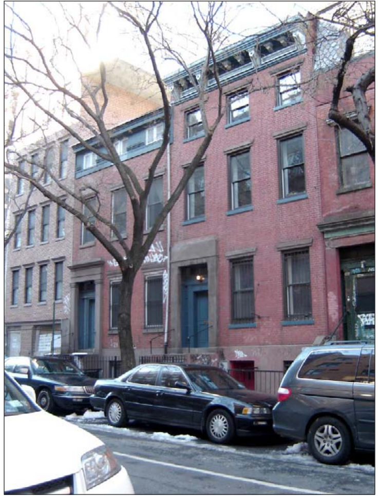
Greek Revival row house at 28 East 2nd Street (28) 25
