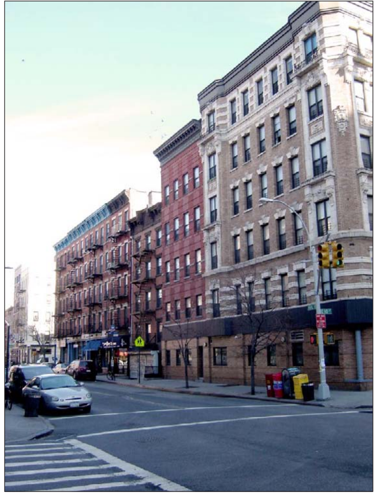
163-173 Avenue B. View north from East 10th Street 71
