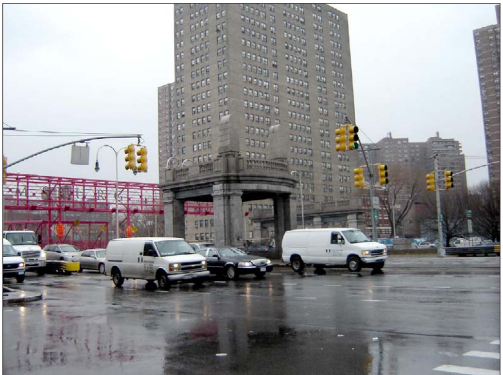
Williamsburg Bridge (86). 66 Entry plaza at Delancey and Clinton Streets
