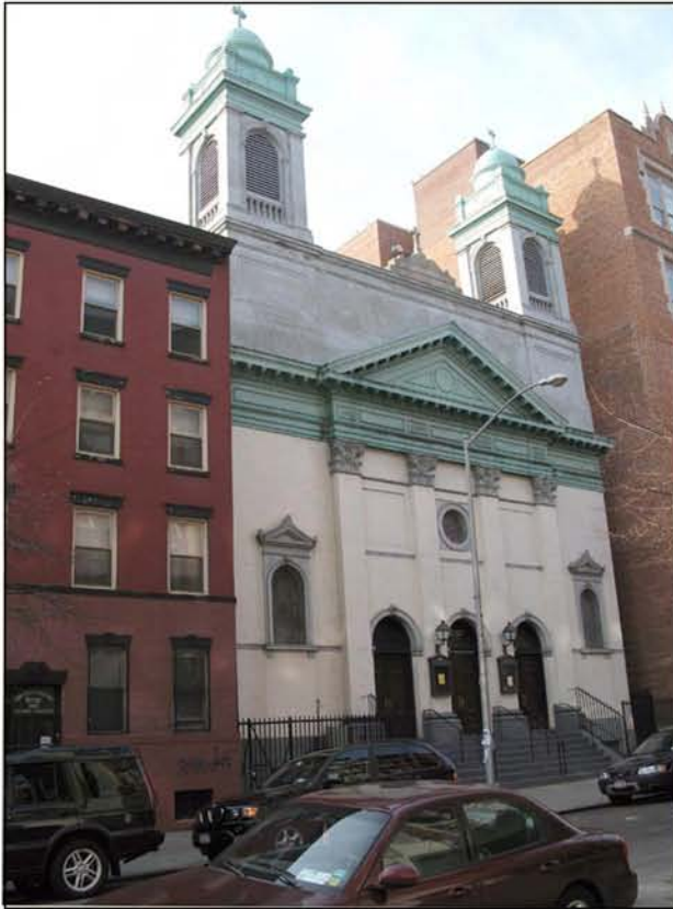
A. View of lots 26 (right) and 27 (left) on East 12th Street
