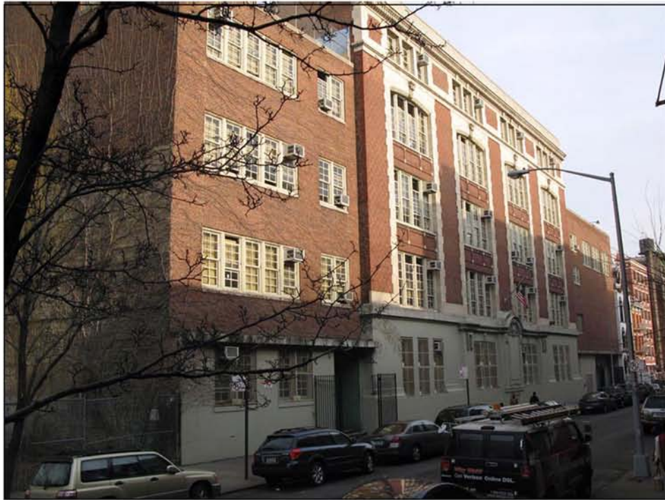
A. View of lot 20 on East 4th Street
