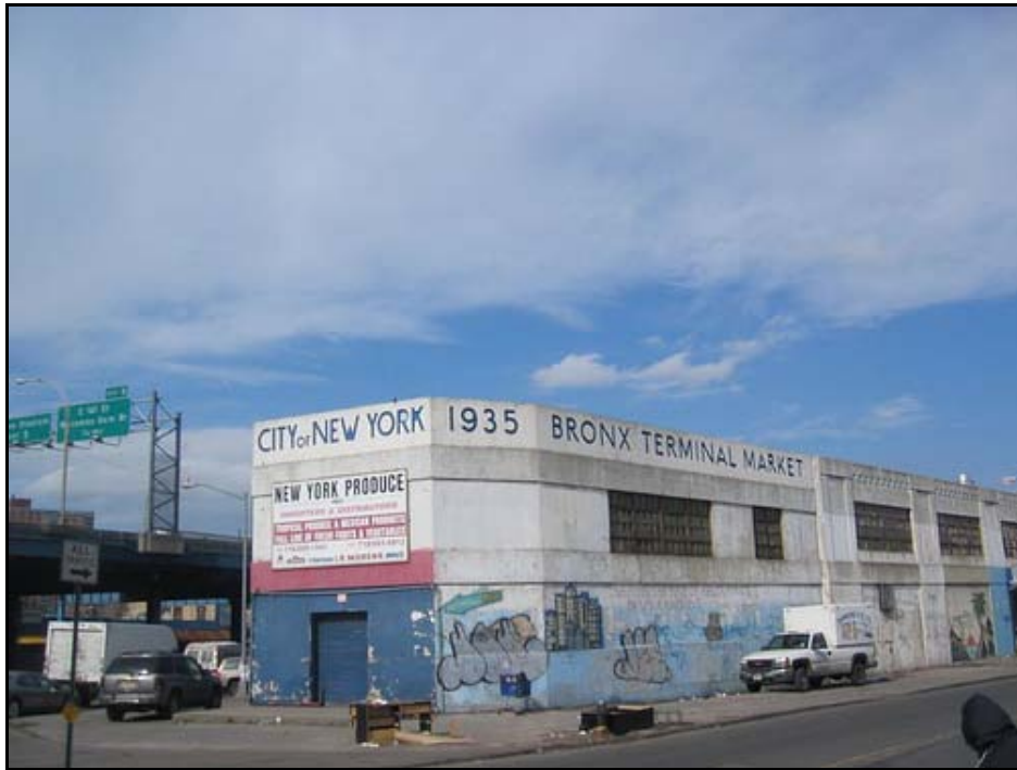
(5) View looking north-northwest to Building D (Resource #5), at the intersection of River Avenue and East 149 th Street, the sole surviving structure of the former Bronx Terminal Market.
