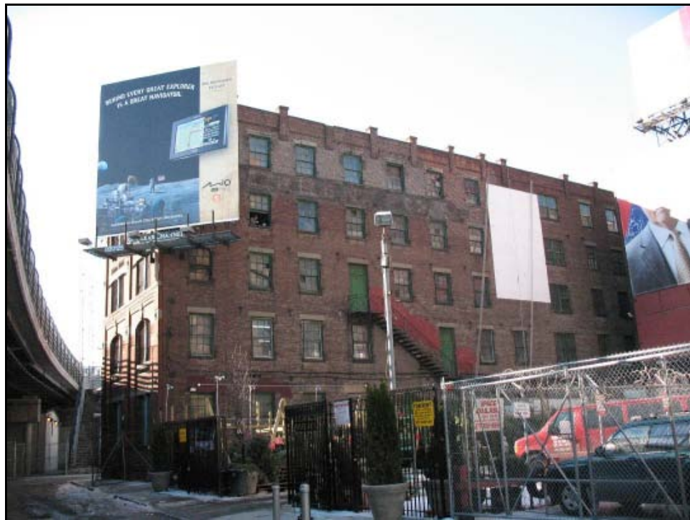
(8) View looking west-northwest toward the J. L. Mott Iron Works (Resource #8), at 220 East 134 th Street.
