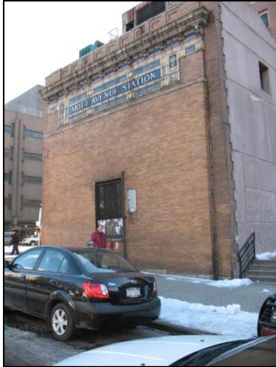
(3) View looking southeast to the Mott Avenue Control House (Resource #3) at the southwest corner of East 149 th Street and the Grand Concourse.
