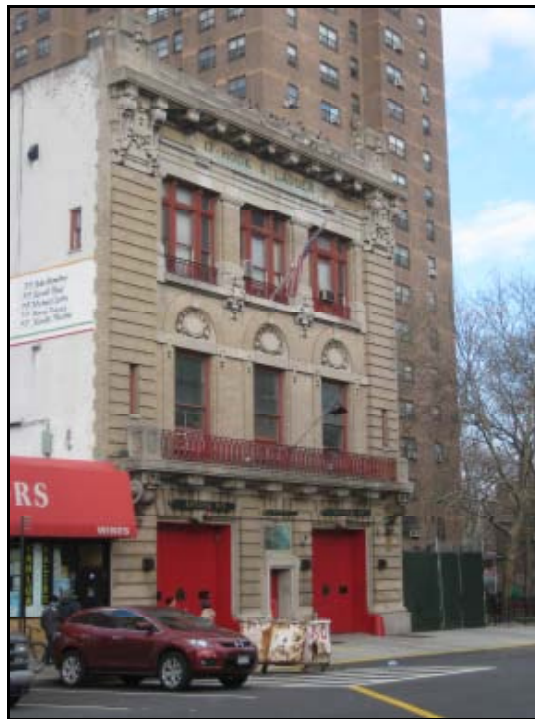
(12) View looking northeast toward the Firehook and Ladder Company 17 (Resource #12)
