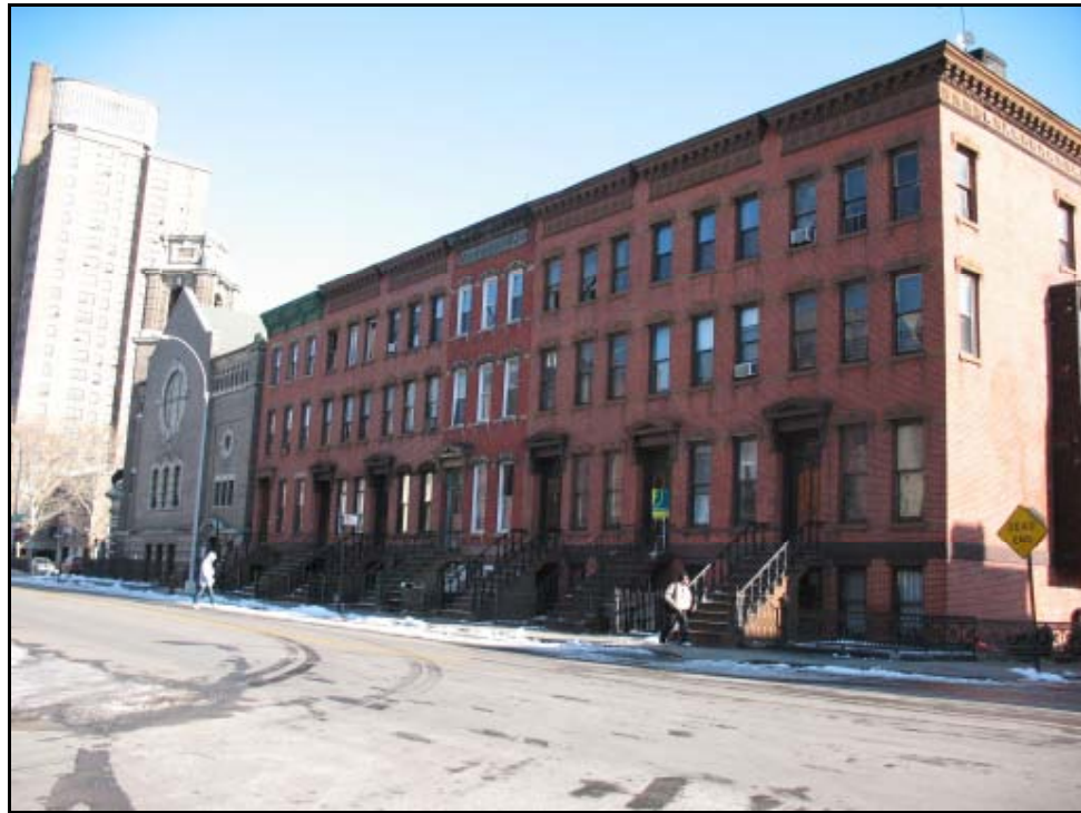
(9) View looking northeast along Alexander Avenue in the Mott Haven NYC Landmarks Preservation Commission Historic District (Resource #9).
